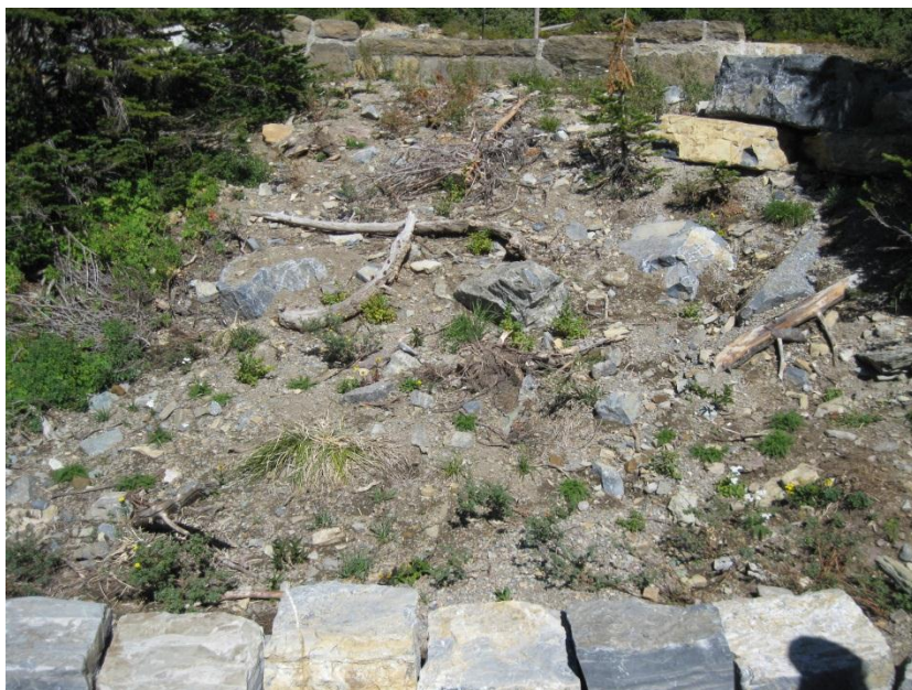
Area B. Open slope at end of walkway - 2012
