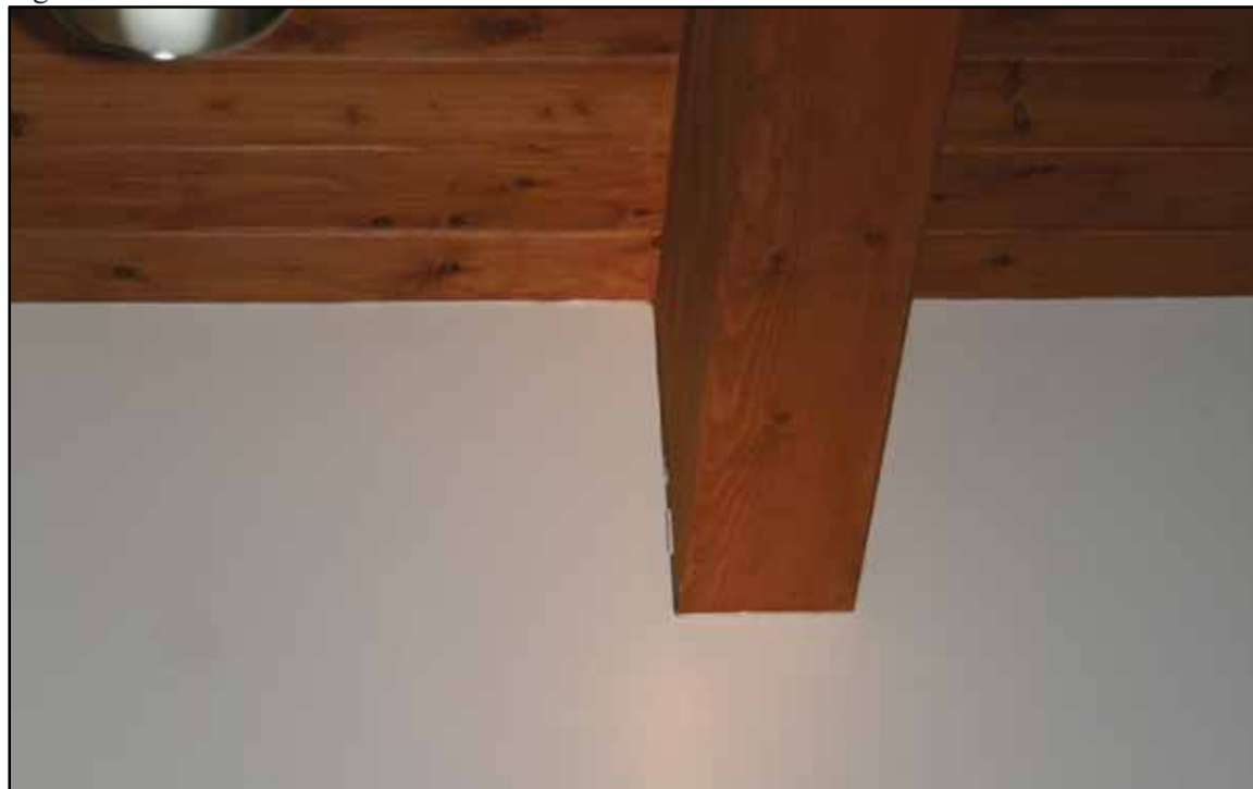
Figure 11. Northwest end of southwest wall of theater addition.
