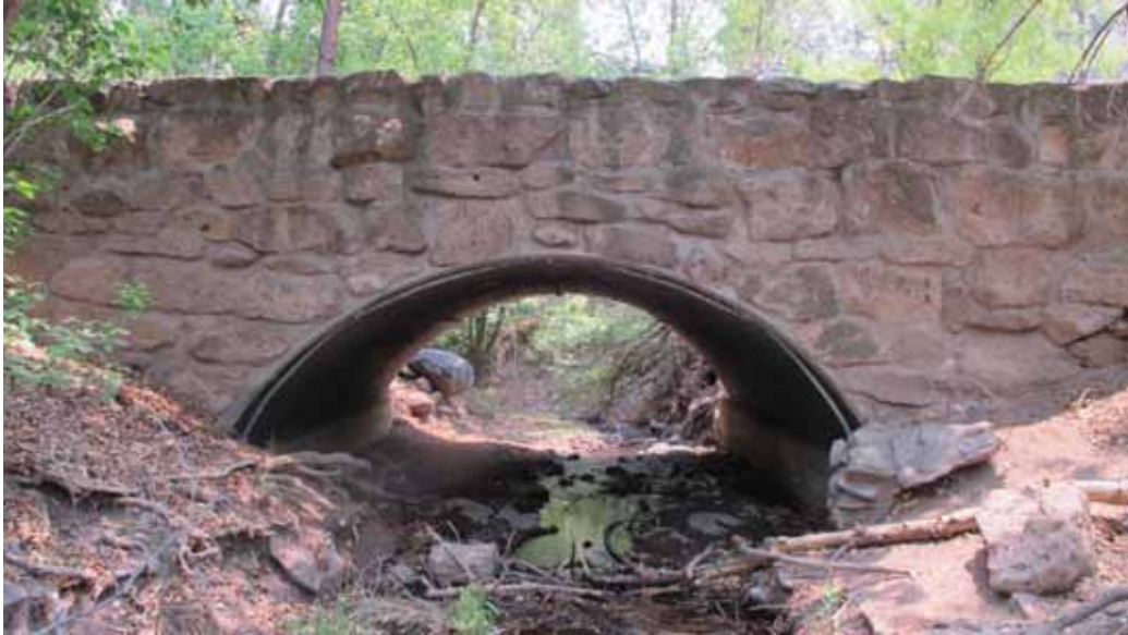
View 1 – Motor Car bridge as viewed from Rito de Frijoles; note that the bridge is essentially a large culvert.
