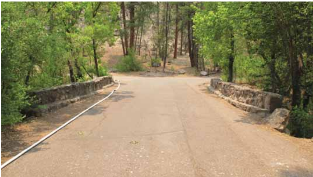
View 2 – Motor car bridge as viewed from the roadbed, crossing Rito de Frijoles.
