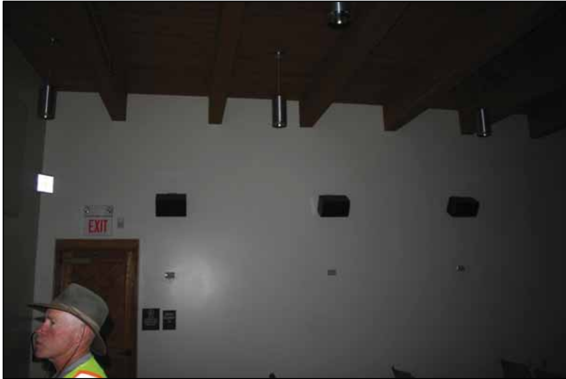
Figure 9. Southeast corner of addition.
