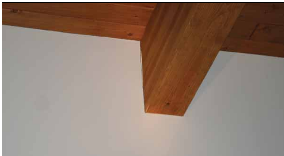
Figure 13. Closeup of wall and the 2 nd beam from the southeast end of the southwest wall of the theater addition.
