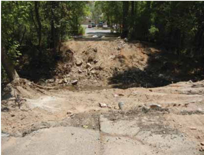
Site of removed motor car bridge.
