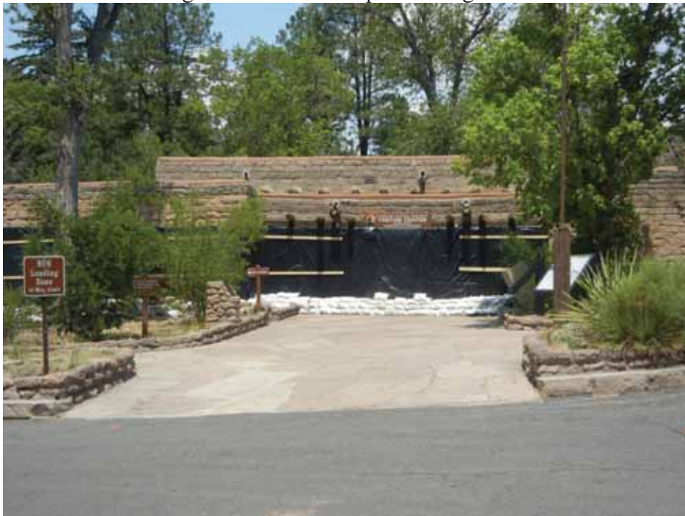
Plywood, plastic sheeting, and sandbags protecting Visitor Center.
