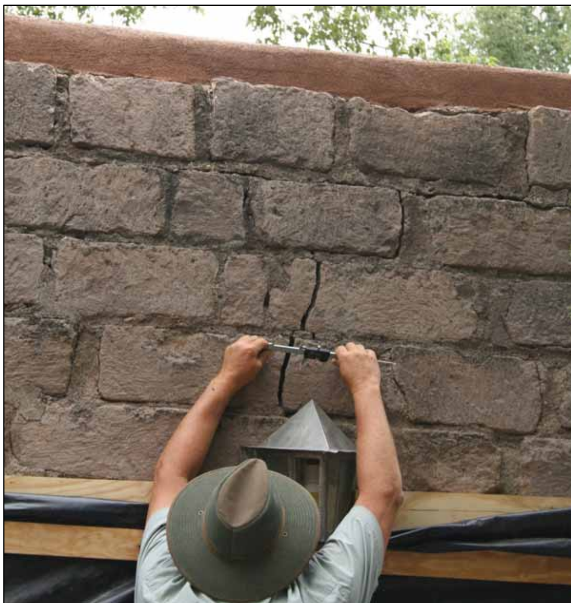
Figure 5. Caliper measurement point on Northwest end of Portale.
