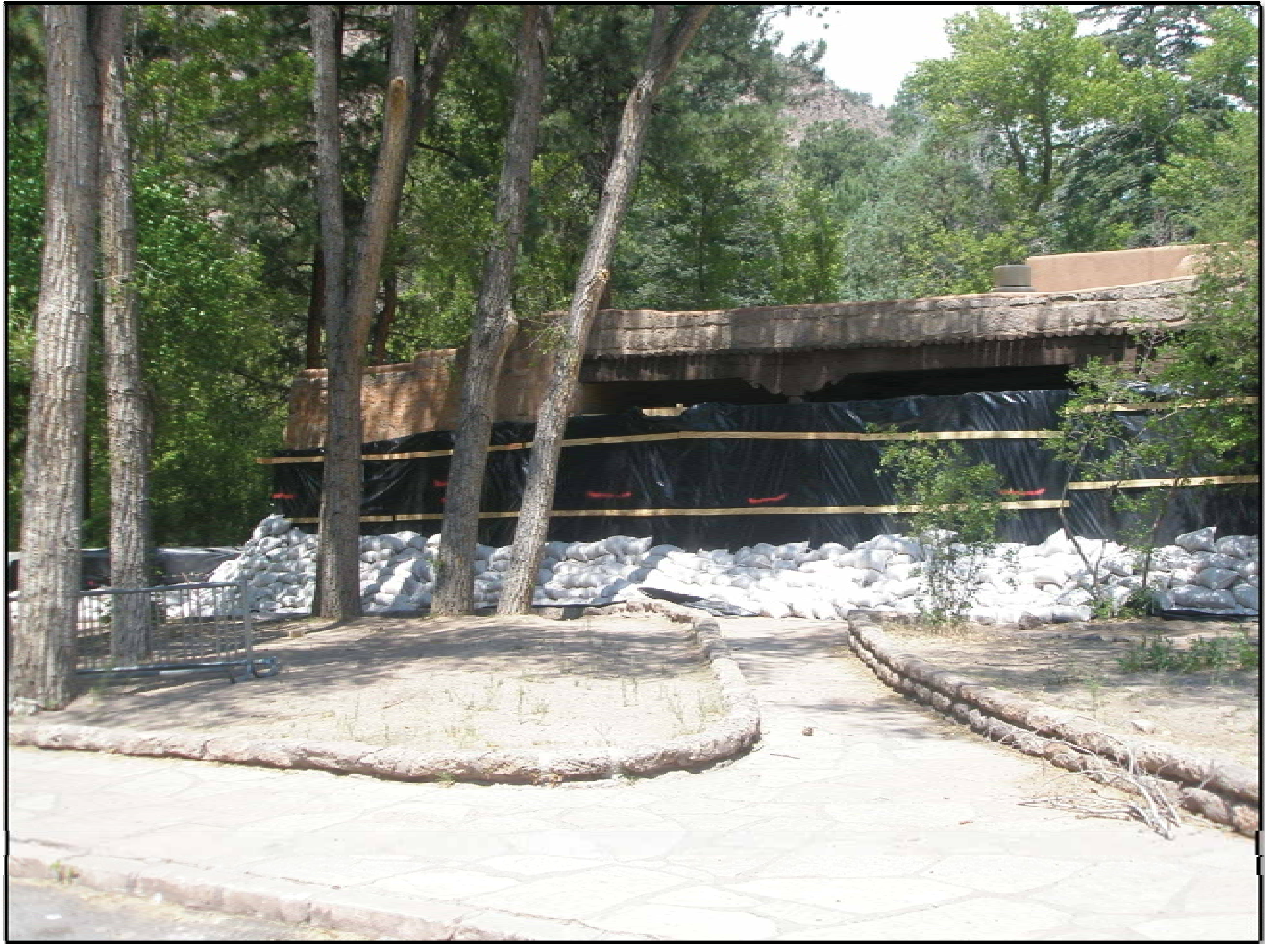
Figure 1. Structure Protection of the Visitors Center Addition
