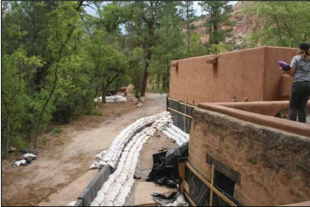
Figure 1. Looking Northwest showing sandbagging and armoring.
