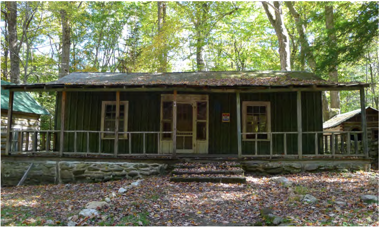
Figure 9: Higdon Cabin, east elevation.
