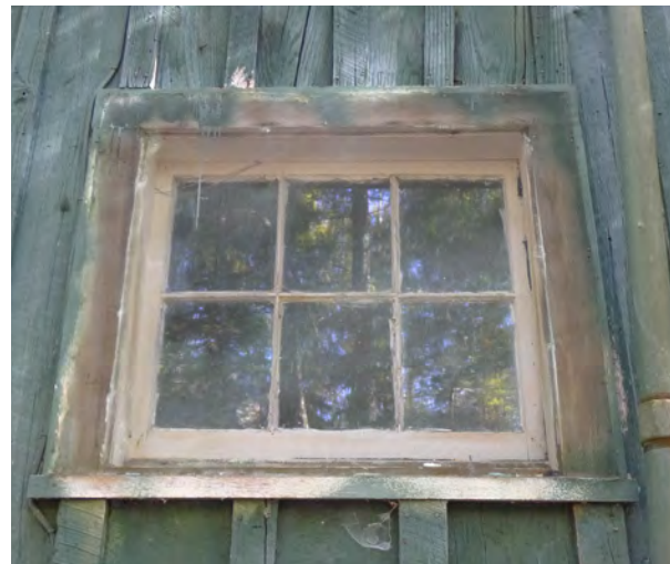
Figure 48: Evidence of a spray-painting campaign on the side of the Chapman-Byers cabin.
