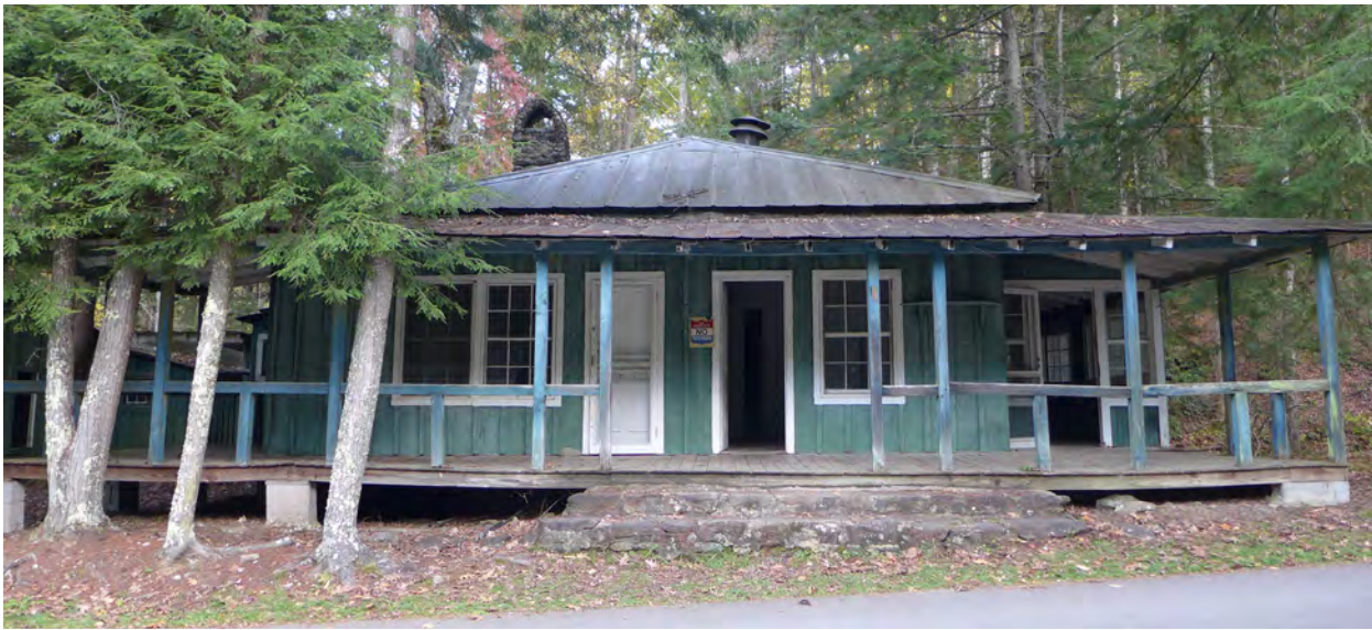
Figure 43: Hale Cabin, west elevation.
