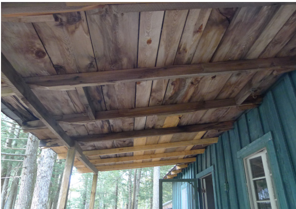
Figure 41: Unpainted porch ceiling with new repair wood.
