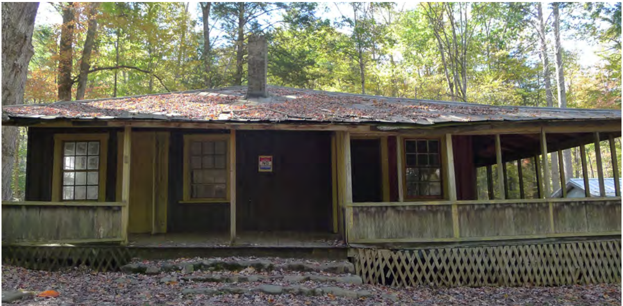
Figure 6: Smith Cabin, east elevation.
