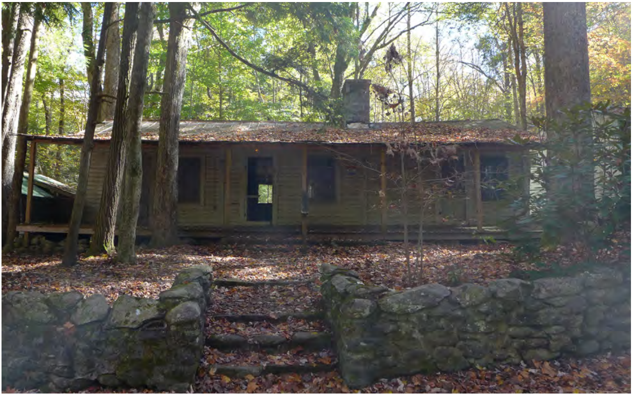
Figure 13: Addicks Cabin, west elevation.
