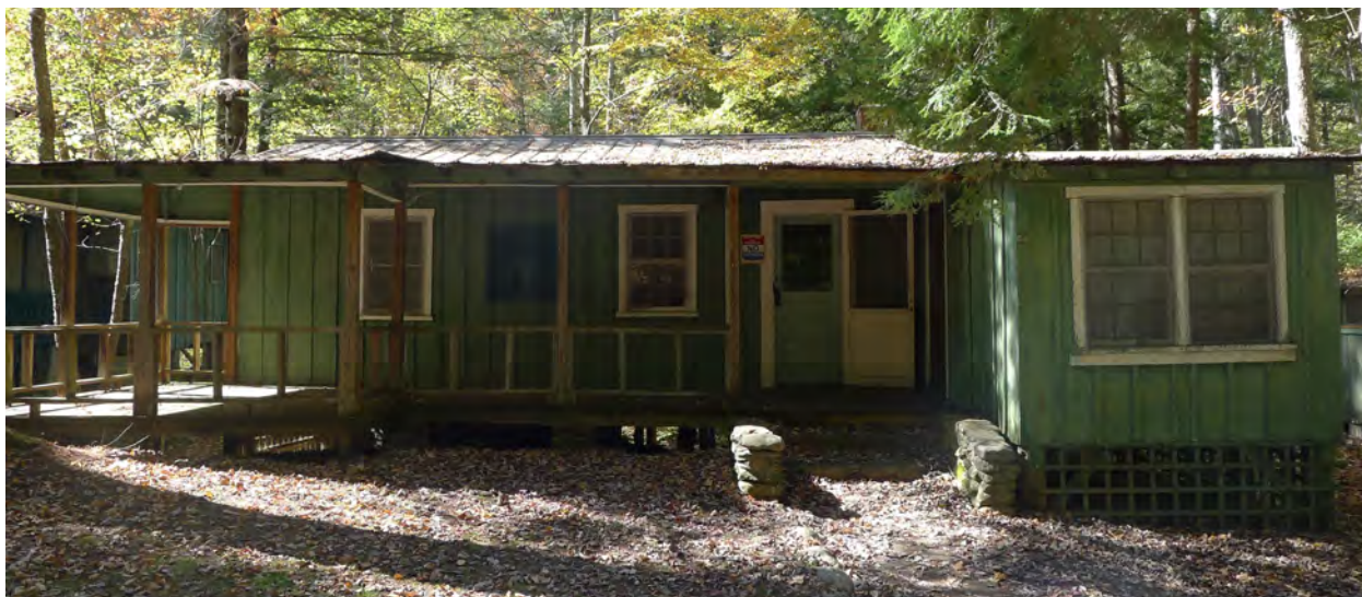
Figure 26: Cain Cabin, east elevation.
