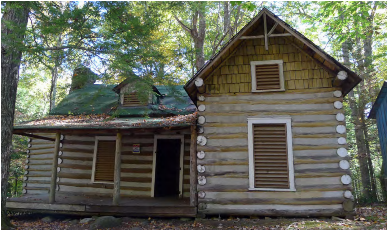
Figure 4: Sneed Cabin, east elevation.
