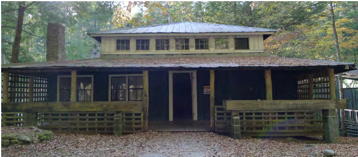
Figure 33: Baumann Cabin, east elevation.
