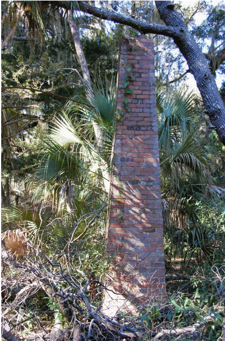
Figure 86: Brick Pyramid Structure.
