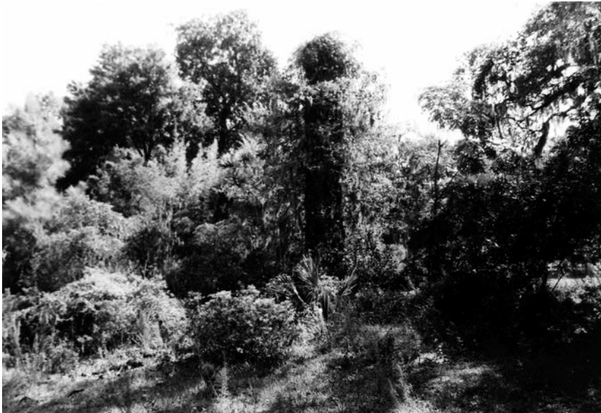
Figure 36: Housekeeper's Cottage foundation, 1994.
