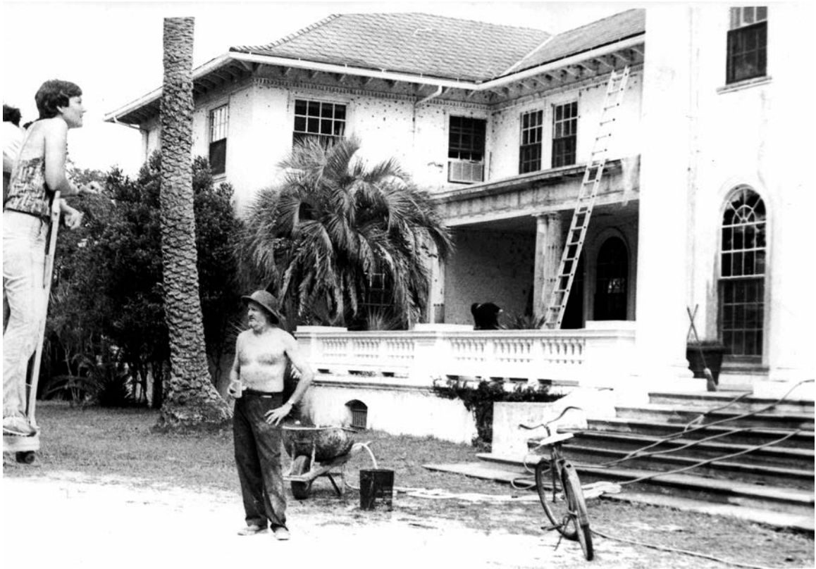
Figure 30: Roofing crew, c. 1977.
