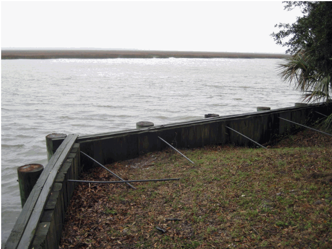
Figure 72: Seawall/Bulkhead.
