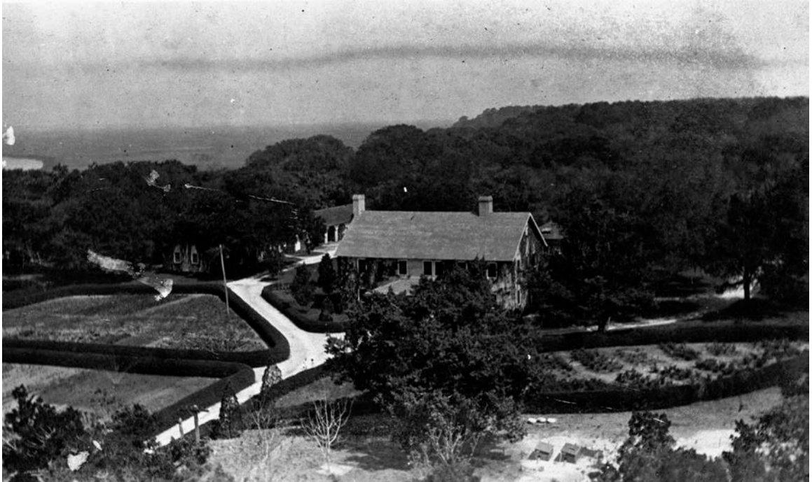
Figure 22: Formal garden spaces around the service road, c. 1910s.
