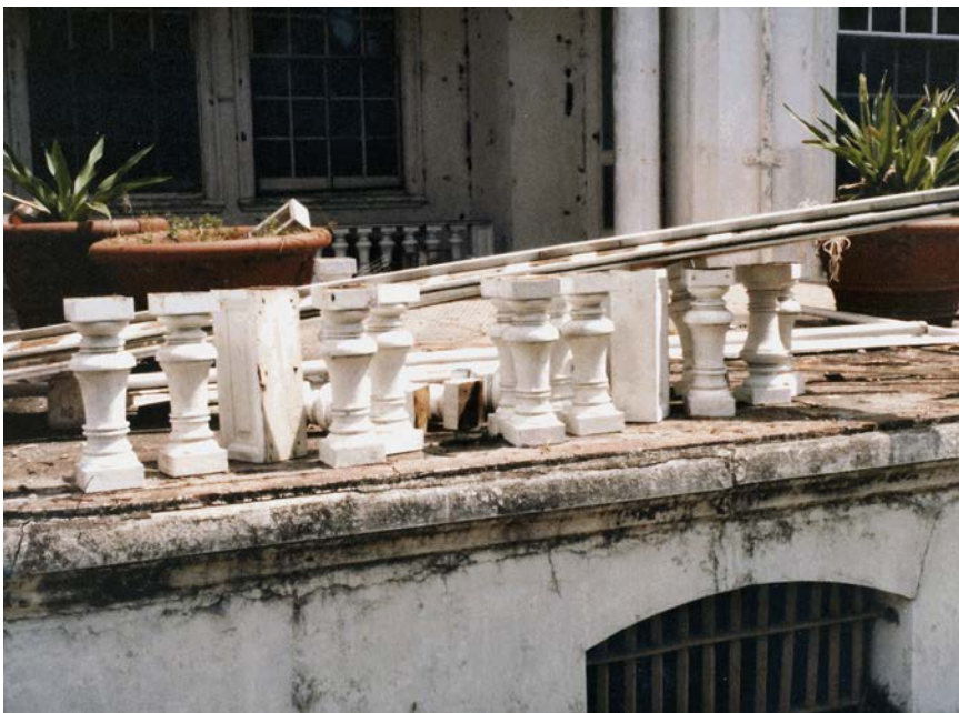
Figure 29: Porch repair, c. 1977.
