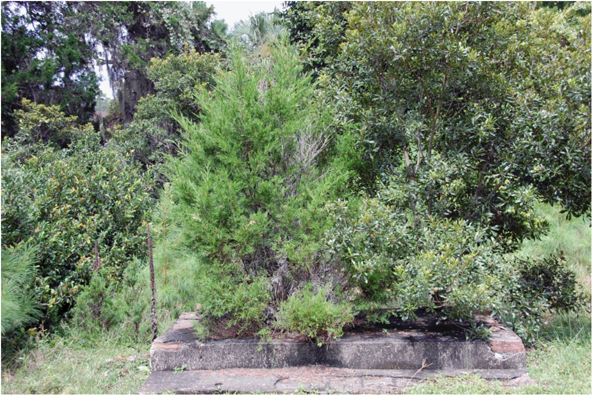
Figure 61: Laundry Building Foundation.
