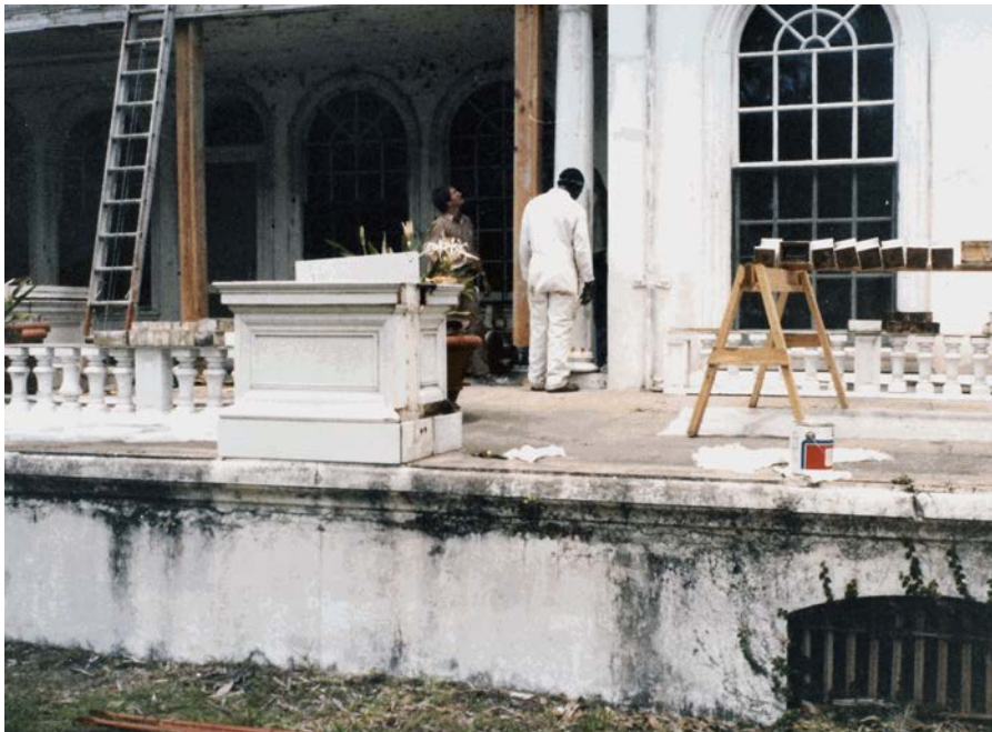
Figure 26: Porch repair, 1970s.
