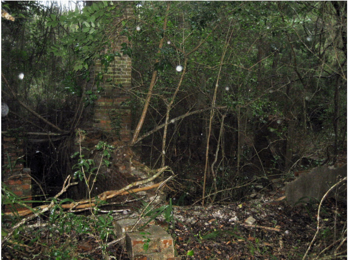
Figure 62: Housekeeper's Cottage Foundation.
