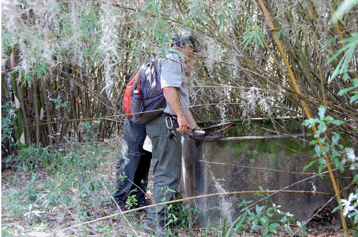
Figure 83: Duck Pond Concrete Enclosure.
