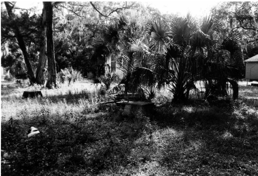
Figure 37: Water Tower foundation, 1994.
