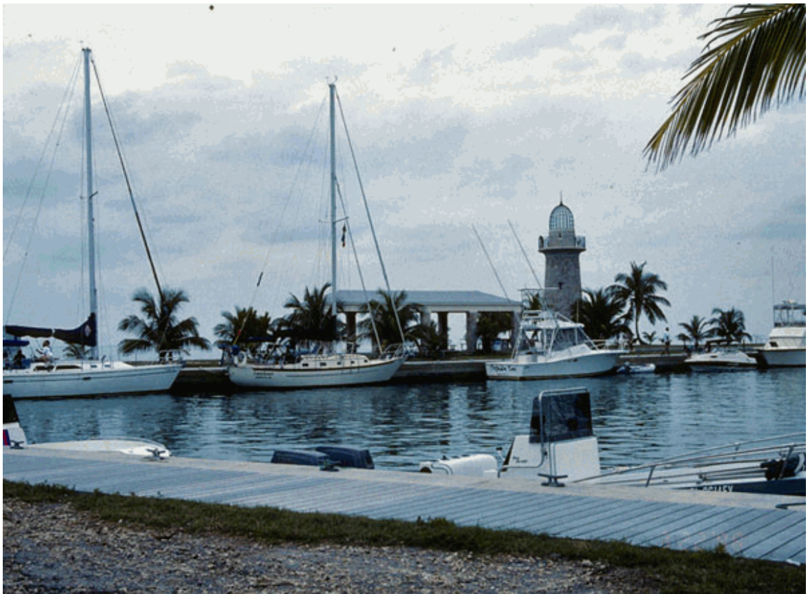
Graphic 31: Rebuilt bulkhead and boardwalk (National Park Service, Biscayne National Park).
