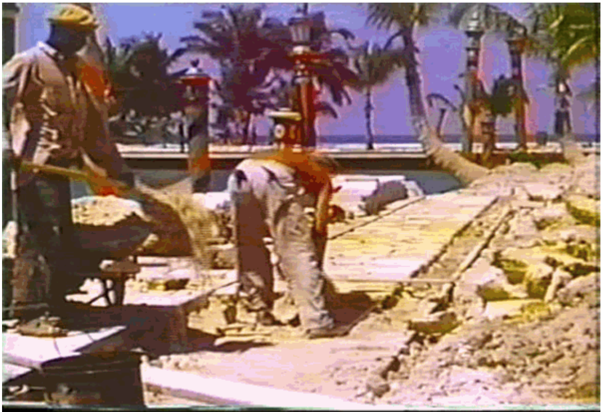
Graphic 13: Walkway under construction and harbor poles, still photo from 1930s construction video (Biscayne National Park Library).
