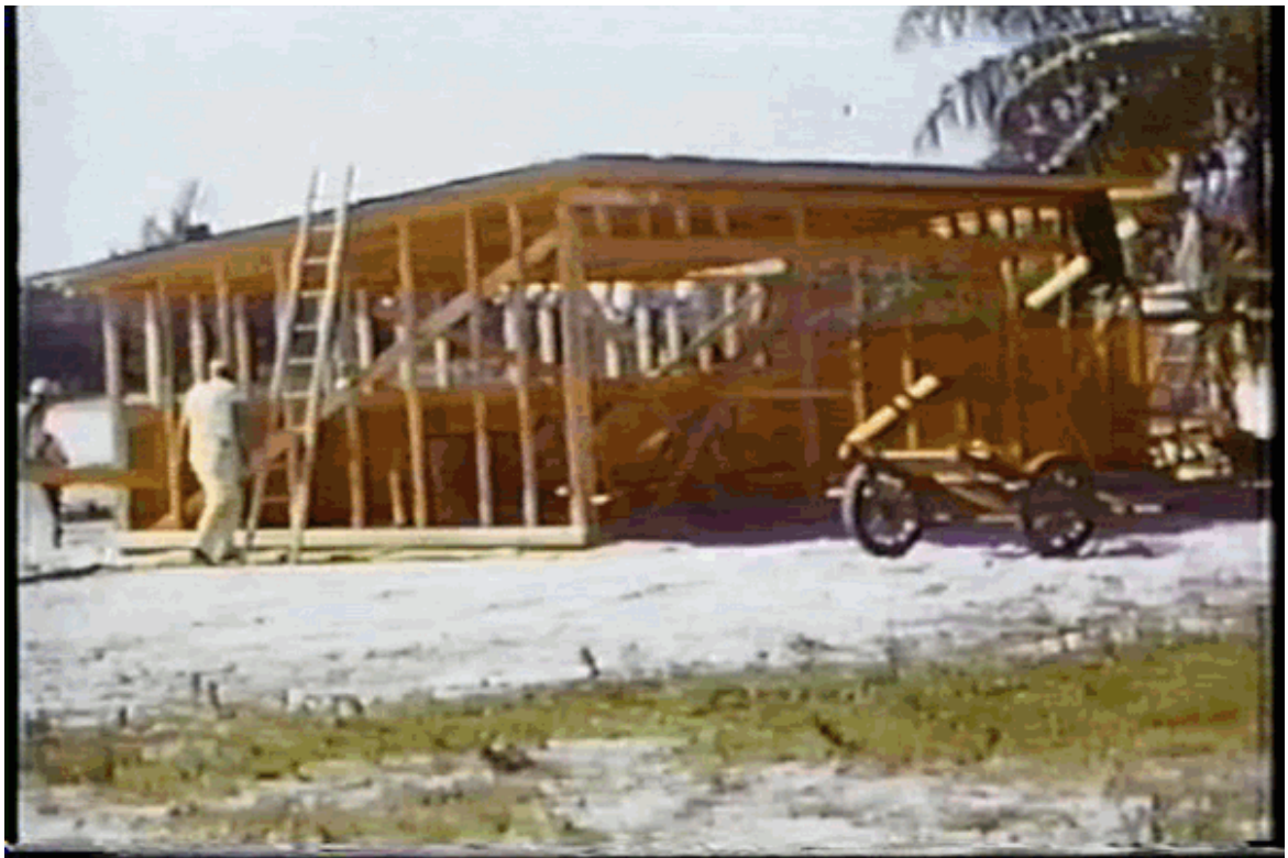
Graphic 11: Frame building under construction, still photo from 1930s construction video (Biscayne National Park Library).
