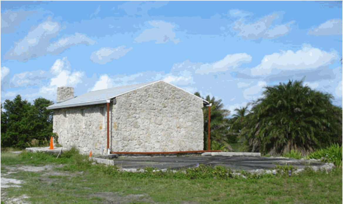
Graphic 45: Boca Chita Engine House and Cistern
