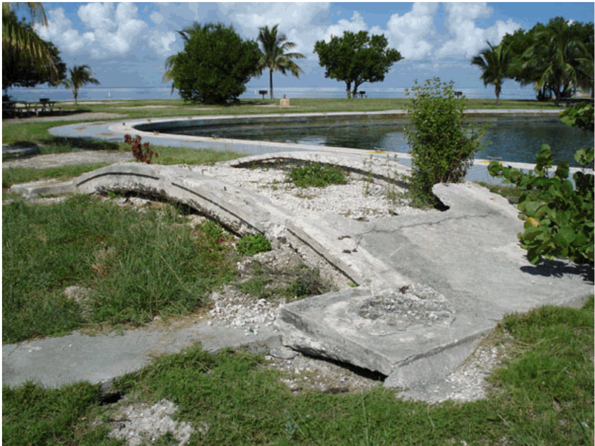
Graphic 46: Boca Chita arched concrete footbridge
