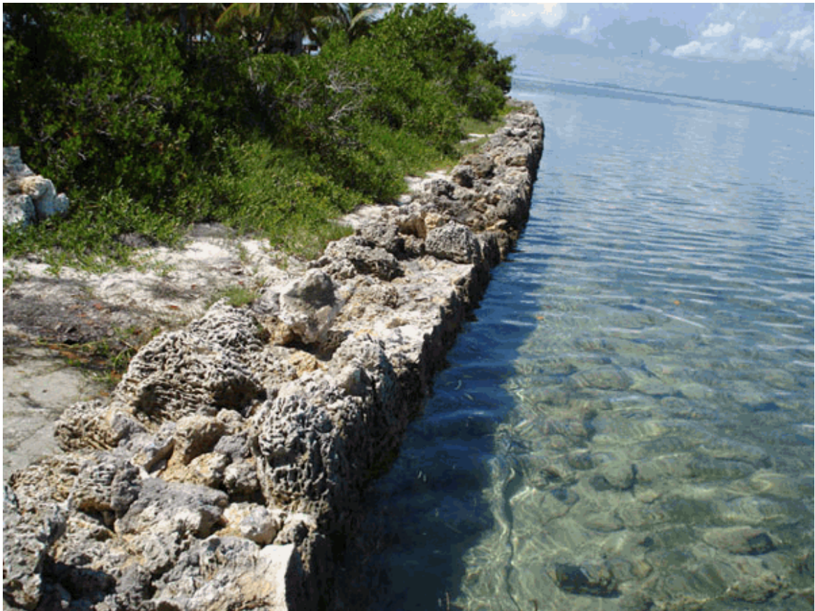
Graphic 49: Boca Chita retaining walls
