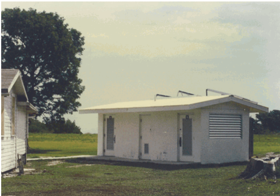
Graphic 27: Restroom building (National Park Service, Biscayne National Park).
