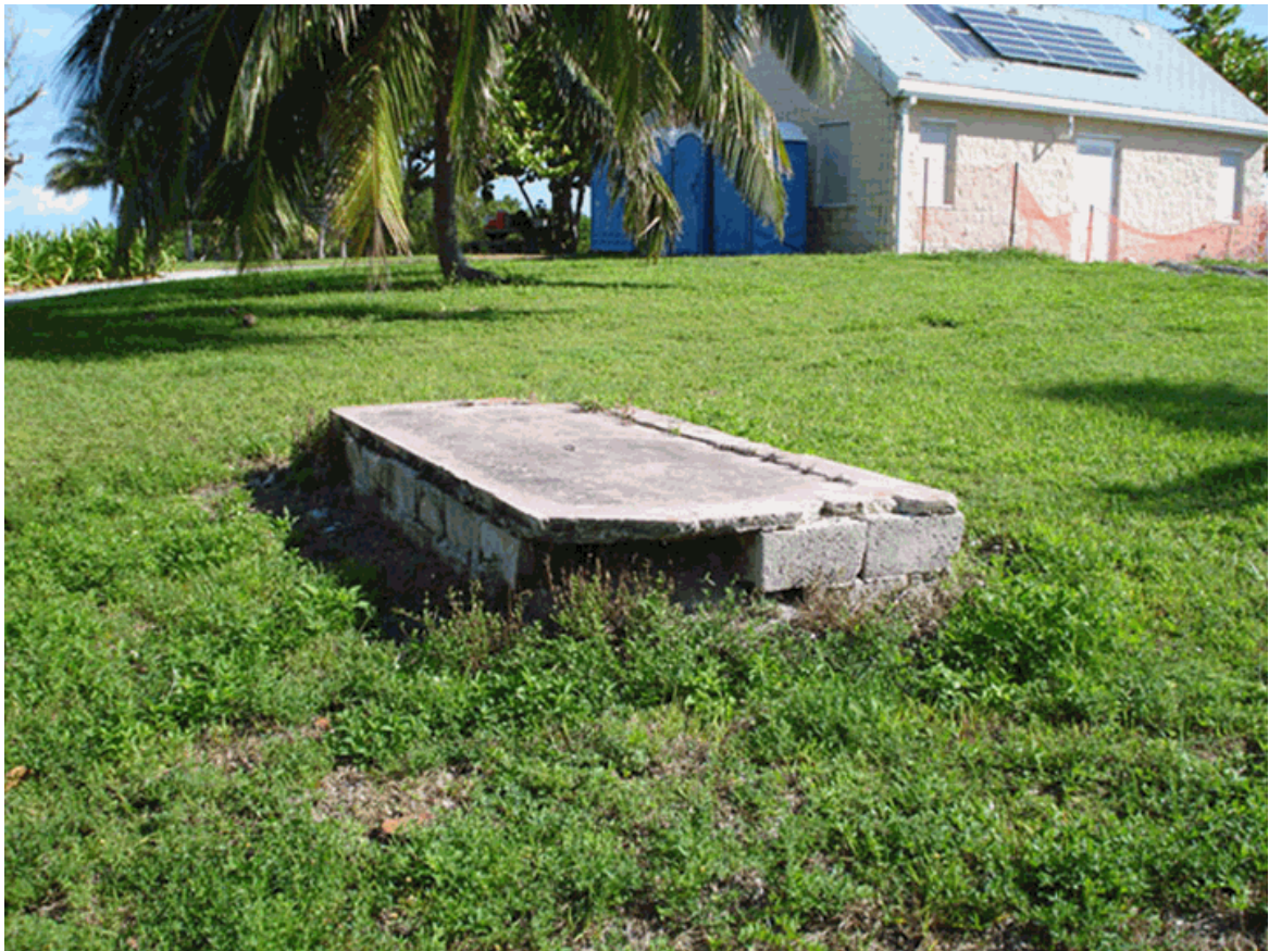
Graphic 51: Shower House foundation
