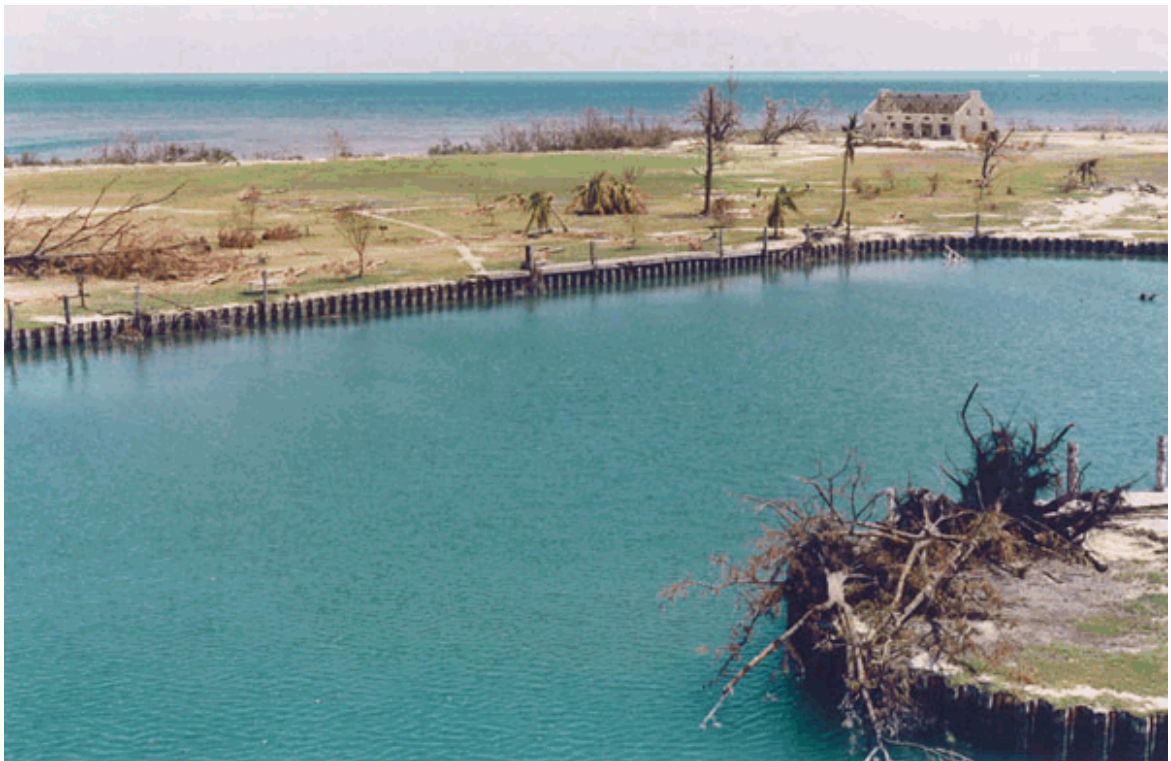
Graphic 30: Boca Chita after Hurricane Andrew (National Park Service, Biscayne National Park).
