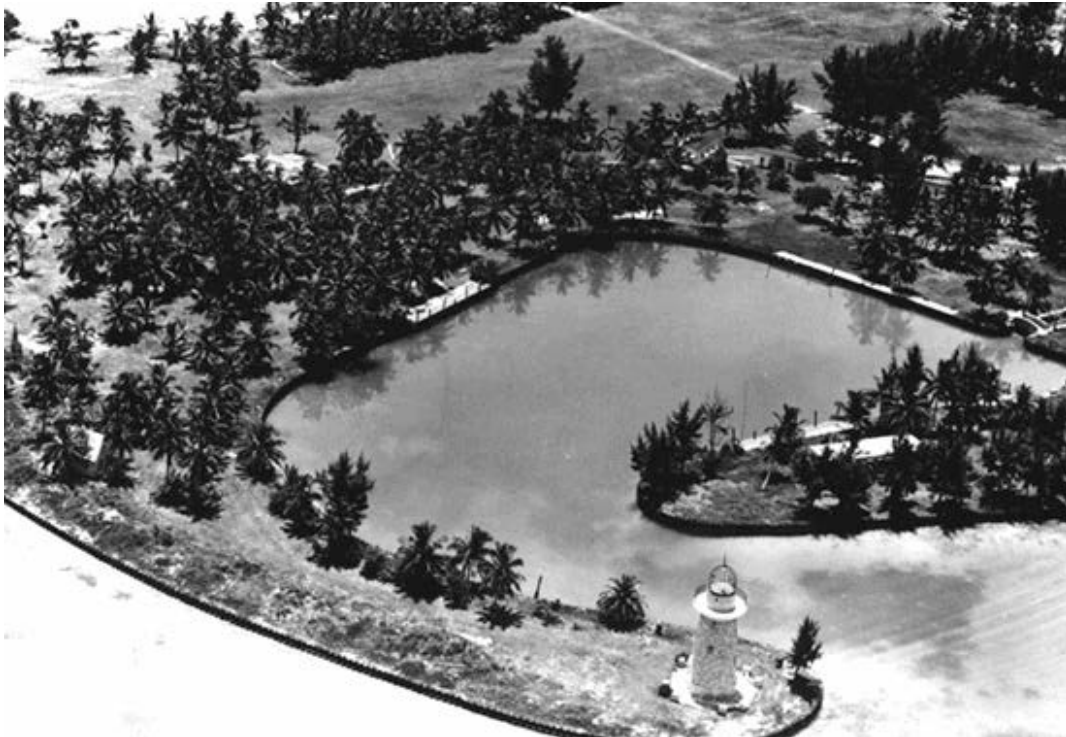
Graphic 19: Aerial photograph showing historic circulation on the island (South Florida Collection Management Center).
