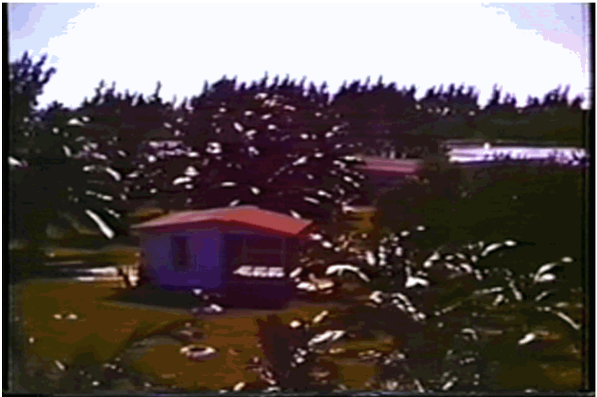
Graphic 10: Frame Structures, still photo from 1930s construction video (Biscayne National Park Library).
