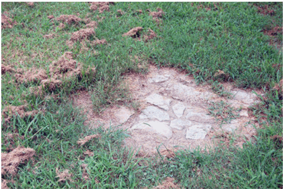
Figure 38: Well foundation, 2011. (Susan Hitchcock/NPS image 0686)
