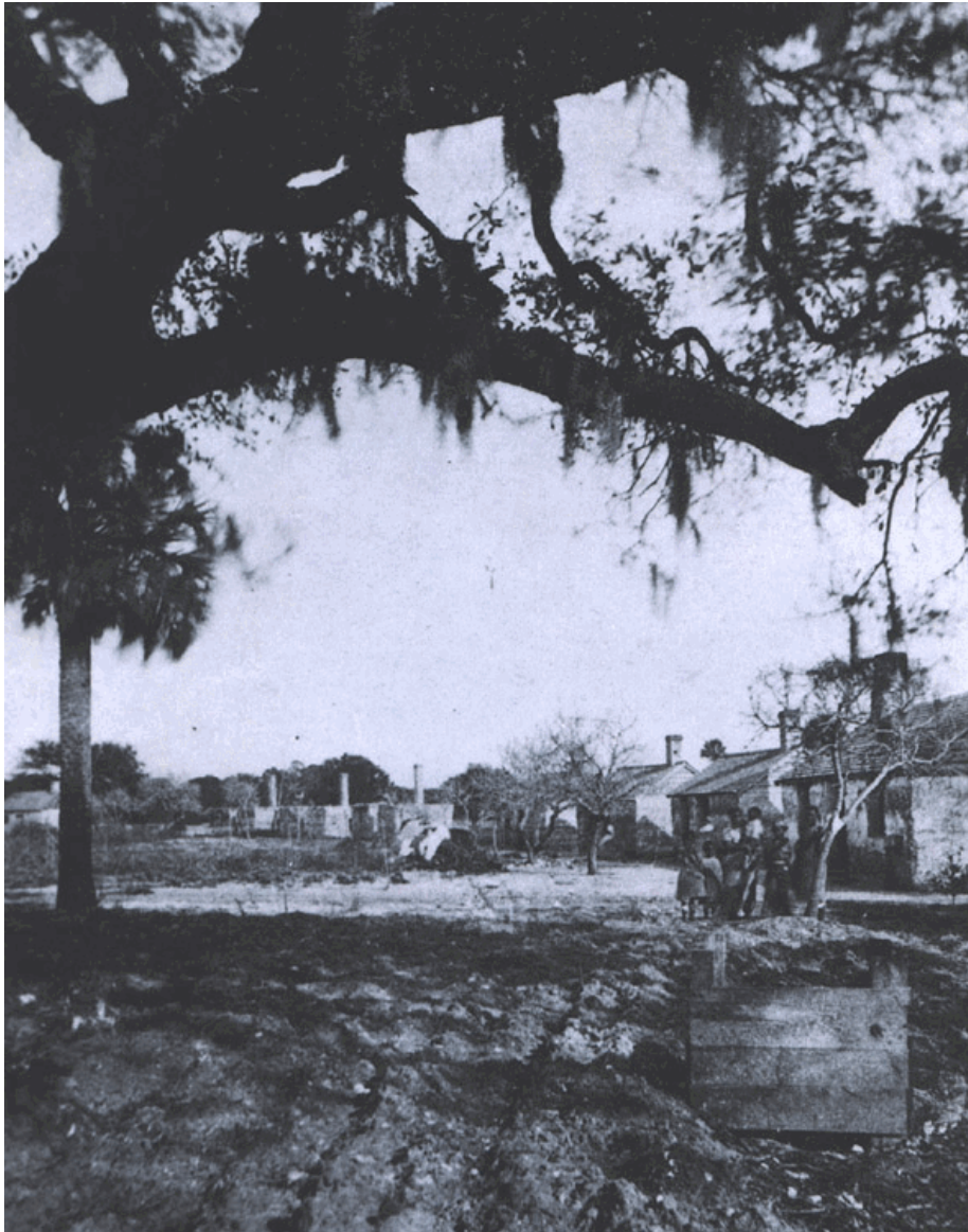
Figure 12: Mid-to-late 19th century photo showing tilled area and wooden well structure (confirmed by archaeological research) in front of Slave Cabins (Timucuan Ecological and Historic Preserve Collection, Courtesy of the Florida State Archives.)
