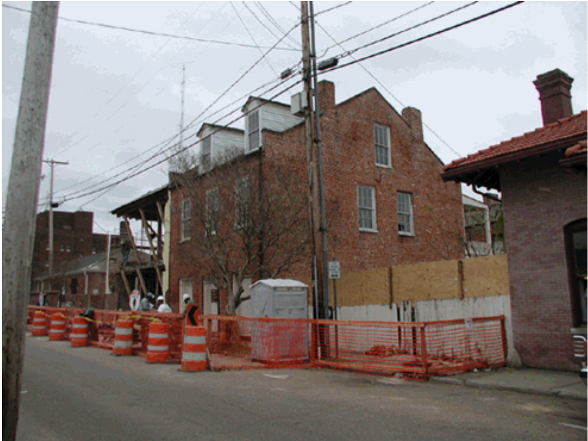
Figure 16: Vertical board fence enclosing west side yard.
