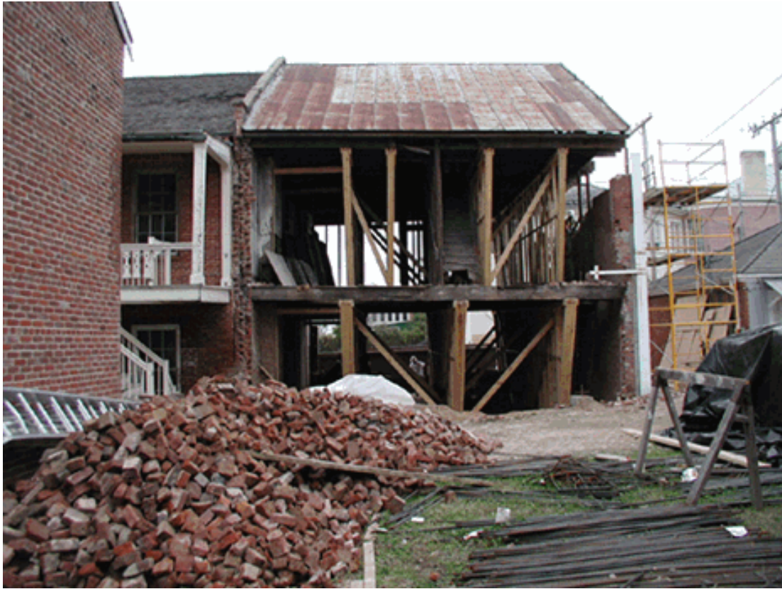
Figure 11: South rear facade of the McCallum House during renovation (January 2003).
