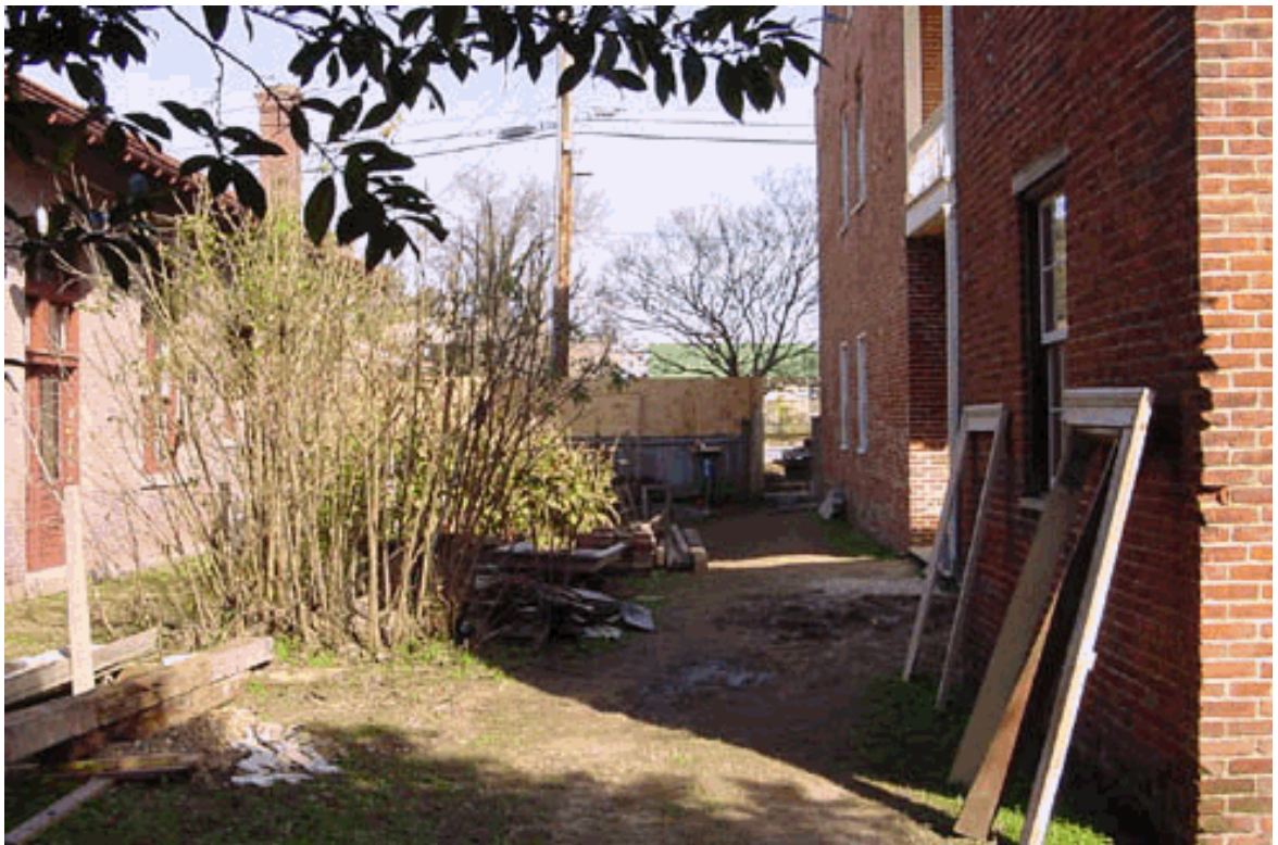
Figure 9: Side yard looking towards State Street with the west side elevation of the kitchen dependency in foreground.
