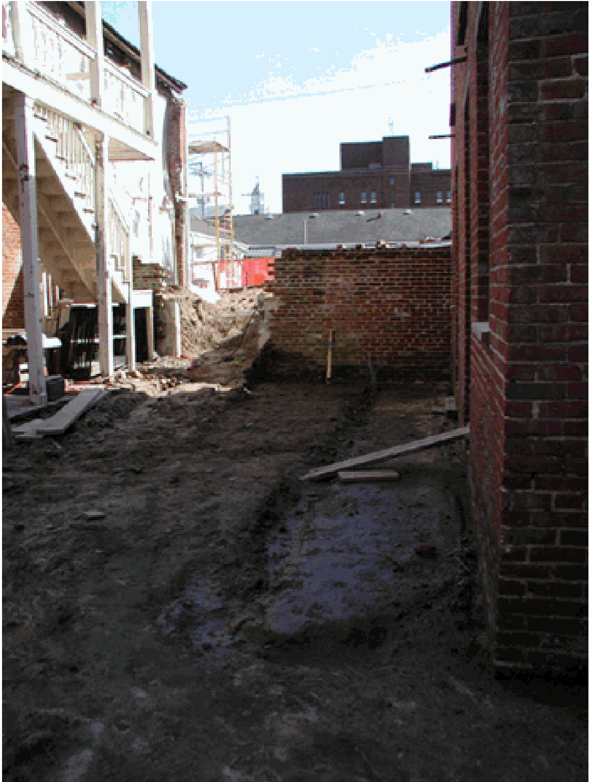
Figure 14: Retaining wall located in the east side yard.
