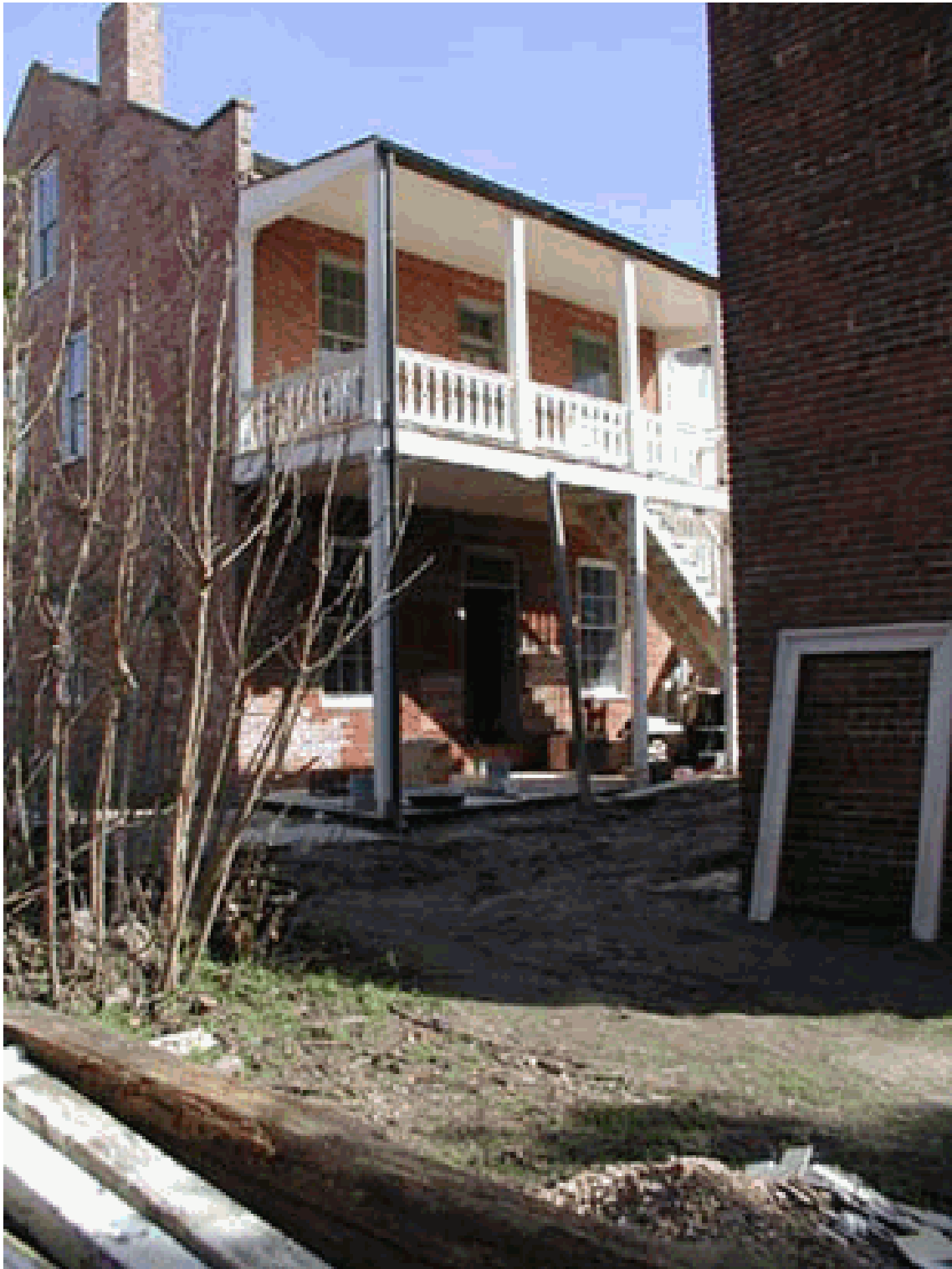
Figure 13: Rear porch of the William Johnson House.
