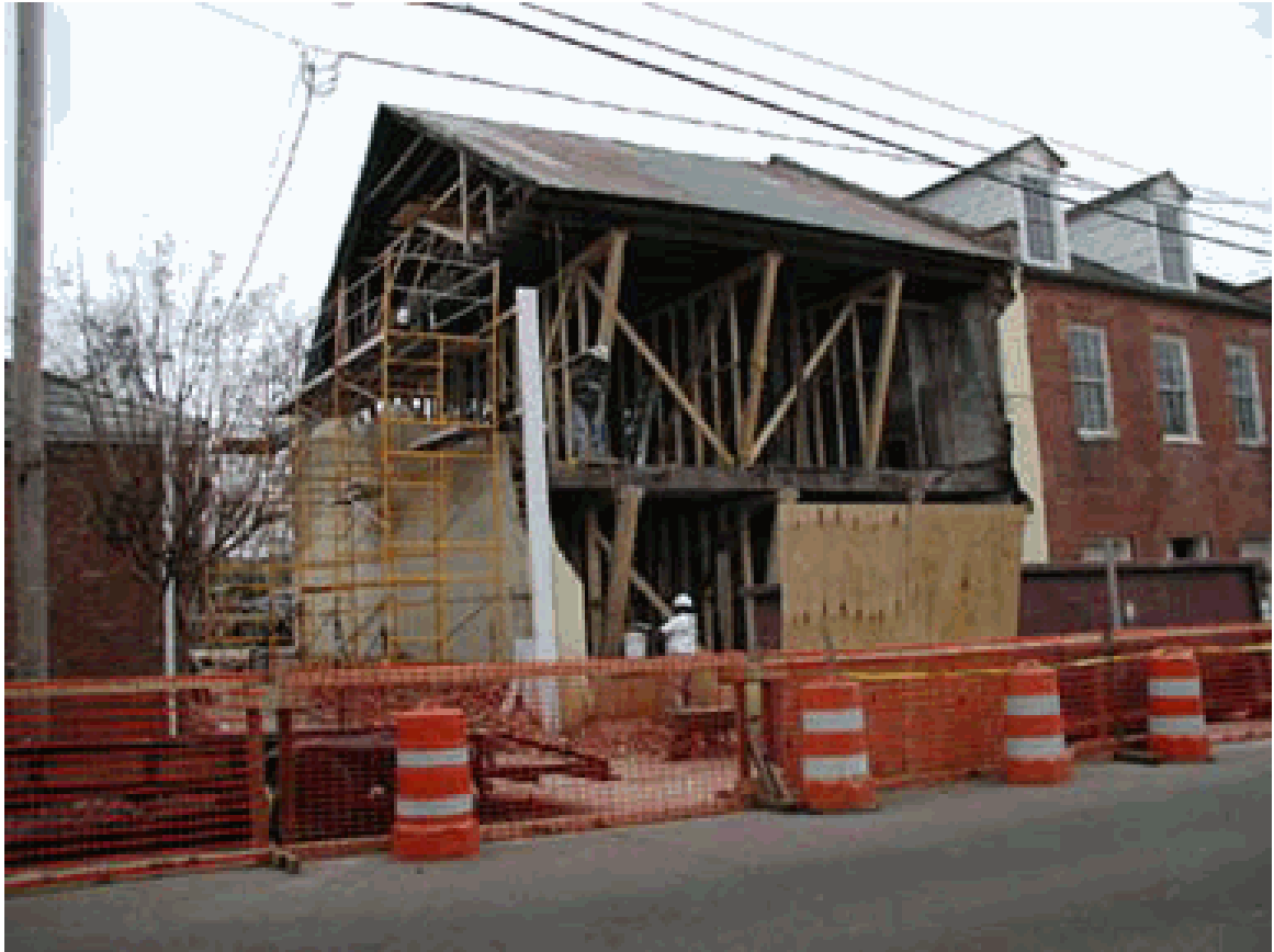
Figure 10: North front facade of the McCallum House during renovation (January 2003).
