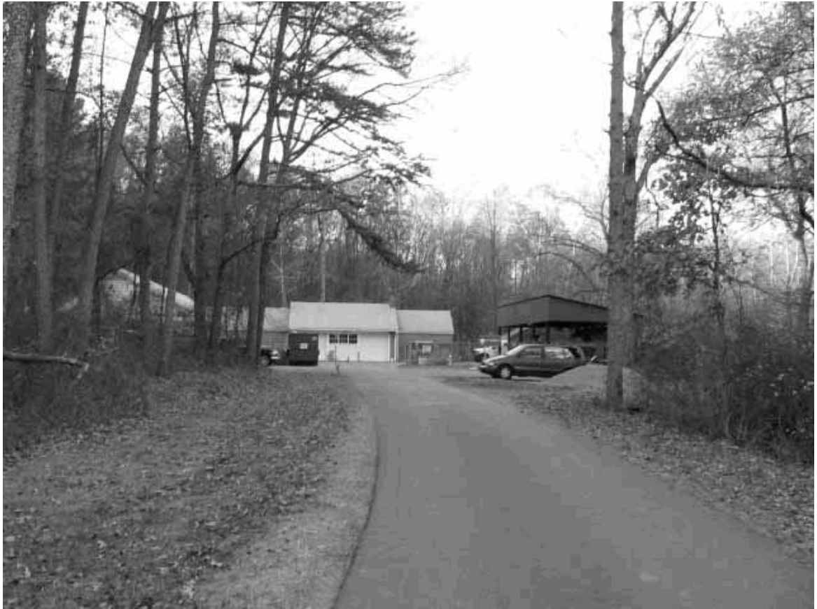
FIGURE 25. Maintenance Complex close to Visitor Center. Source: John Milner Associates, 2007.
