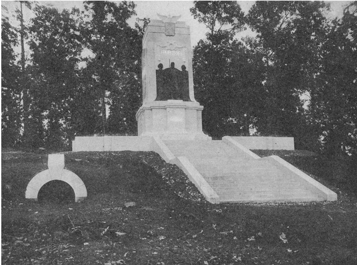
FIGURE 10. The Illinois Monument and the tunnel entrance arch shortly after its dedication. Source: NPS files at park.
