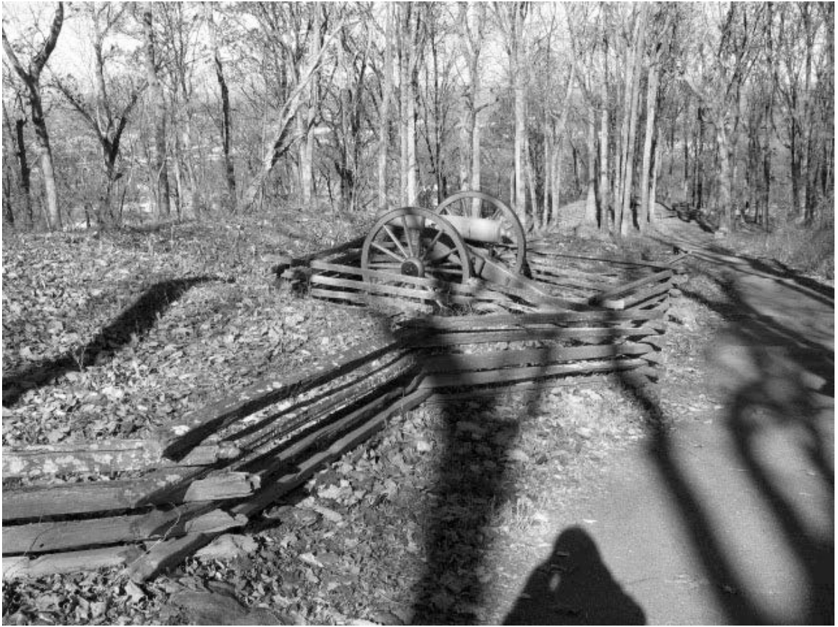
FIGURE 30. Snake rail fencing used to control access along the trail on Big Kennesaw Mountain. Source: John Milner Associates, 2007.
