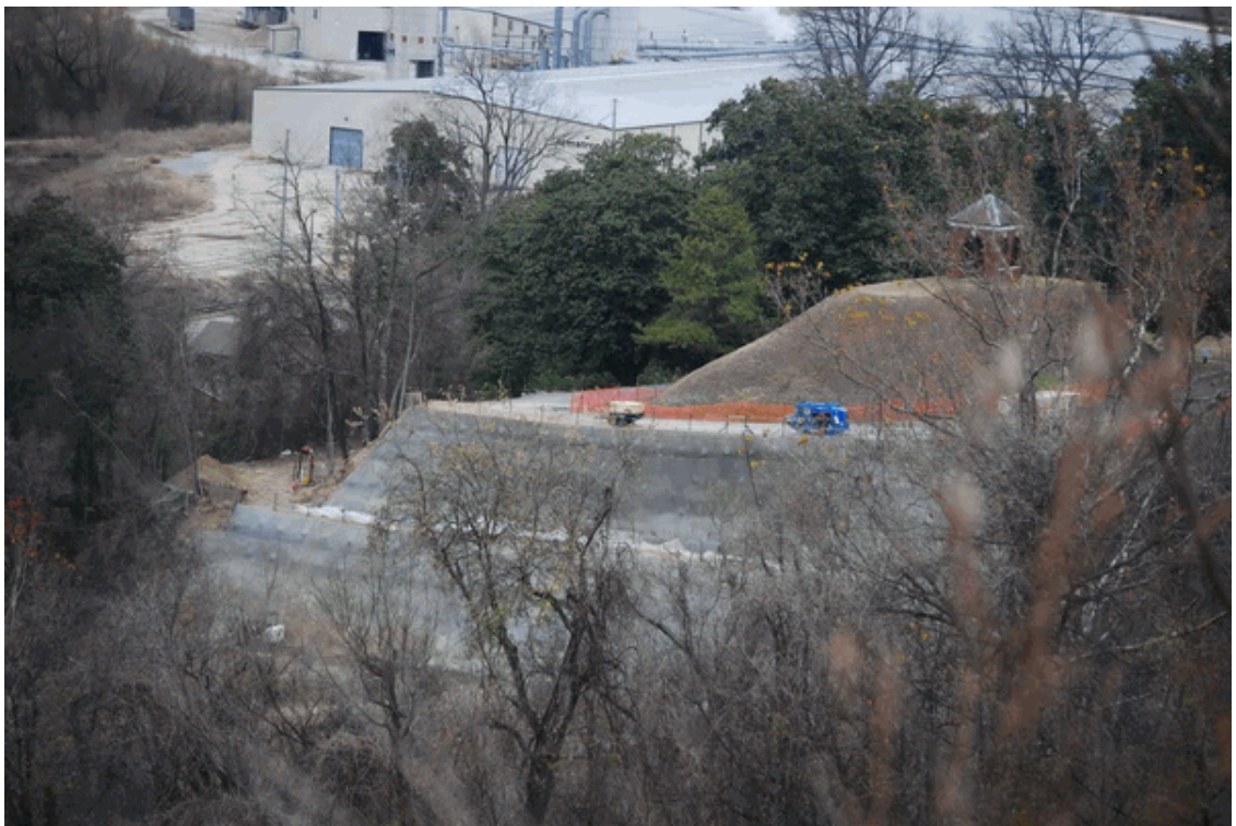
Stabilization work at the bluff above Mint Spring was completed in 2011. Source: Vicksburg National Military Park, 2011.
