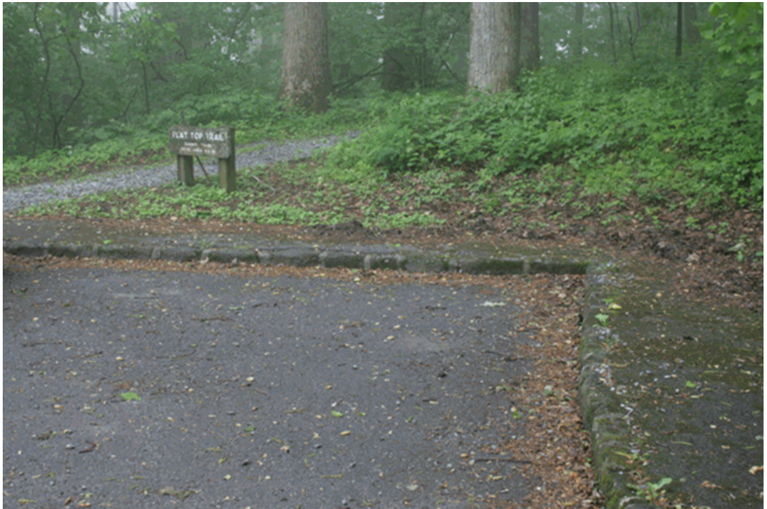
FIGURE 18. The asphalt sidewalk along the edge of the parking area at the Flat Top Trail parking area (2012 Peaks of Otter Cultural Landscape Report).
