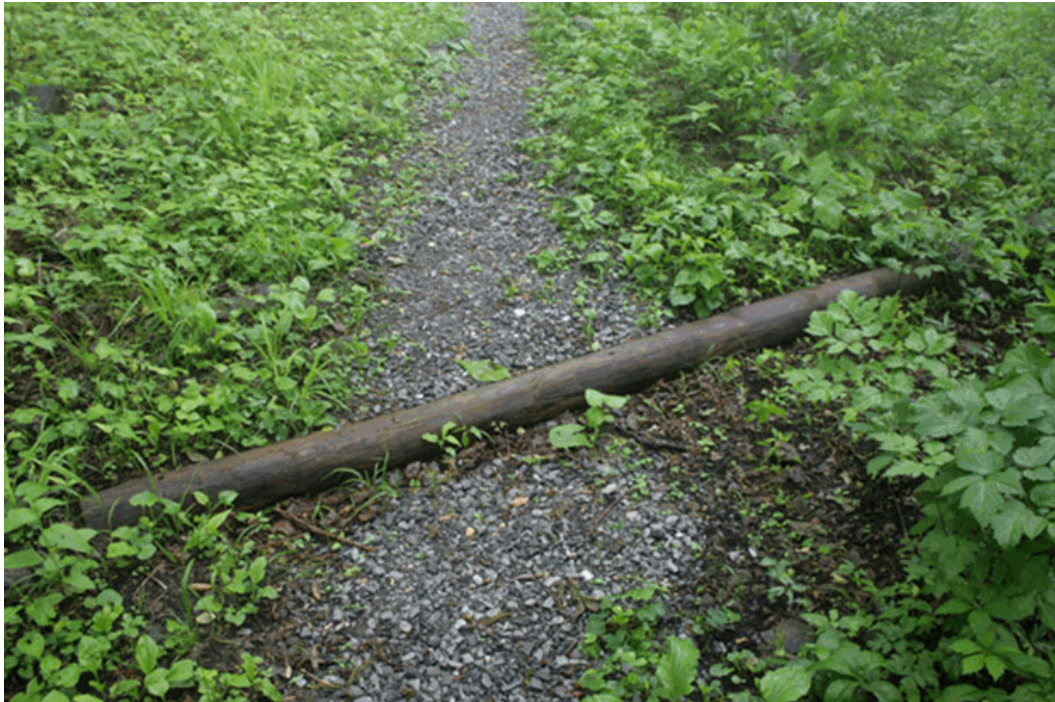
FIGURE 22. Waterbars are incorporated into the trails to direct the flow of storm water runoff (2012 Peaks of Otter Cultural Landscape Report).
