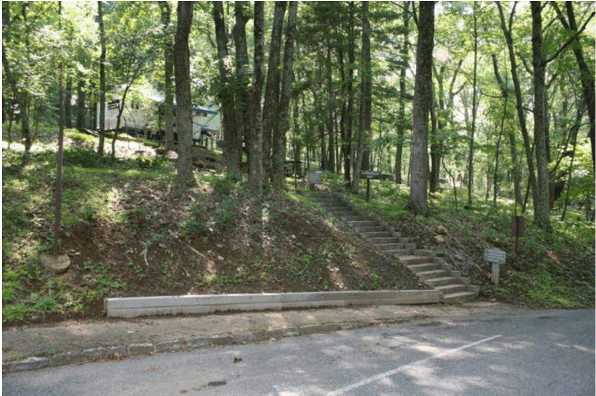
A longer set of steps composed of cast concrete slabs leads to the campground from the access road. (2012 Peaks of Otter Cultural Landscape Report)
