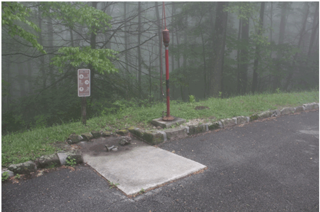
The campground dump station, where campers with recreational vehicles can empty their holding tanks. (2012 Peaks of Otter Cultural Landscape Report)
