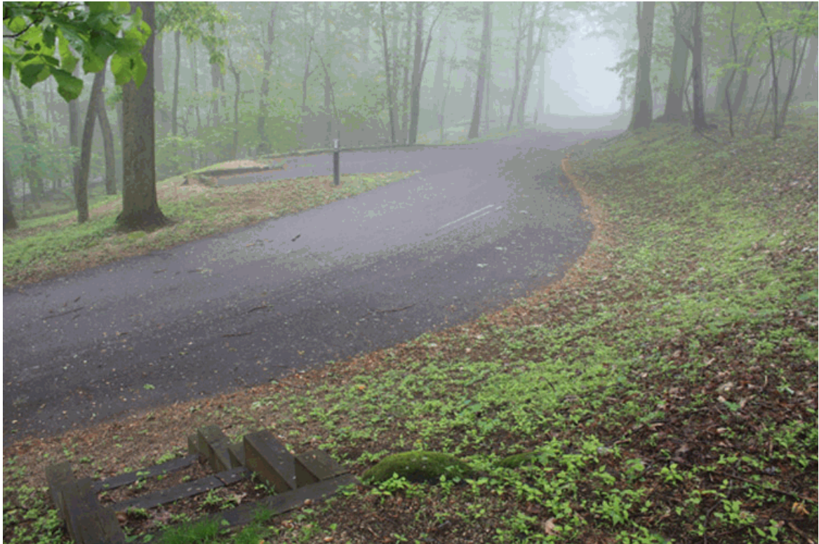
Asphalt parking spurs and trailer pull-offs branch from either side of the camping loops. (2012 Peaks of Otter Cultural Landscape Report)
