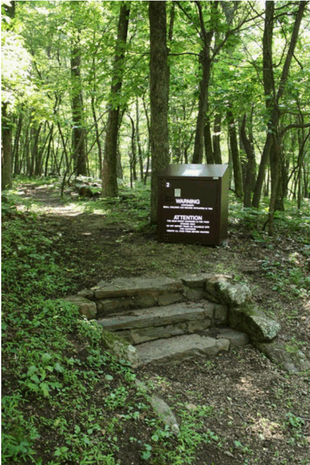
Some of the native stone steps were constructed with cheek walls. (2012 Peaks of Otter Cultural Landscape Report)
