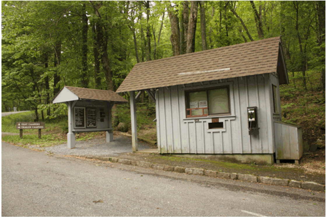
A stone-edged asphalt sidewalk runs alongside the entrance station. (2012 Peaks of Otter Cultural Landscape Report)
