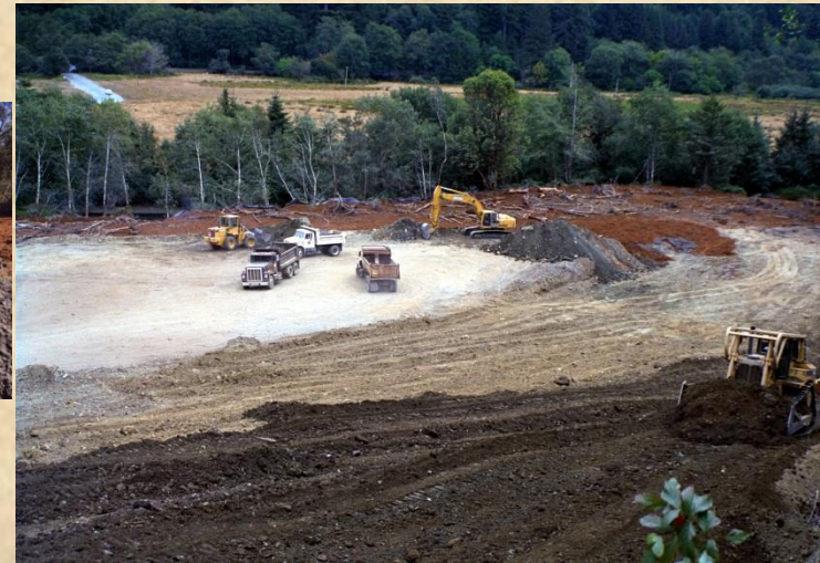
First Strip of Deck Excavation
