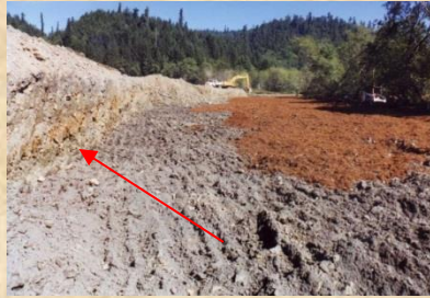
Contact of Deck Fill and Wetland Soil
