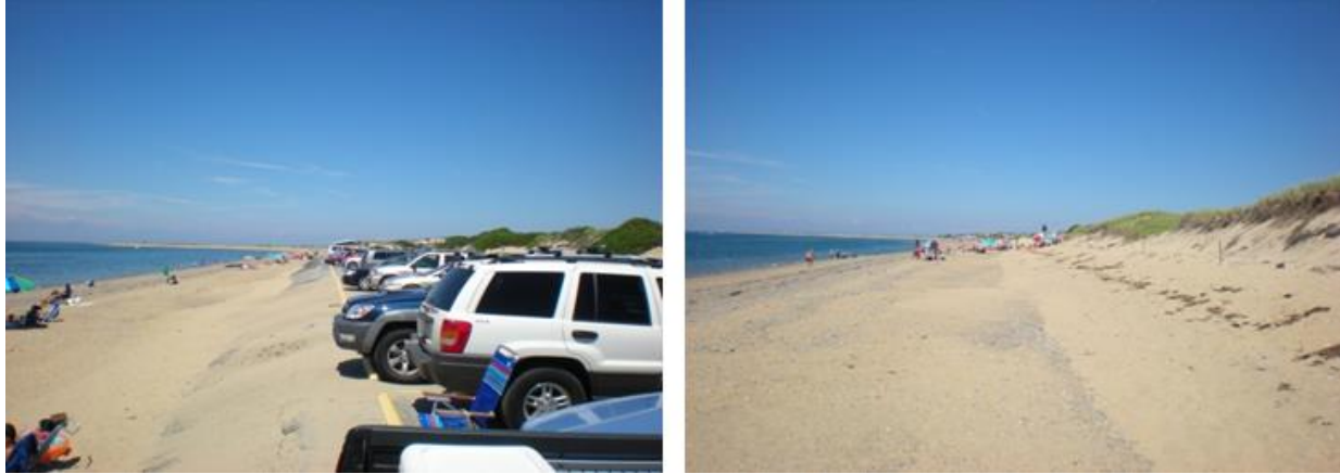
Figure 2. Two views of Herring Cove Beach, Cape Cod, showing effects of removing an asphalt revetment. The left panel shows the old road used as a parking lot and protected by the asphalt revetment (Wall 1, Table 5, Appendix A). The right panel shows the naturally-evolving shore where structures were removed.
