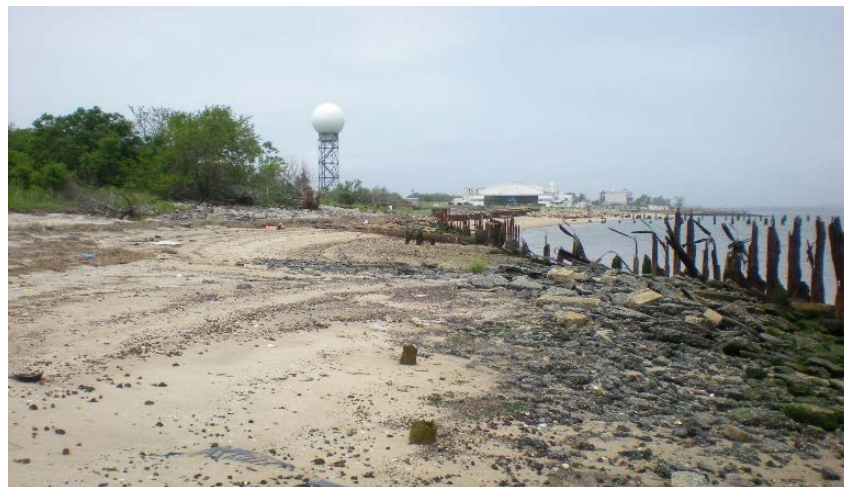
Figure 21. The evolving beach north of Ranger Road, showing the degraded bulkhead (Wall 4) and rip-rap that are interfering with exchanges of sediment and biota across the intertidal zone.
