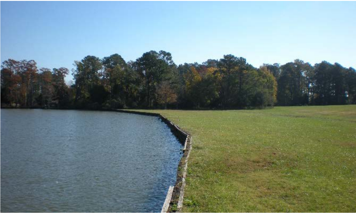
Figure 38. Bulkhead (southeast portion of Wall 6) protecting low grassy area landward of causeway to Jamestown Island in a location suitable for future marsh development.
