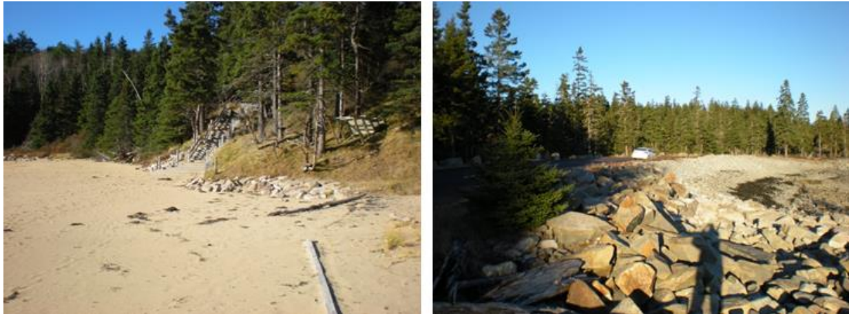
Figure 6. Acadia, showing Sand Beach, looking west toward the concrete walkway (left panel) and Wall 16 with angular riprap in the foreground contrasting with the gravel beach in the background (right panel).
