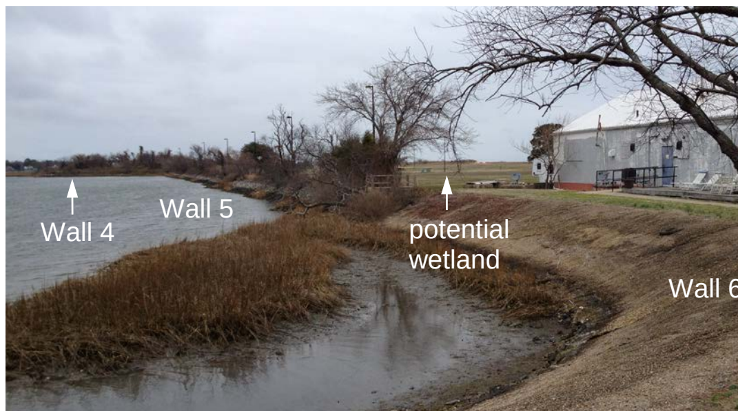
Figure 3. North end of Wall 6, looking north.
