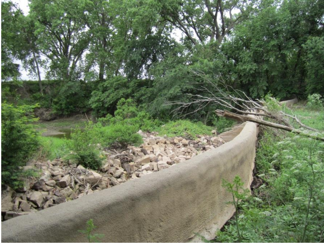
Figure 6. Concrete check dam located just downstream from FOLS. Note the height of the riverbed on the right (upstream) side of the dam due to sediment accumulation compared to the downstream riverbed height on the left (bed elevation difference of approximately 10 feet). Also note the presence of surface water in the riverbed on the downstream side, possibly indicating a connection between the channel and the water table there.
