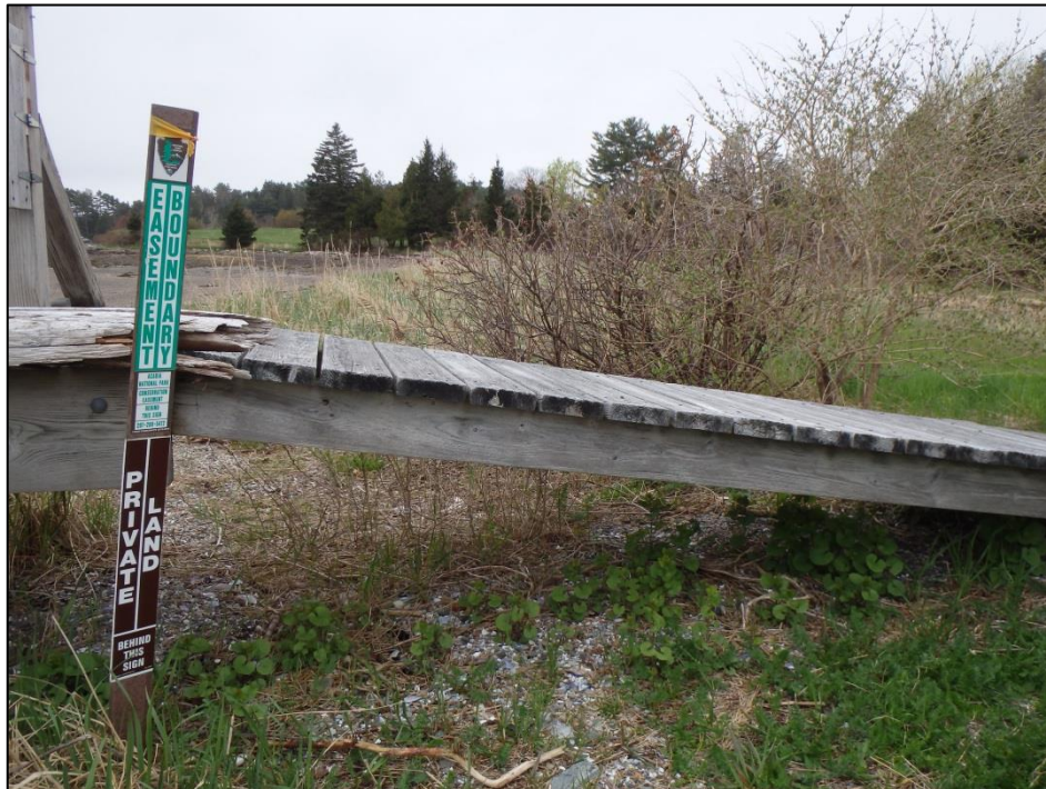
Figure 2. Cyclic maintenance is carried out in some locations, like this site on Fernald Point, in Southwest Harbor, ME. First-year leaves of garlic mustard ( Alliaria petiolata ) are seen growing underneath this ramp. Pulling these plants before they seed during their second year will reduce the seed bank and, over time, significantly reduce or eliminate this population (NPS photo, taken 05/15/2014).
