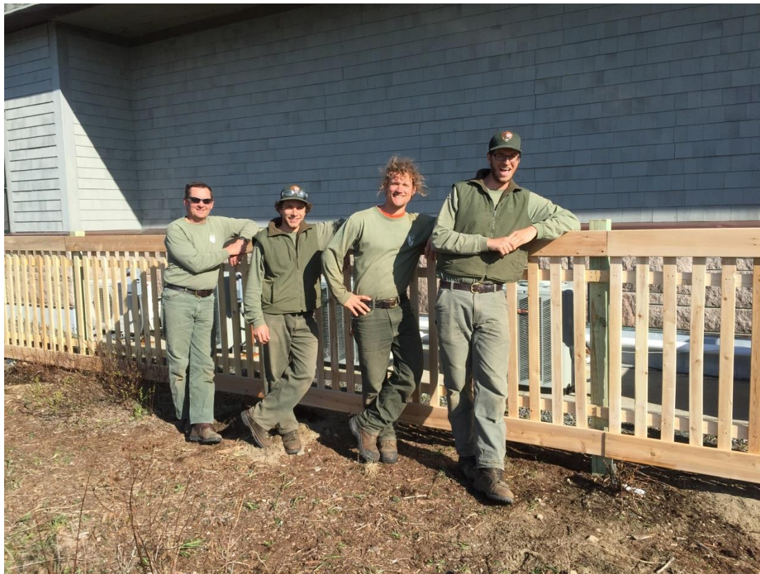
Figure 12. Team members and their newly built fence screening air handlers at the Moore Auditorium, Schoodic Education and Research Center, May 2015. (NPS Photo/Judy Hazen Connery).
