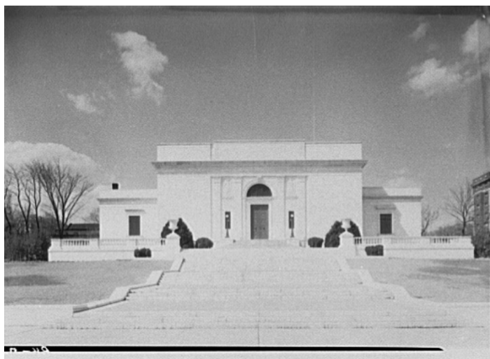
Figure 12 –This photograph appears to date from the period just after construction of the APhA headquarters, judging from the few plantings associated with the building. (Theodor Horydczak, "American Institute of Pharmacy," ca. 1934, Library of Congress, Prints and Photographs Division)
