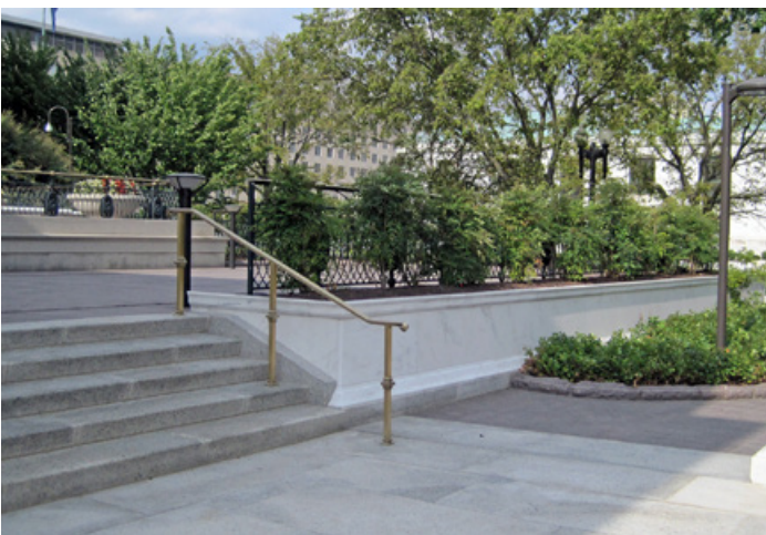
Figure 39 – Northeast courtyard raised and screened with heavenly bamboo.
