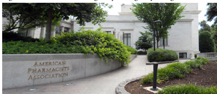
Figure 31 – Courtyard entryway on 23rd St.
