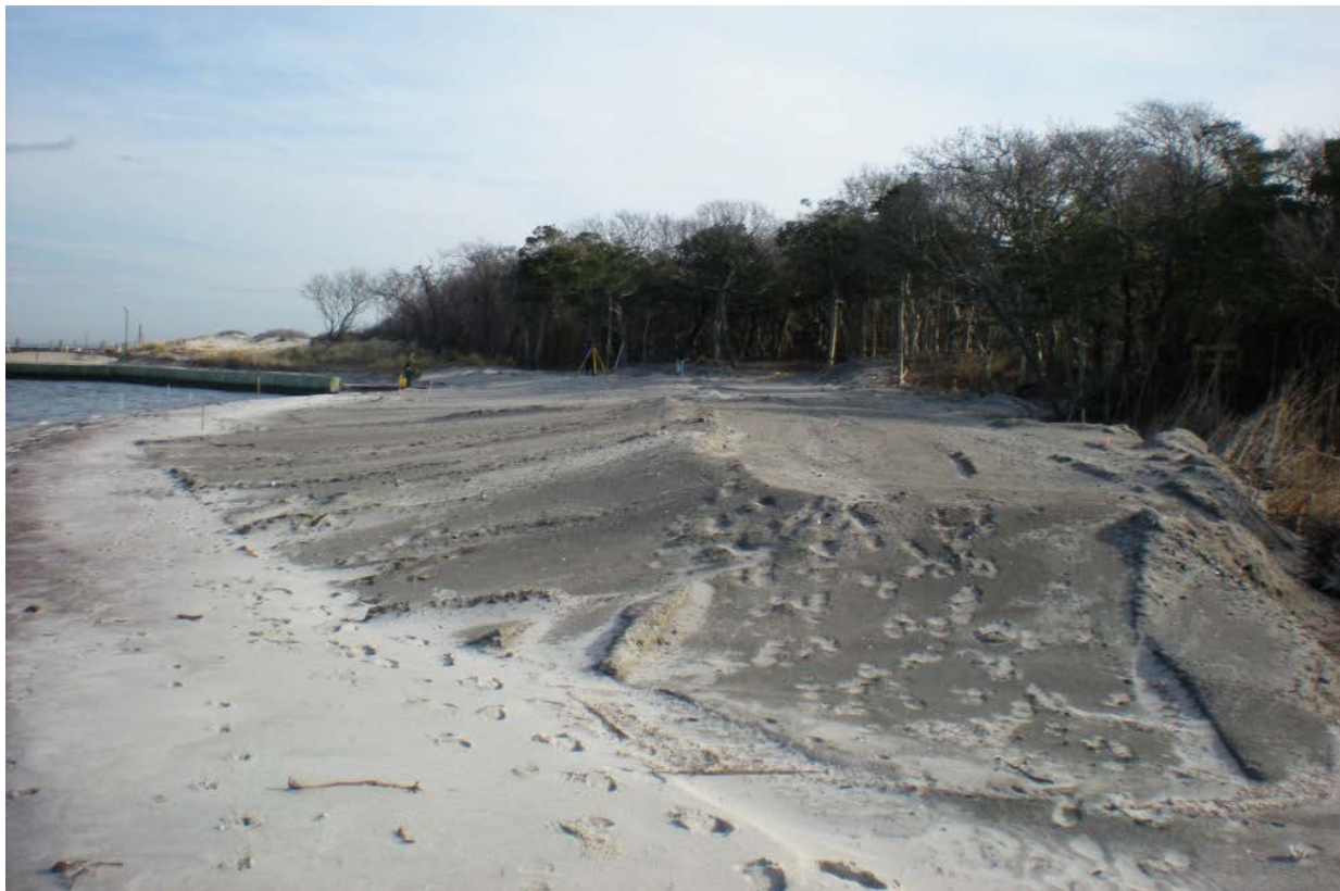
Figure 4. The shoreline west of the fill site, looking east on 20 November 2011, just after fill placement and reshaping by bulldozers.
