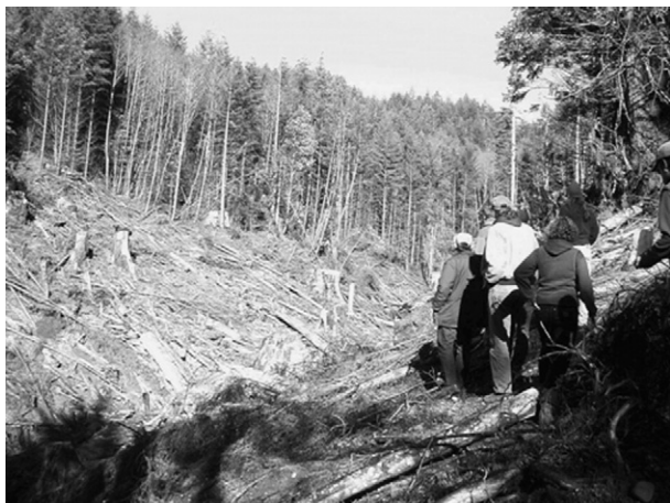
Fig. 4. Photograph of a newly excavated stream crossing following culvert removal from an abandoned logging road. View is looking upstream where the culvert and overlying road fill were removed and the streambanks pulled back to resemble natural topography. Stumps on the left side of the photo had been buried under road fill, but were exposed during the excavation. Following excavation, wood was placed on the banks and in the channel in order to control channel incision and streambank erosion.
