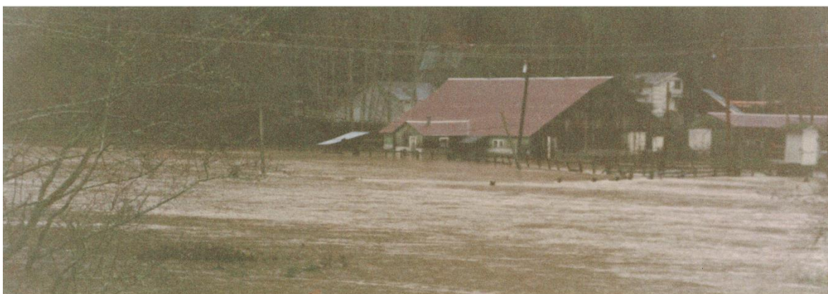
Figure 8: Barn and Mill A during the flooding event of winter 1996-97 (Courtesy of the Barlow family).
