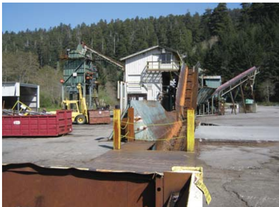
Hog fuel conveyor, view to the north
