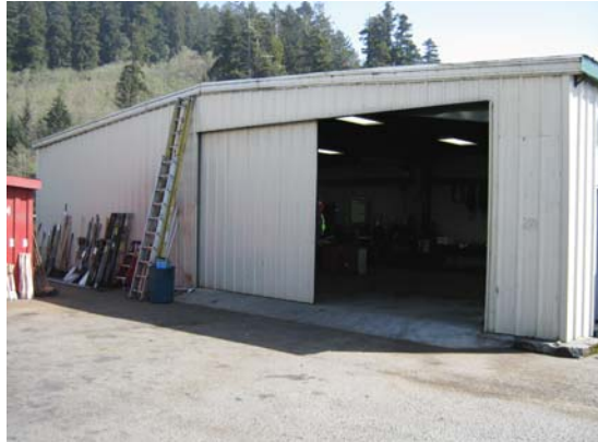
View to the northeast of modern metal framed shop
