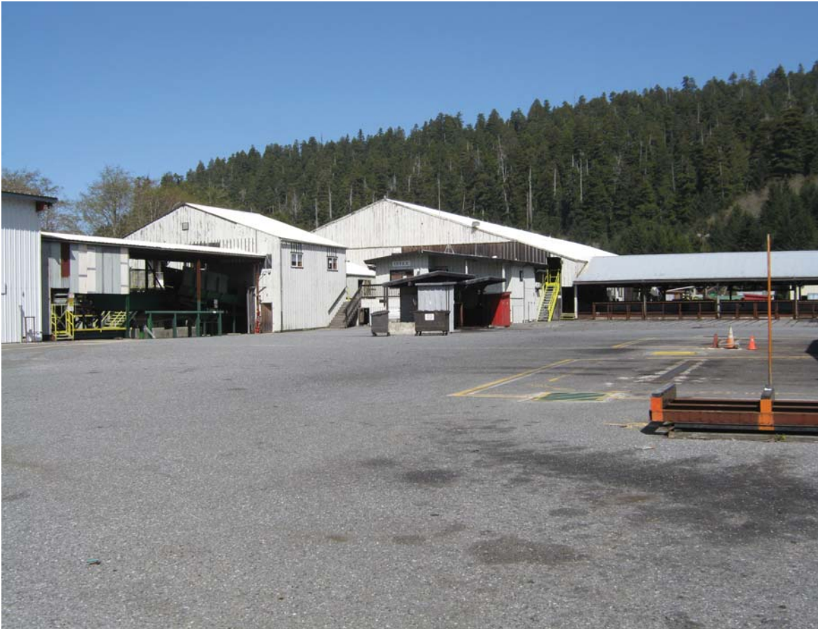
View to the north of Sawmill building.
