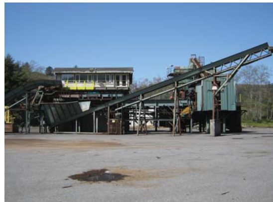
Hog fuel area, view to the west
