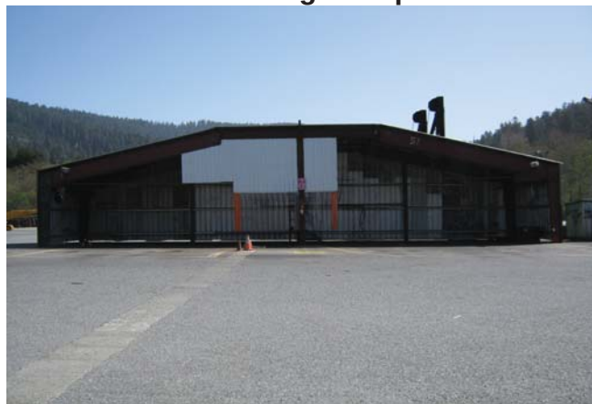
View to the south of spray shed
