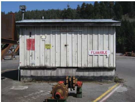
View to the northeast of oil house
