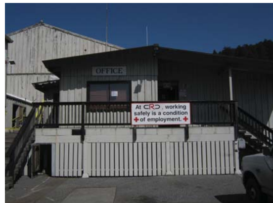
Company office, view to the northeast.
