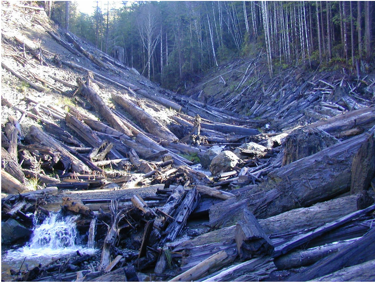
Figure 4. A stream crossing excavation with extensive woody debris placement. This photo was taken after the first winter following excavation.
