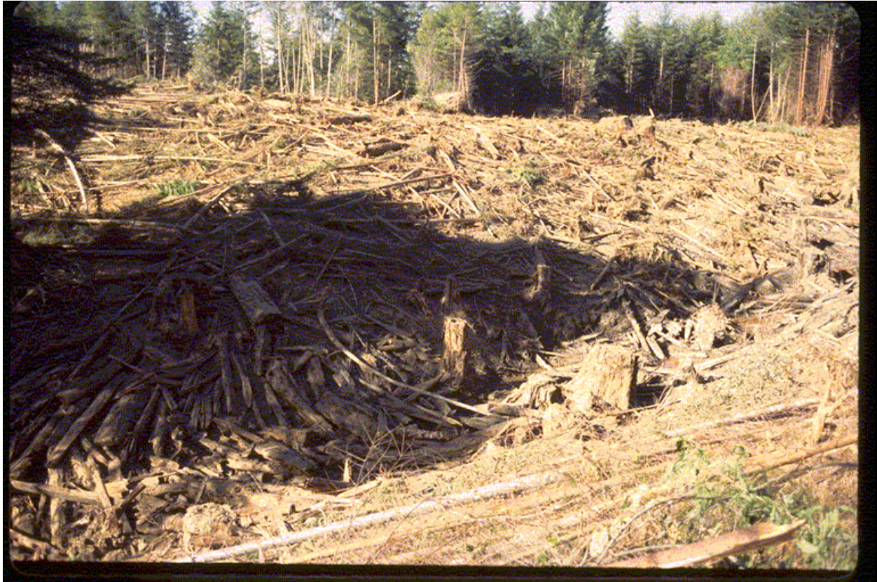
Figure 3. Vegetative debris mulching on excavation sideslopes provides for control of surface and fluvial erosion (this depicts a heavy rate of mulch application). Note the excavated stream channel with large woody debris placement in the foreground.
