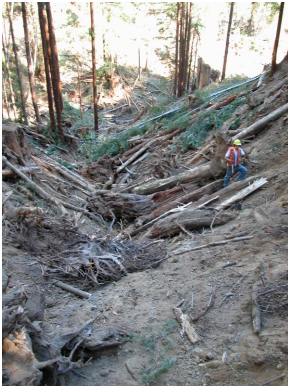
Figure 14. Work Item 23 (RX10, SBRX). Looking downstream from PT1 PP4 to finished RX10 and RX11 channels.
