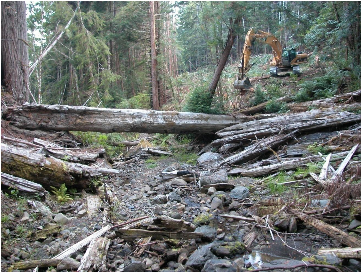
South Fork Lost Man Creek at former A100 crossing. Unit 08-02C, work item #39 at excavator. Pre-treat.
