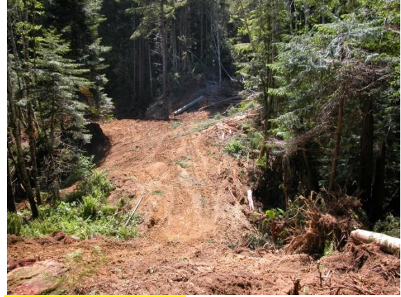
RX-6 partial excavation.
