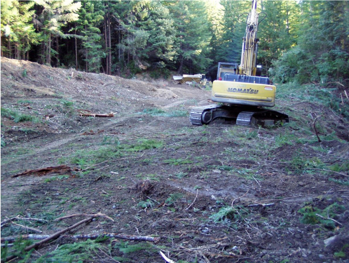
Photo E1, work item E14 where over 12,000 cubic yards of road fill was excavated and a new rock fjord crossing was installed on the Geneva road.
