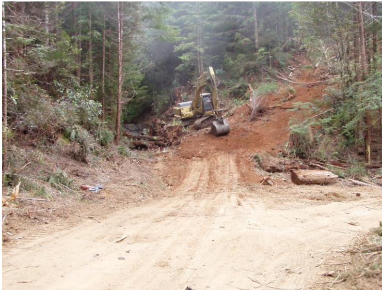
Photo C1, the upper portion of Work Item C5 RX excavation
