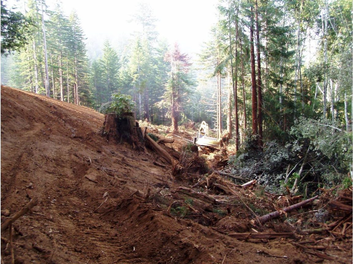
Photo C3, looking back at the ridge landing that instigated the additional excavation volume for work item C8.
