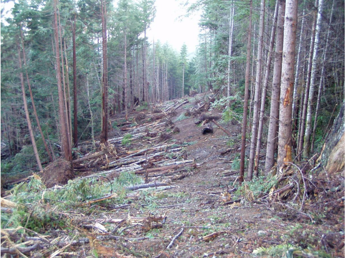
Photo F2, smaller swale above a skid road crossing excavation (work item F5)
