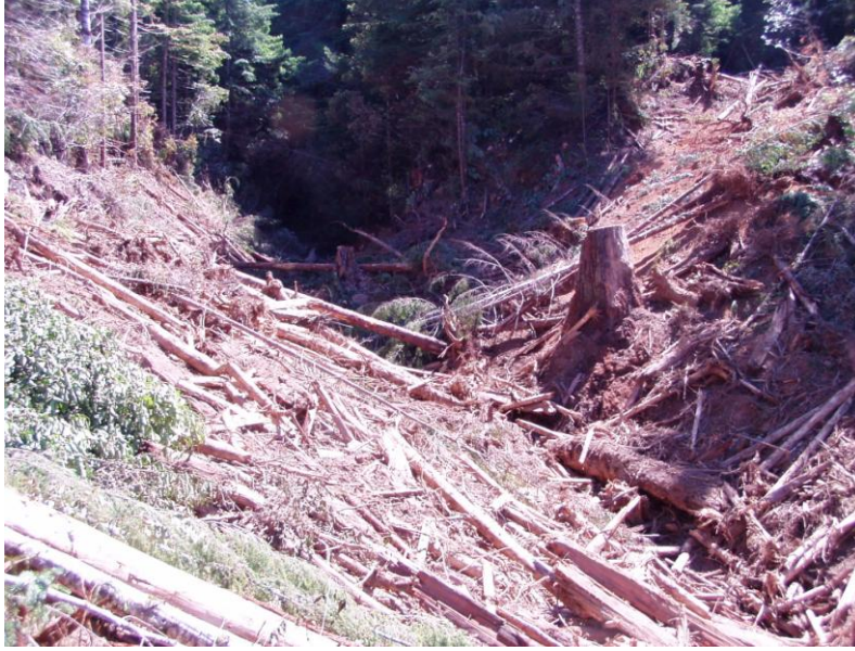
Photo C2, the completed Work Item C5
