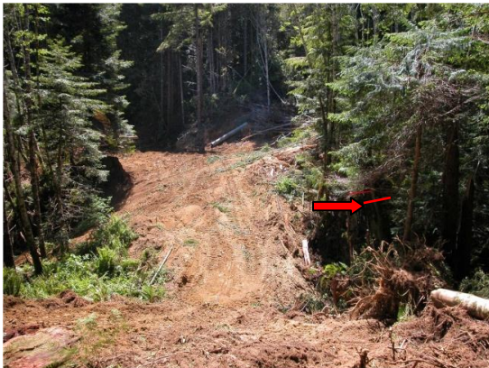
RX-1 opened for access. Looking Right Bank. June 17, 2008
