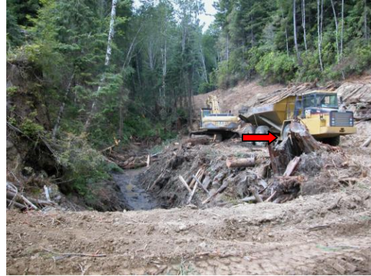
RX-1 Looking Up Stream. July 8, 2009.
