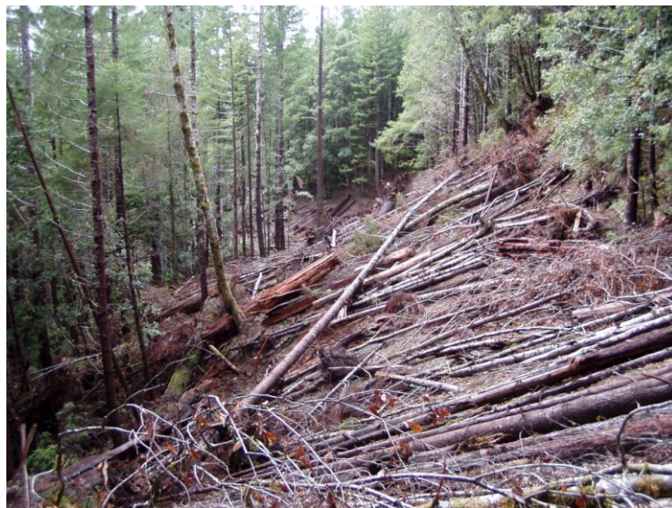
Image shows upper headwater swales following landform restoration. Photo was taken from Holter Ridge Road, looking down the previous A300 road alignment.
