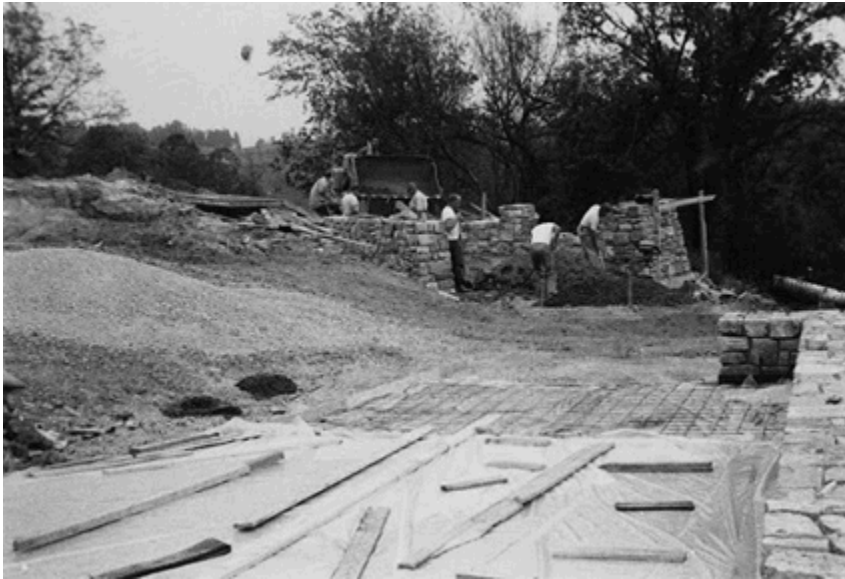
"1964 Overlook Terrace Construction." Image used from the Antietam National Battlefield Archives
