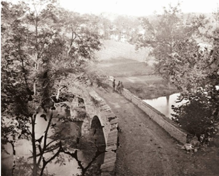
“1862 Wet Plate Photo by Alexander Gardner two days after the battle, showing damage to the bridge.” (From http://johngensorphotos.com/?tag=washington-county , accessed October 5, 2015)
