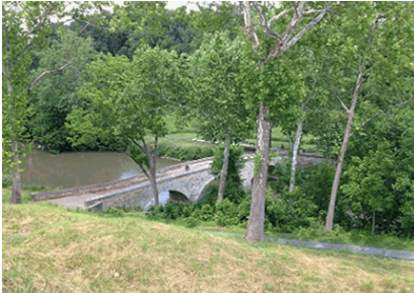
View from the Rifle Pit Overlook north and east to the Burnside Bridge and Antietam Creek. Photograph taken on July 21st, 2015.
