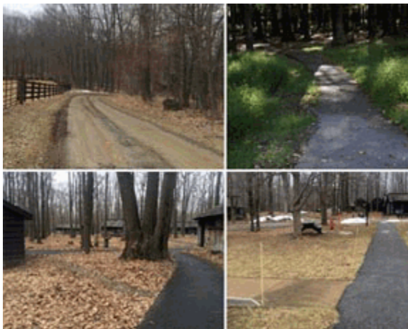
Camp Greentop current circulation patterns: main gravel loop road (top left), asphalt surfaced pedestrian trail (top right), social trail between cabins (bottom left), and concrete sidewalk to recreation hall (bottom right). (NCR)
