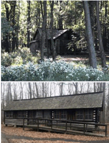
Contributing buildings and structures at Camp Greentop include the camping cabins (NCR).
