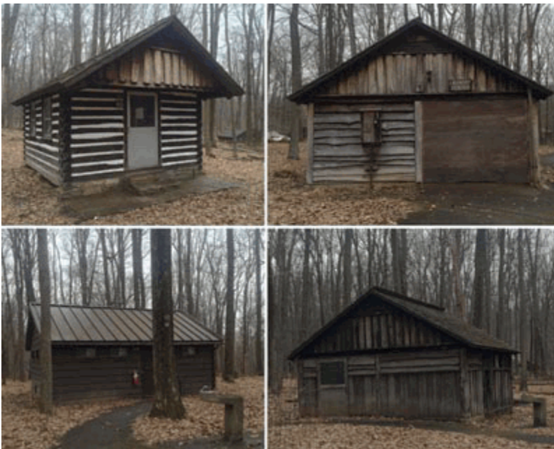
Buildings and structures: leader's cabin (top left), unit "A" latrine and laundry building (top right), non-contributing unit "A" comfort station (bottom left), and unit "B" latrine (bottom right). (NCR)
