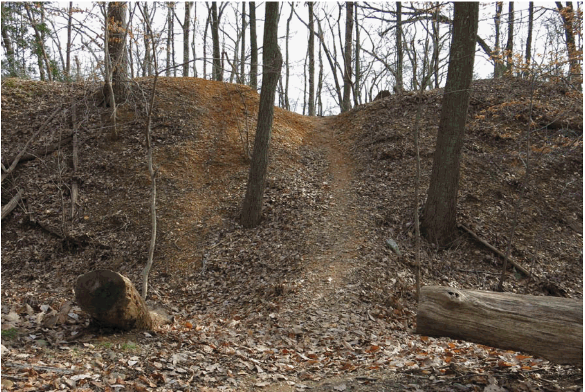
Fig 23 2014 North face earthwork with social trail.
