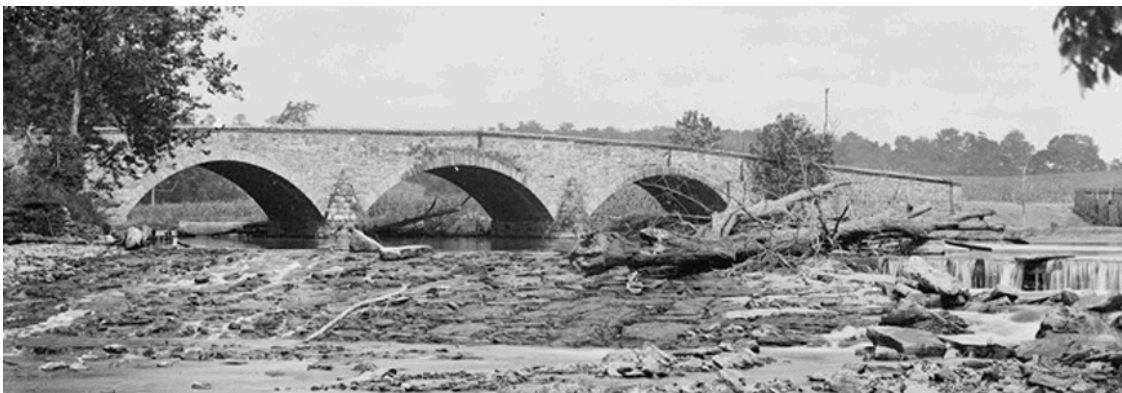
Middle Bridge looking upstream. Note the dam on the right, which appears to be damaged. (LoC, Aexander Gardner 1862)
