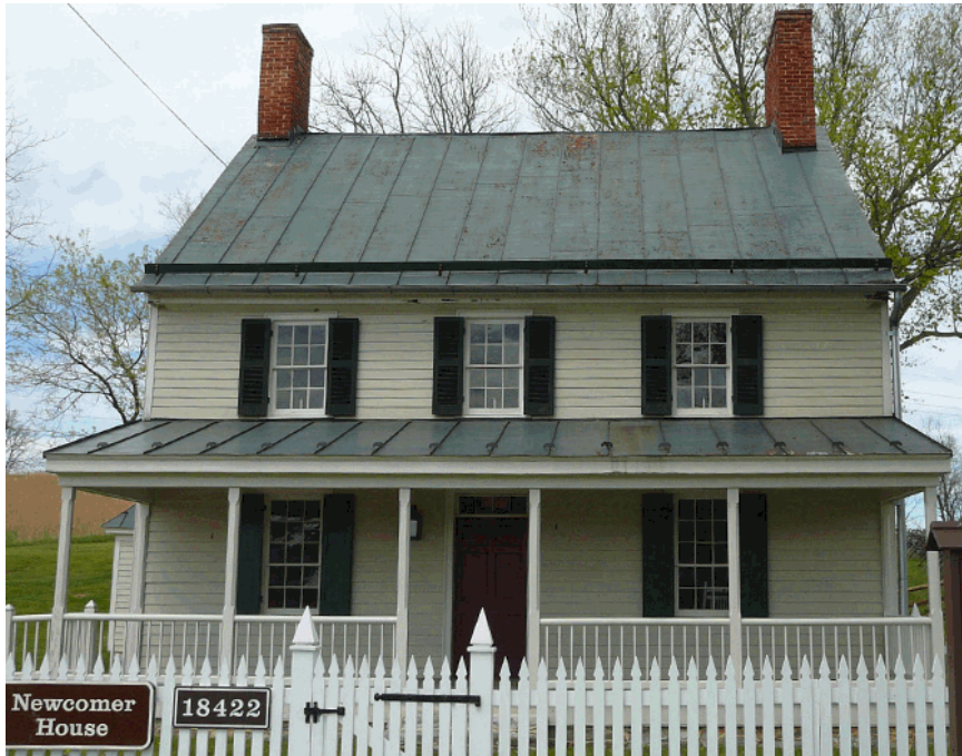
Newcomer House, Front elevation 2012 (NCR/CLP)
