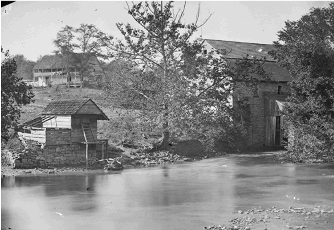
View of Orendorff House ( left-rear), and on the creek from left to right; an outbuilding and the Newcomer Mill (LoC, Alexander Gardner 1862)
