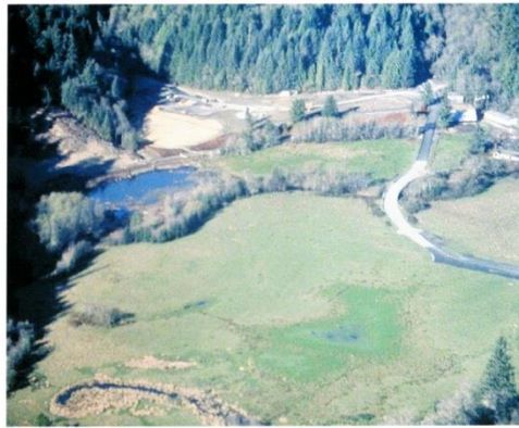
Mill B site after rehab 1999
