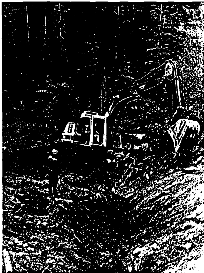
FIGURE 37. Heavy equipment at Sites 9 & 10.
