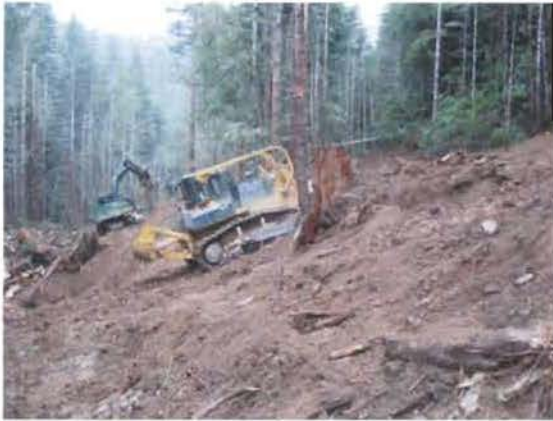
Photos 10 and 11: Outslope prescription, A100 Road. Left photo shows equipment in process of outsloping road. Right photo shows condition after excavation was completed.
