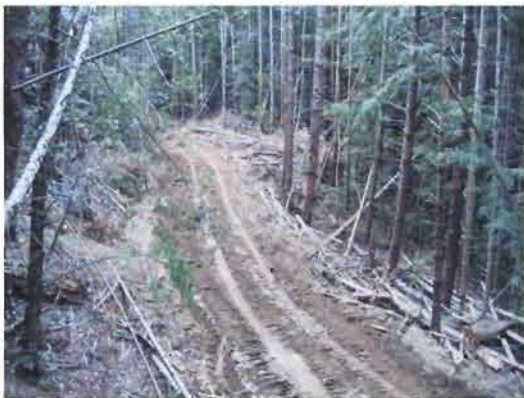
Photos 8 and 9: EOS prescription on the A100 Road. Left photo shows pre-existing condition with the center of the swale demarked by flagged (pink) tree on outboard edge of the road. Right photo is the final condition after swale has been excavated.
