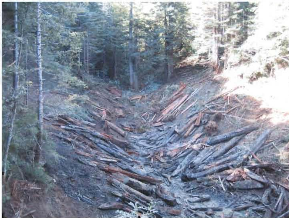
Photos 7: RX 1, A111 Road.
