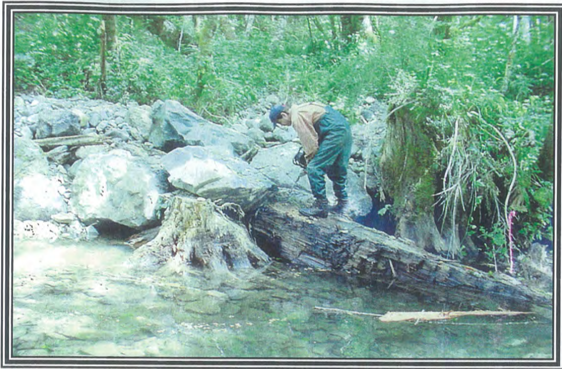
Plate #7. Dan Burgess anchoring a “Log-Rootwad-Boulder” instream habitat structure in South Fork Rowdy Creek, Smith River Basin.
