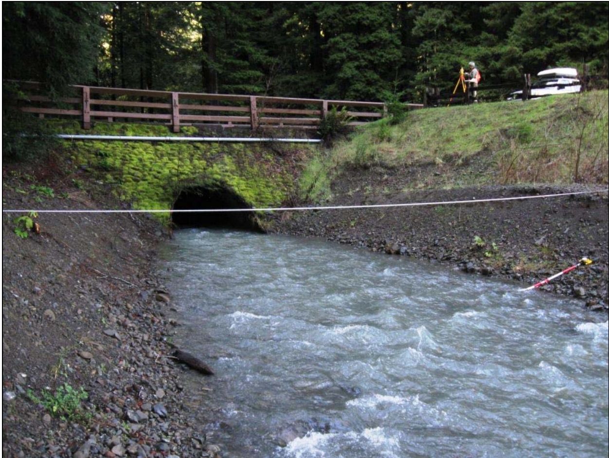
Figure 2. Example of tape location for measuring the tail-water cross-section, Durphy Creek #1 in Richardson Grove.
