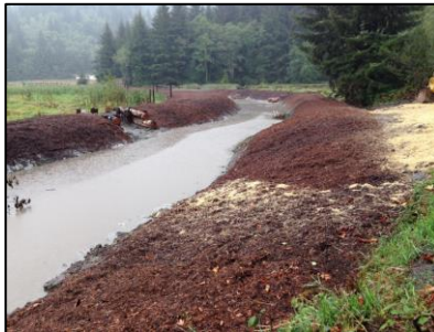
09/24/2014. Equipment work completed and mulch spread one day before first storm of year.
