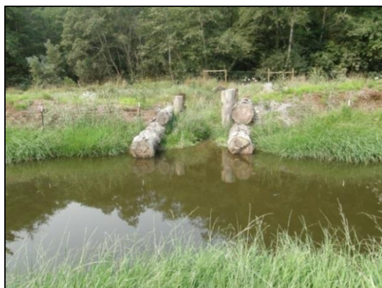
PP 53 (STA 2+90). View from mainstem right bank, looking directly across channel to left bank.
