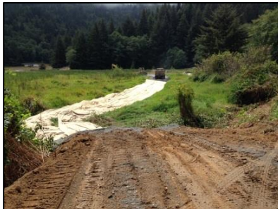
08/13/2014. Fabric (burlap) layer in place. Gravel being placed on top.
