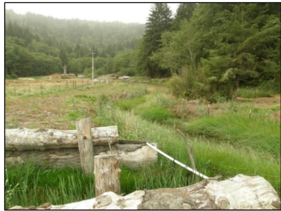
PP 57 (STA 8+30). View from mainstem right bank, on top of mound, looking obliquely upstream and across log crib structure that provides surface water flow conveyance between wetland and Strawberry Creek mainstem.
