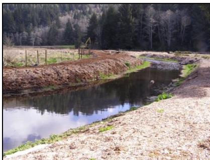
03/02/2015. Fence construction getting underway. Excavator in distance installing 12 ft. wood posts.
