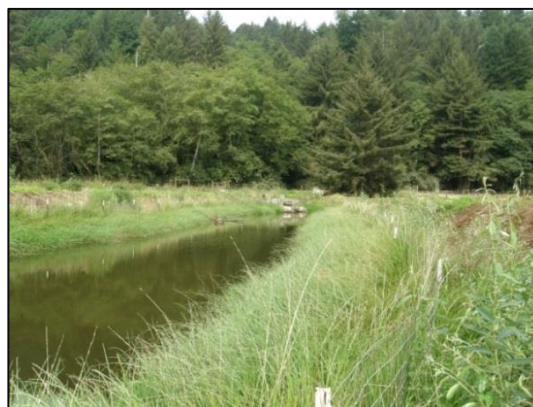
PP 54 (STA 4+50). View from mainstem right bank, looking downstream. Crib wall structure in distance is same as that in photo above.
