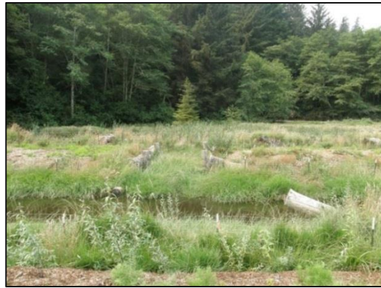
PP 55 (STA 5+50). View from mainstem right bank, on top of mound, looking across channel to crib wall structure on left bank.
