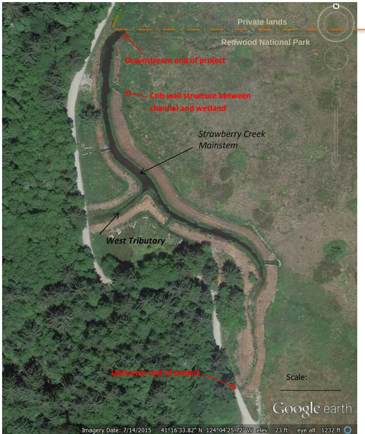
Figure D-1. Google earth image dated 7/14/2015 showing the project reach approximately nine months post-construction of Strawberry Creek mainstem and portion of West Tributary reaches. Visible in photo are the crib wall structures providing conveyance of flows between wetland and constructed channel, planting mounds covered with redwood bark mulch, open water channel of mainstem and West Tributary and invasive grasses lining the bank at the water's edge. The portion of the project not yet constructed is the culvert replacement on West Tributary and log structures upstream of the culvert.
