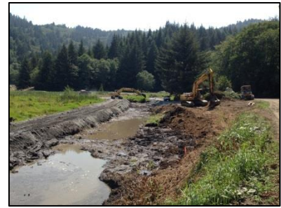
08/19/2014. Gravel portion of mounds in place allowing equipment access. Channel vegetation excavation in progress.
