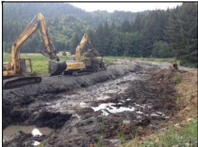
08/22/2014. Channel fill (clean, no vegetation) being excavated.
