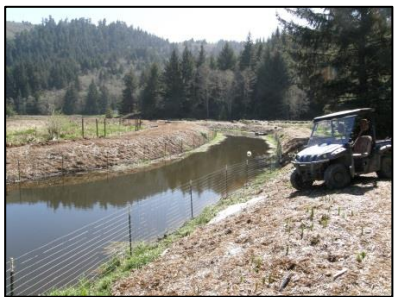
03/18/2015. Fencing construction in progress.
