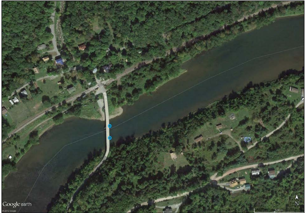
Figure 2. Aerial view of Lordville Road Bridge across Delaware River near Lordville, NY. The top circle, located near the primary river flow, outlines the Eastern Rivers and Mountains Network water quality monitoring equipment whereas the bottom circle outlines the United States Geological Survey river stage recorder.
