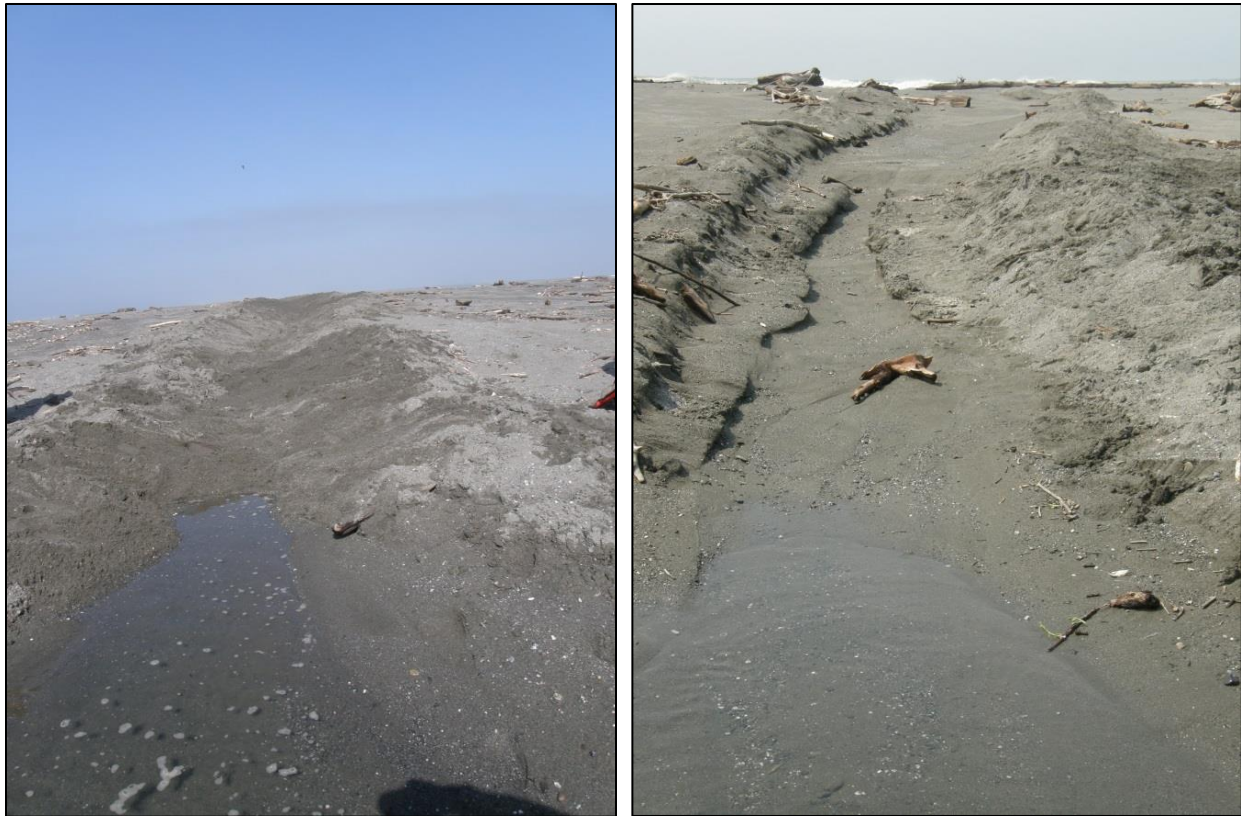
Figure 11. Ditch filled in from sides on August 19 (left) and results of wave overwash filling in more of the ditch with sand overnight on August 20, 2013. (RNP photo)
