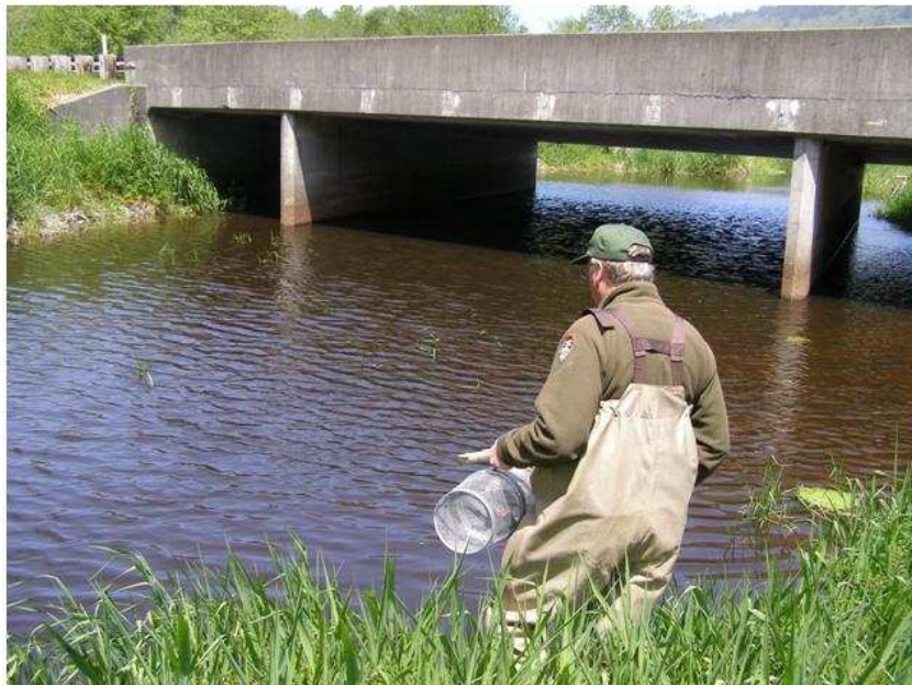
Upstream of Highway 101 Bridge on May 7, 2008 (RNSP).
