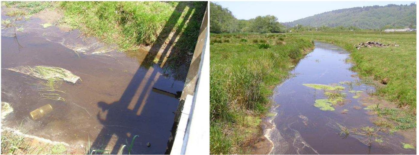
Wooden bridge sampling site at Barlow pasture (L) and Strawberry Creek channel downstream of wooden bridge through pasture (R) on May 7, 2008 (RNSP).
