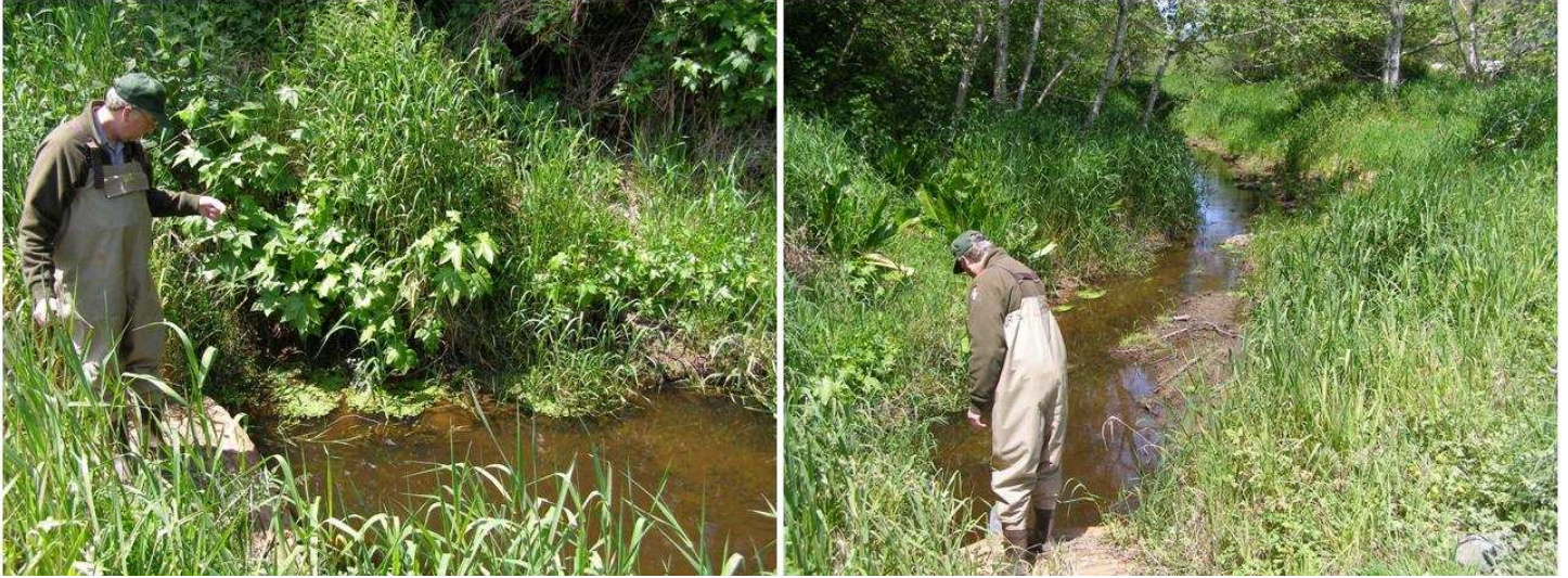
Downstream end of Hiltons Road culvert (L) and downstream channel (R) on May 7, 2008 (RNSP).
