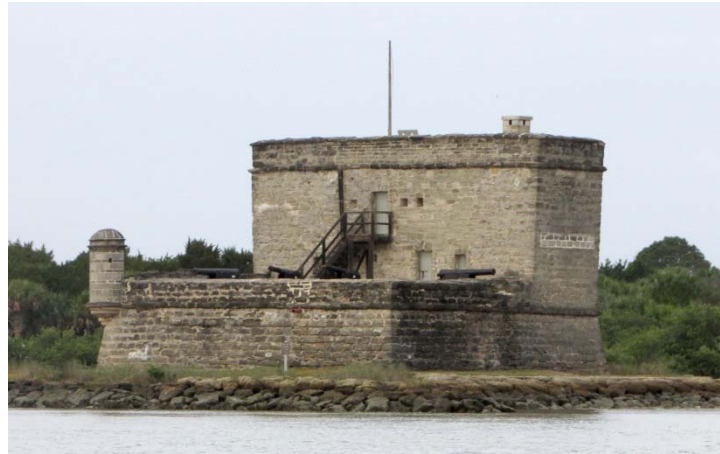
Figure 1: South and east elevations of Fort Matanzas viewed from ferry on Matanzas River (2016, Faisant Associates).
