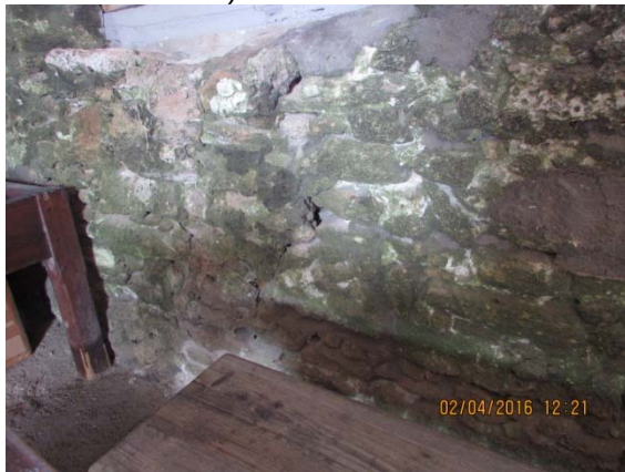
Photo C-5: Biological growth on north wall (2016, Faisant Associates).
