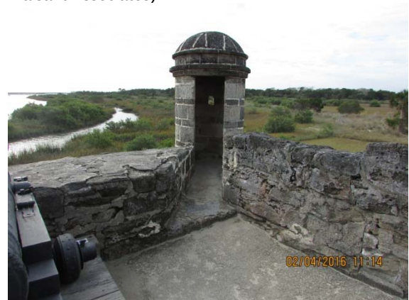
Photo B-6: Sentry box (2016, Faisant Associates).
