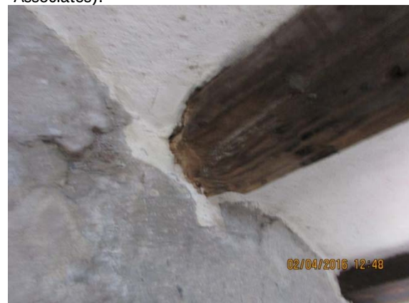
Photo D-4: Historic joist, bearing at south wall (2016, Faisant Associates).
