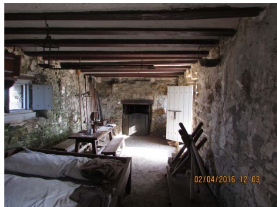
Photo C-2: First floor room, looking east (2016, Faisant Associates).
