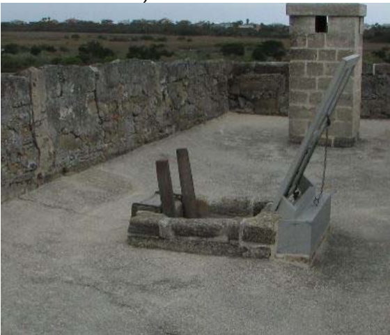
Photo F-3: Roof scuttle (2016, Faisant Associates).
