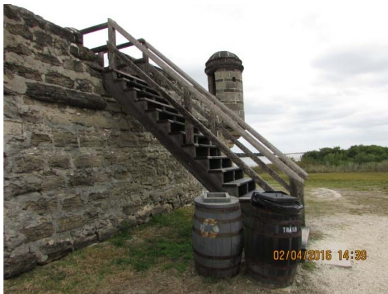
Photo B-7: Stair at Fort entrance (2016, Faisant Associates).
