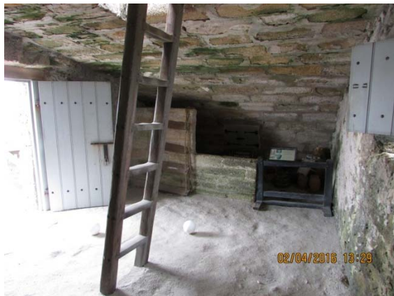
Photo E-1: Second floor room, looking west (2016, Faisant Associates).
