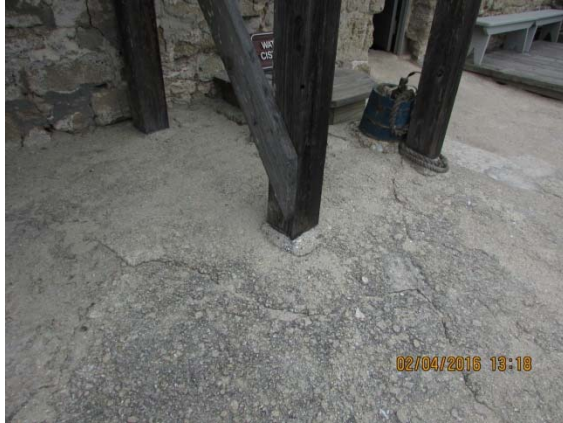
Photo B-10: Stair posts at terreplein deck support (2016, Faisant Associates).
