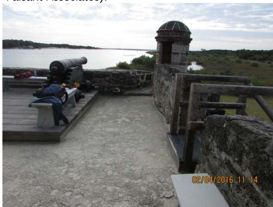
Photo B-3: Terreplein, looking south (2016, Faisant Associates).
