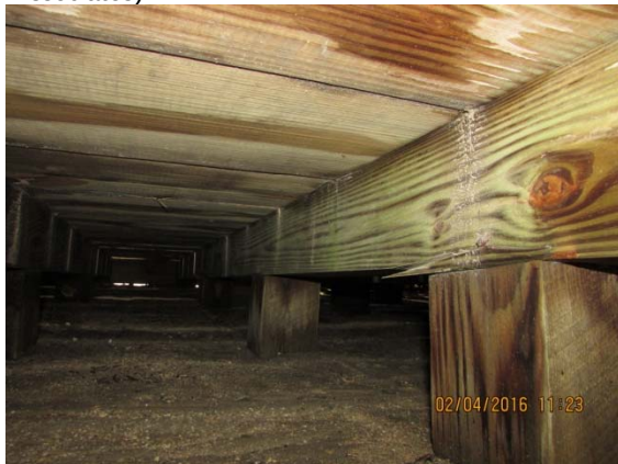
Photo B-5: Wood deck framing (2016, Faisant Associates).
