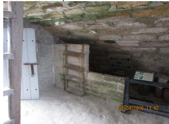
Photo E-6: Coquina partition wall (2016, Faisant Associates).
