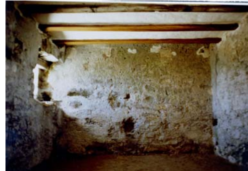
Photo D-5, above: First Floor Room looking west (1983, FOMA, M1890).
