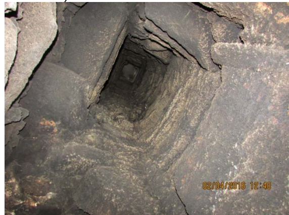
Photo C-6: Chimney flue (2016, Faisant Associates).
