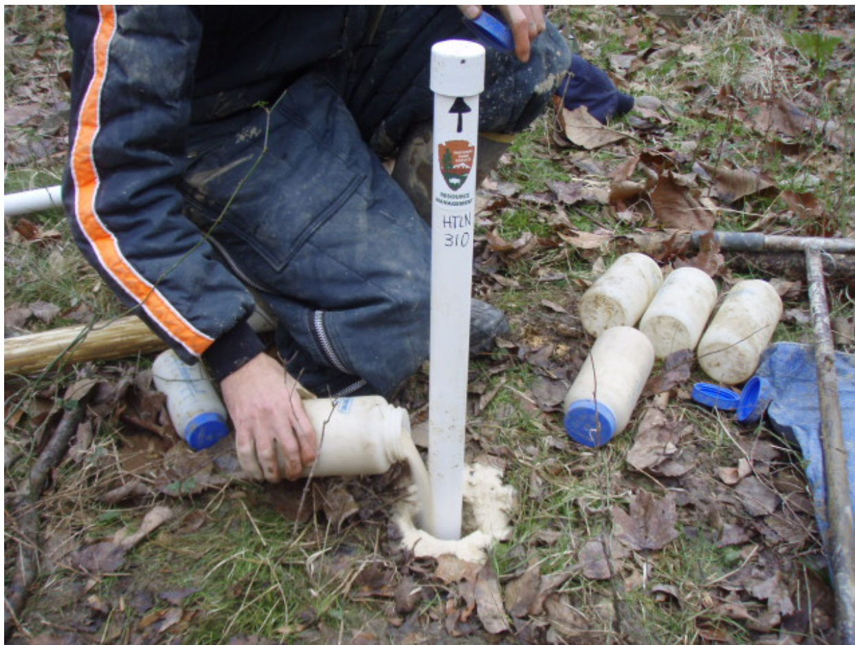
Figure 7.3. After the well is centered in hole, silica sand is sued to backfill the hole along the well screen. A layer of bentonite clay and soil backfill are the final layers.
