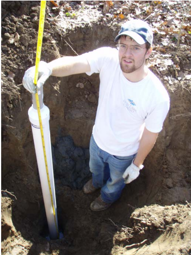
Figure 8.2. The Installation of an 80-inch logger may require hand-digging a hole. Silica sand is packed against the well screen using a concrete building form tube and the hole is backfilled with native soil.
