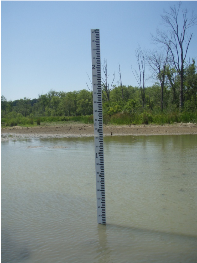
Figure 9.1. Installed staff gauge at Fawn Pond, Cuyahoga Valley National Park.
