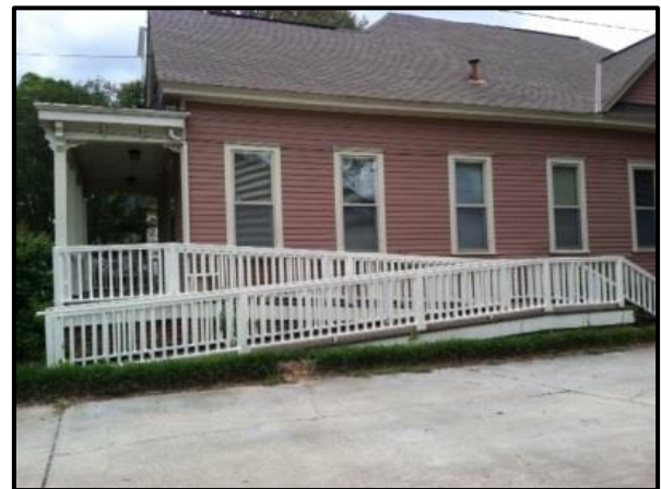
Figure 84: Example of Appropriate Placement of Handicap Ramp
