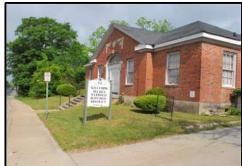
Figure 7: Gillespie-Selden Hospital Building
