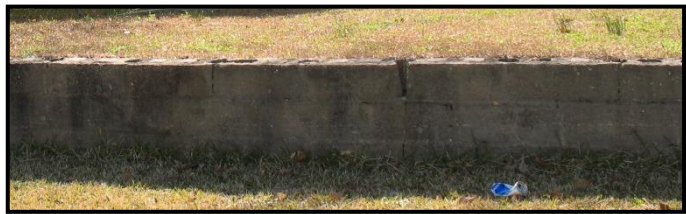
District Example of Cinder Block Wall
