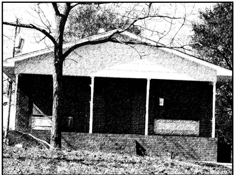
Figure 95: District Example of Brick Siding
