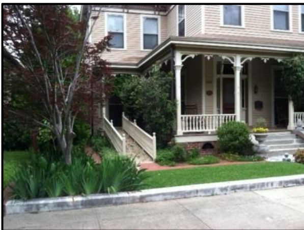
Figure 83: Example of Appropriate Placement of Handicap Ramp
