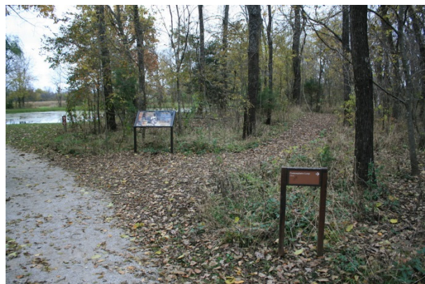
FIGURE 265. Wood chip mulch trail surfacing should be replaced with a material that meets universal accessibility standards.
