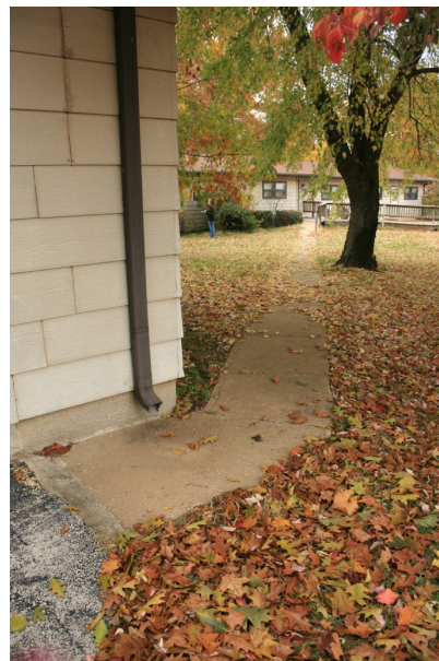
FIGURE 123. A concrete walk links two of the residences in the former housing/administrative area.
