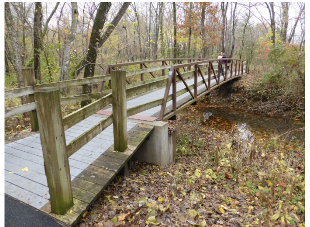
FIGURE 158. Bridge 1, view looking north and showing the approach ramp and bridge truss configuration.
