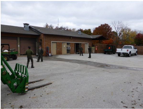
FIGURE 141. The maintenance building, view looking northeast from the maintenance yard.
