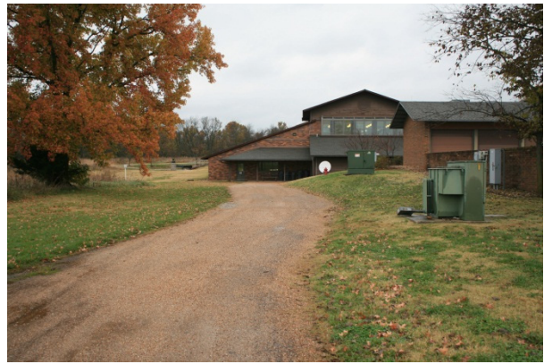
FIGURE 88. A gravel-surfaced road leads to the rear of the visitor center.
