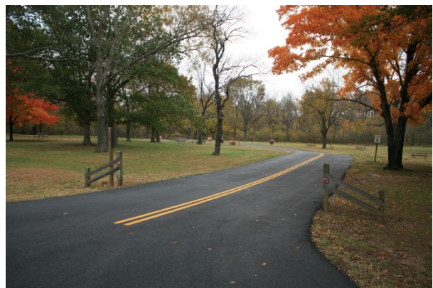
FIGURE 89. The paved picnic area spur road leads north from the park entrance road.
