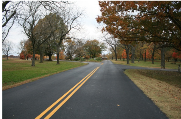
FIGURE 80. The park entrance road as it passes the picnic grove.
