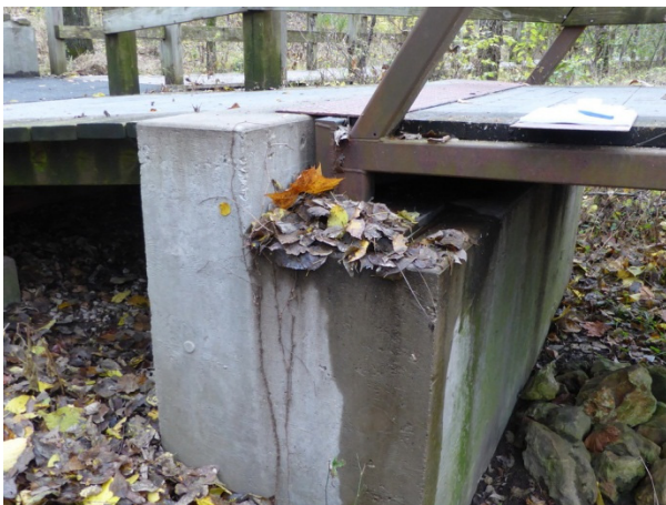
FIGURE 160. Detail of the concrete foundation stem wall on Bridge 1.
