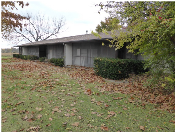
FIGURE 152. The four-unit seasonal housing building, view looking northwest towards the front facade.
