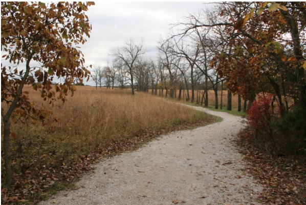
FIGURE 107. Gravel surfacing is used where the trail passes out of the woodland and follows the walnut fencerow.
