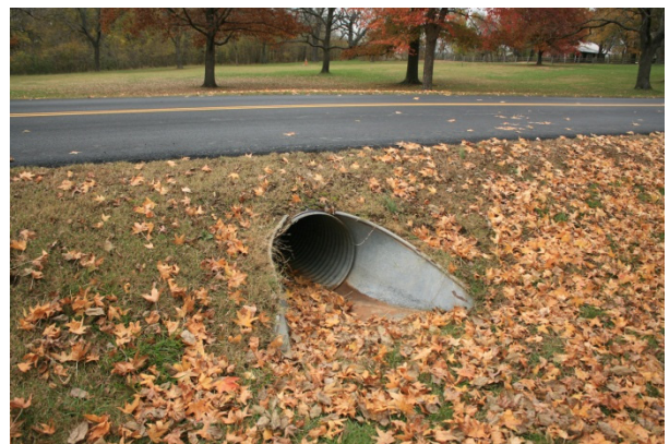
FIGURE 64. Swales and culverts convey storm water away from the entrance road.
