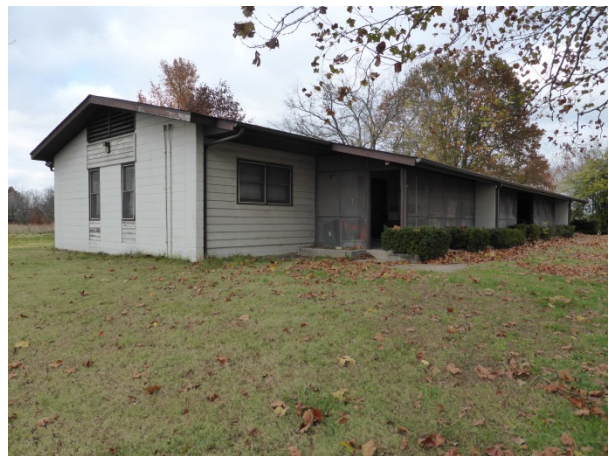
FIGURE 154. The four-unit seasonal housing building, view looking northeast.
