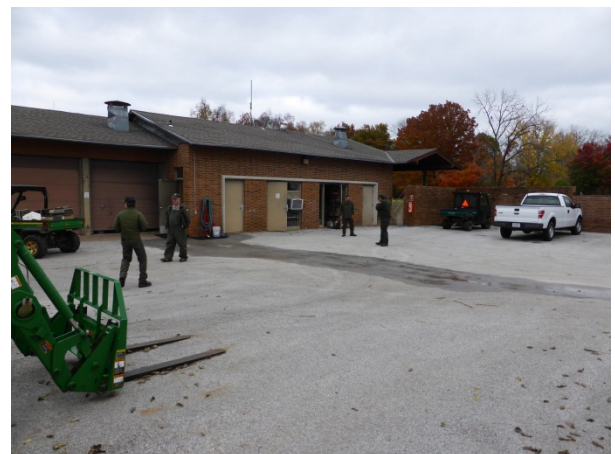
FIGURE 229. Maintenance facility and staff at George Washington Carver National Monument.
