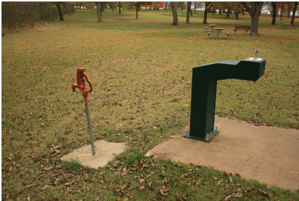
FIGURE 186. The drinking fountain and water spigot in the picnic area.
