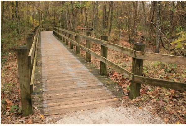
FIGURE 105. Boardwalk is used where the trail crosses the confluence of Carver and Williams branches.
