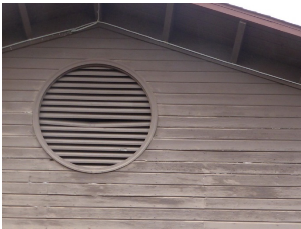
FIGURE 138. Detail of the warped and deteriorated wood siding and paint, as well as the damaged ridge vent, under the roof.
