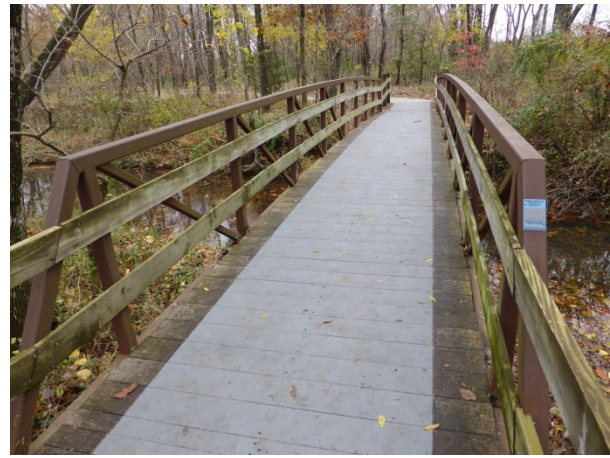
FIGURE 161. View of wood decking and the wood railings.
