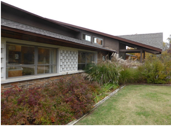
FIGURE 136. View looking northwest of the original visitor center, foreground. Note the decorative limestone panels between the steel sash windows.
