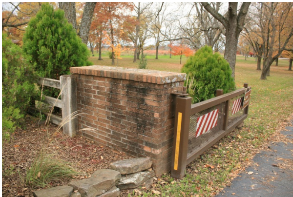
FIGURE 170. The brick piers that flank the park entrance were constructed as part of the Mission 66-era park development program.
