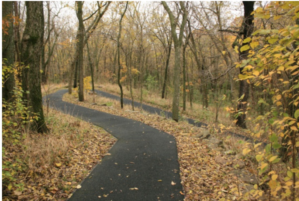
FIGURE 67. Portions of the Carver Trail feature switchbacks to meet universal accessibility standards.
