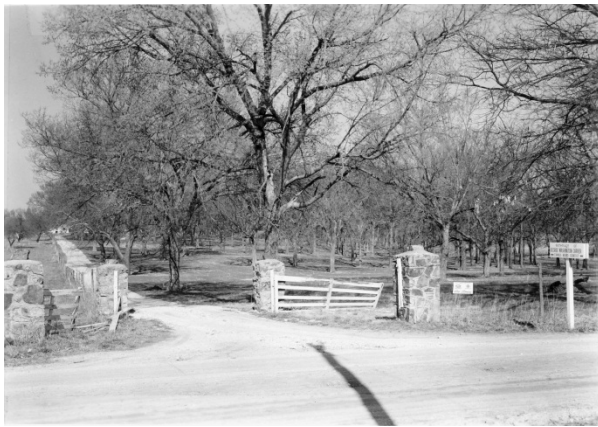
FIGURE 194. Similar stone piers marked the entrance to the property during Shartel ownership. Source: George Washington Carver National Monument photo collection.
