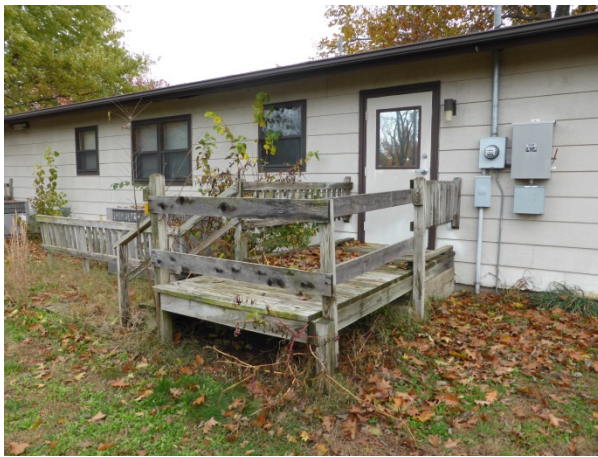
FIGURE 150. Detail of the rear wood deck.
