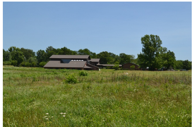
FIGURE 234. The leach field and fields west of the visitor center; the leach field should be screened from view from visitor use areas.
