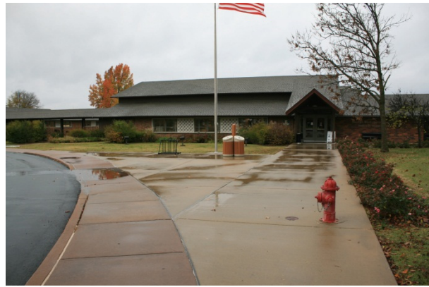
FIGURE 118. A wide concrete walk leads from the parking area to the front of the visitor center.
