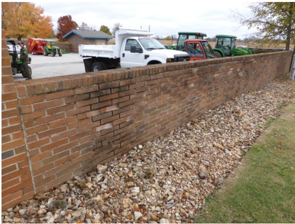
FIGURE 230. The parking area for maintenance vehicles.
