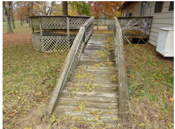
FIGURE 146. Detail of a deteriorated wood ramp and deck behind the Superintendent's residence.
