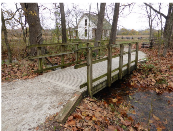
FIGURE 248. The bridge over Williams Branch leads to the Moses Carver house and demonstration gardens.
