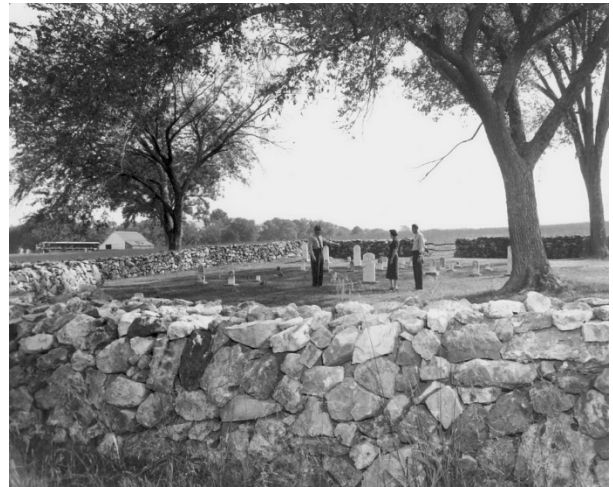
FIGURE 298. Photograph dated 1955 of work completed on the cemetery stone wall. Source: George Washington Carver National Monument Photo Collection, image 417.
