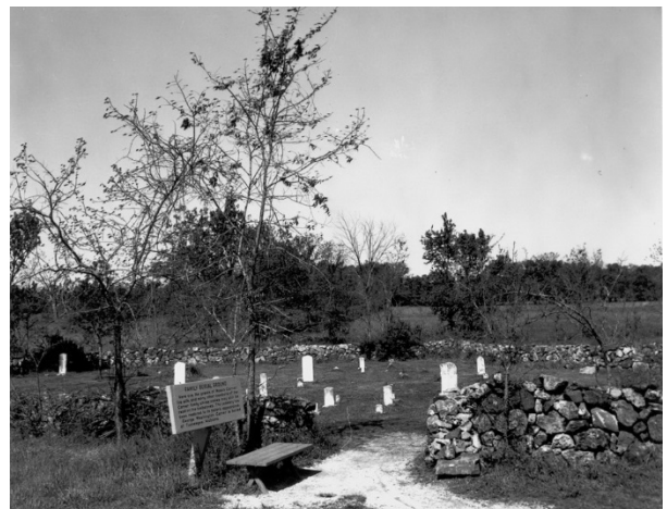
FIGURE 299. Another view of the wall soon after the 1954 restoration. Source: George Washington Carver National Monument Photo Collection, image 2120.
