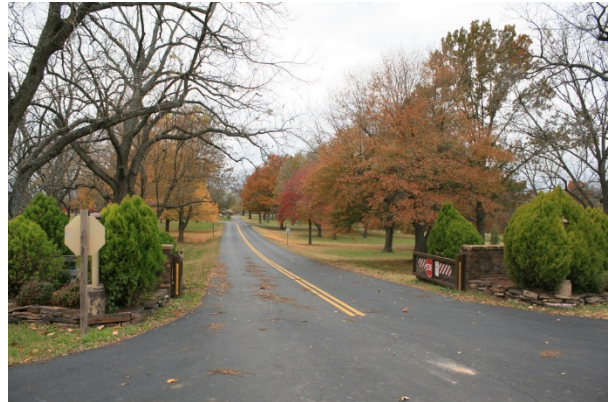
FIGURE 249. The park entrance road is a tree-lined corridor that affords views to the visitor center.
