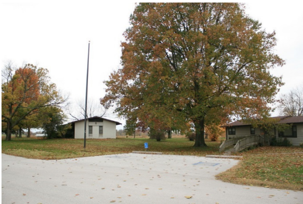
FIGURE 255. Current structures would be demolished before development of an overflow parking area.
