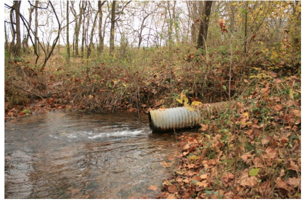
FIGURE 164. The Williams Pond dam includes a discharge pipe.
