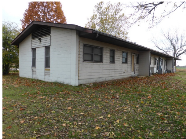
FIGURE 155. The four-unit seasonal housing building, view looking towards the east and rear facades.
