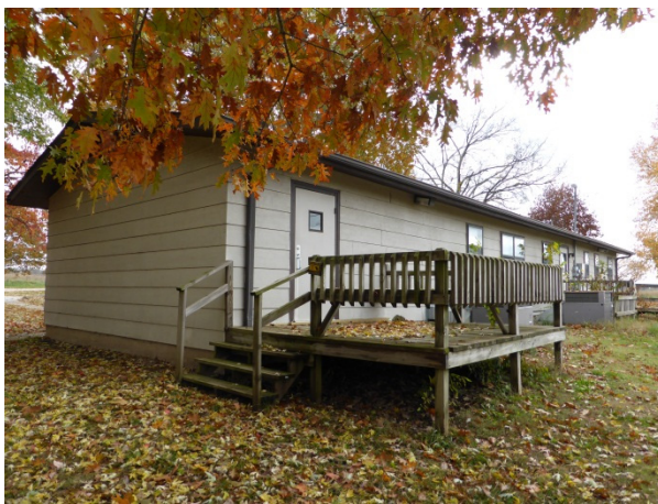
FIGURE 151. Detail of the rear wood deck.
