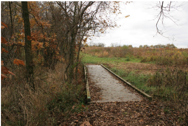
FIGURE 112. A wood-edged boardwalk conveys the trail over a wet area on the south side of the pond.
