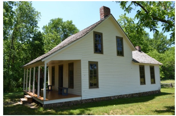
FIGURE 228. A ranger on the porch of the Moses Carver house.
