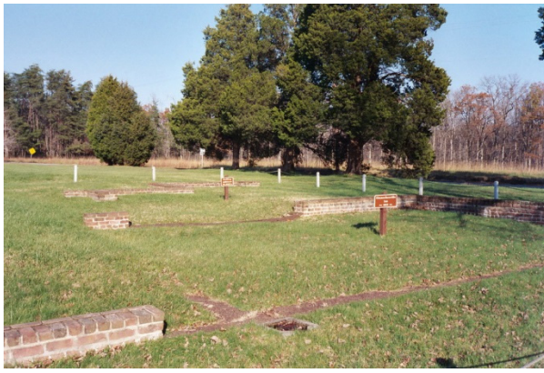
FIGURE 290. An example of the interpretation of missing features using low brick foundation structures. Source: JMA collection.
