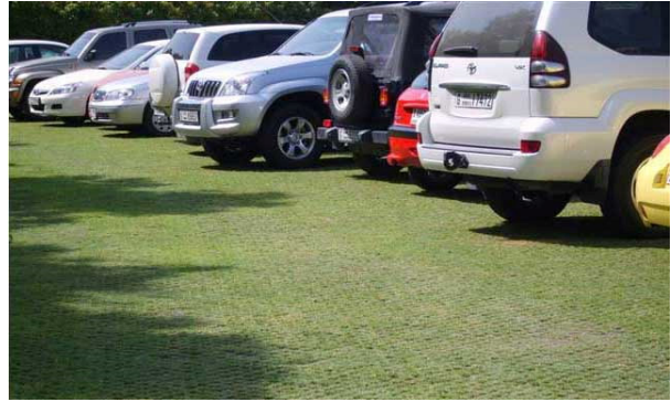
FIGURE 306. An example of a pervious grass paver system used for parking. Source: JMA collection.
