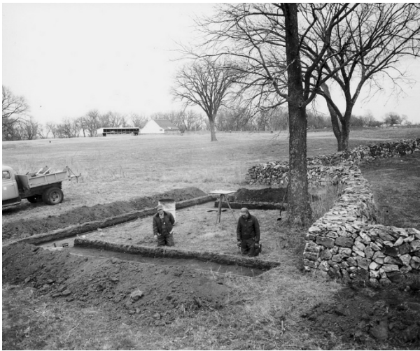
FIGURE 300. This photograph offers clues to the construction methods used in the 1954 restoration. Source: George Washington Carver National Monument Photo Collection, image 5065.
