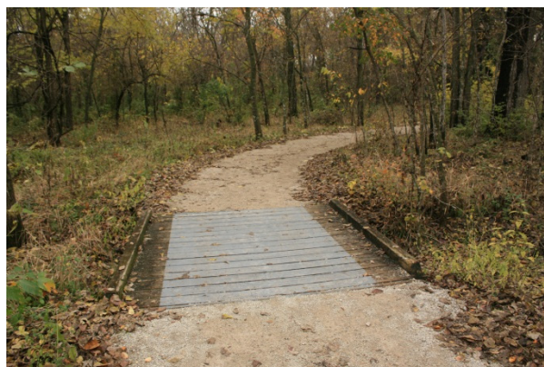
FIGURE 103. The trail is surfaced with gravel as it passes through the woodland, and is set with wooden footbridges where it passes over wet areas and ephemeral streams.
