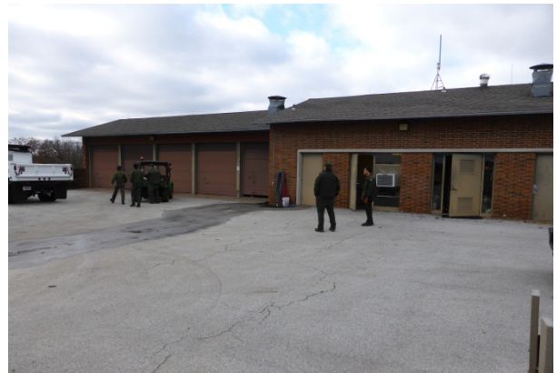
FIGURE 140. The maintenance building, view looking northwest from the maintenance yard.
