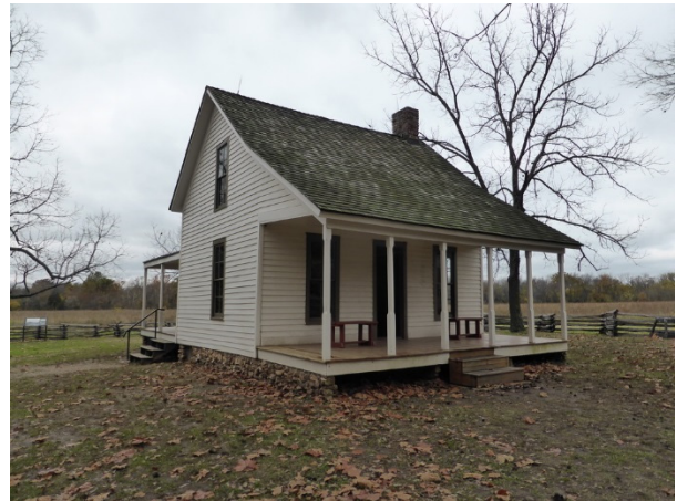
FIGURE 266. Steps in front of the Moses Carver house are not consistent with universal accessibility standards, and prevent a barrier to some to enjoy the interior of the building and associated interpretive information.
