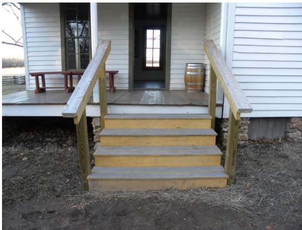
FIGURE 129. View of the rear porch stair and floor. The porch stairs were rehabilitated in 2014.
