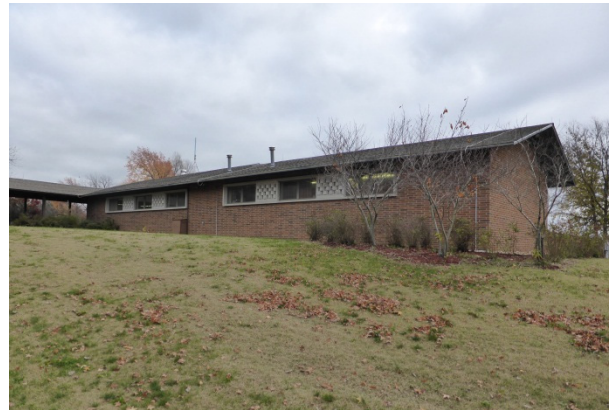
FIGURE 139. The maintenance building, view looking southeast.
