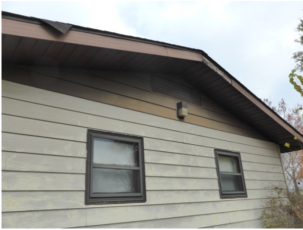
FIGURE 147. Detail of the west gable showing the deteriorated fascia and roofing.
