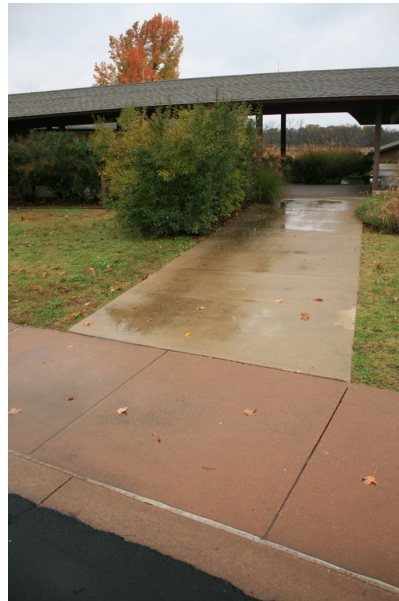
FIGURE 120. A walk connects the drop-off area and the breezeway between the visitor center and the maintenance building.
