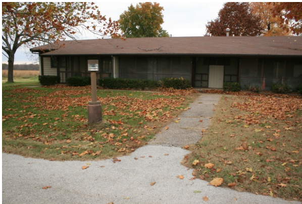
FIGURE 177. A residential-scale light in front of the four-unit seasonal housing building.
