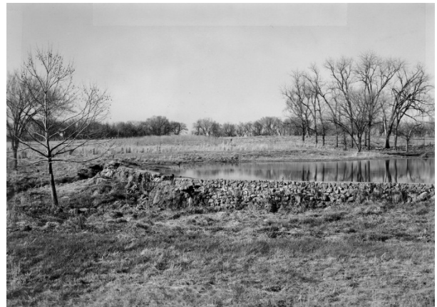
FIGURE 165. The original dam was constructed in the 1930s. As shown, the earthen structure was reinforced with a mortared rock wall. Source: George Washington Carver National Monument photo collection.
