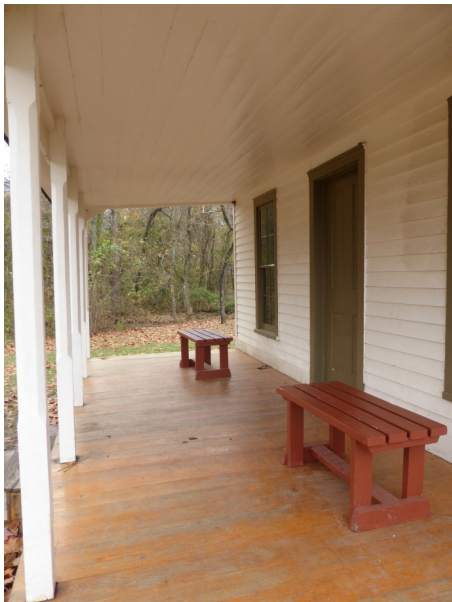
FIGURE 130. The front porch of the Moses Carver house.
