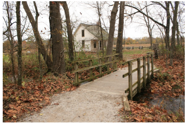
FIGURE 48. A footbridge conveys visitors over Williams Branch near the Moses Carver house.
