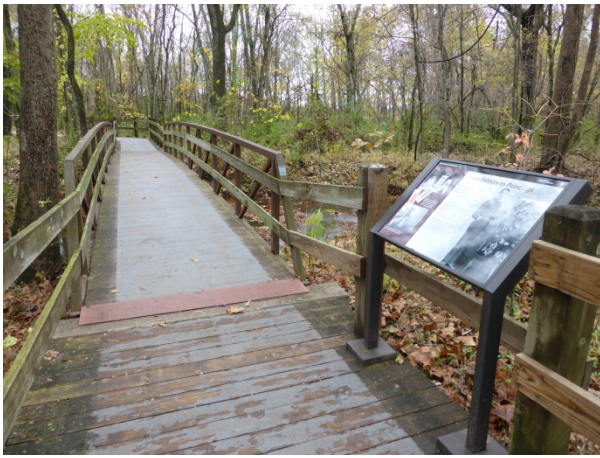
FIGURE 159. Bridge 2, view looking south from the approach ramp.
