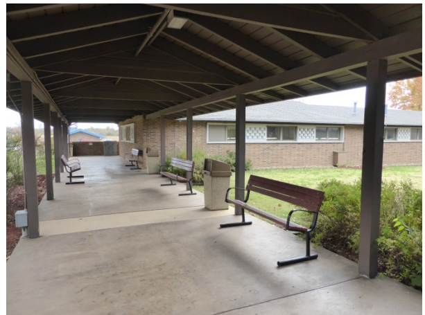
FIGURE 134. View south of the breezeway connecting the visitor center and the maintenance building.
