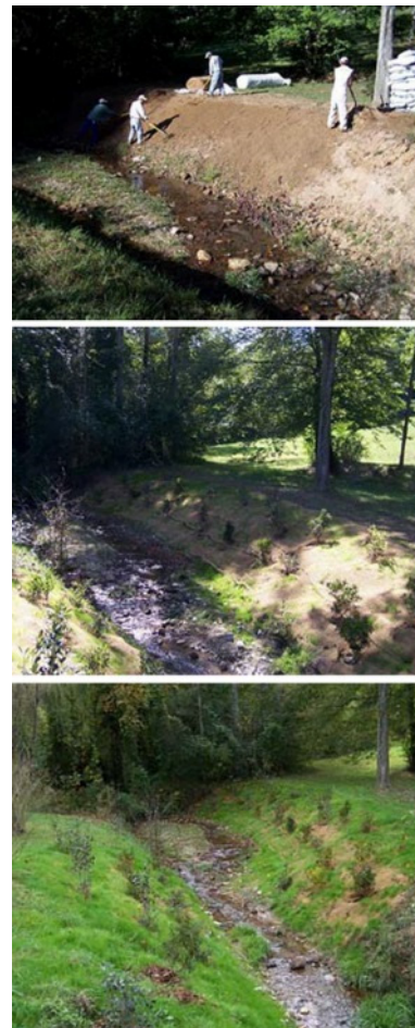
FIGURE 304. The process of streambank restoration would follow a comprehensive plan developed for the park. Source: JMA collection.
