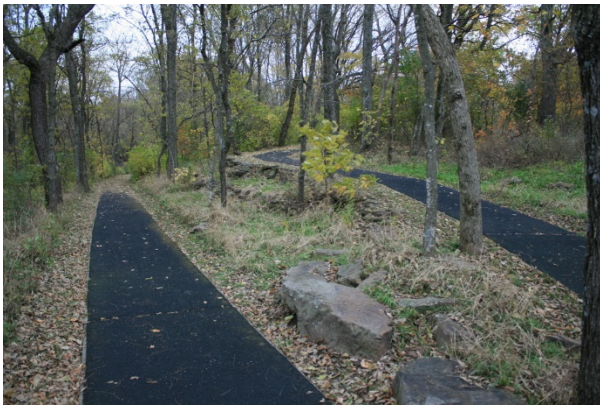
FIGURE 281. Asphalt surfacing is used on the steeper slopes of the switchbacks leading to Carver Spring.
