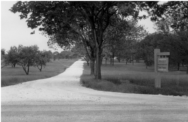
FIGURE 26. The entrance to the park, 1954. Source: George Washington Carver National Monument Photo Collection.
