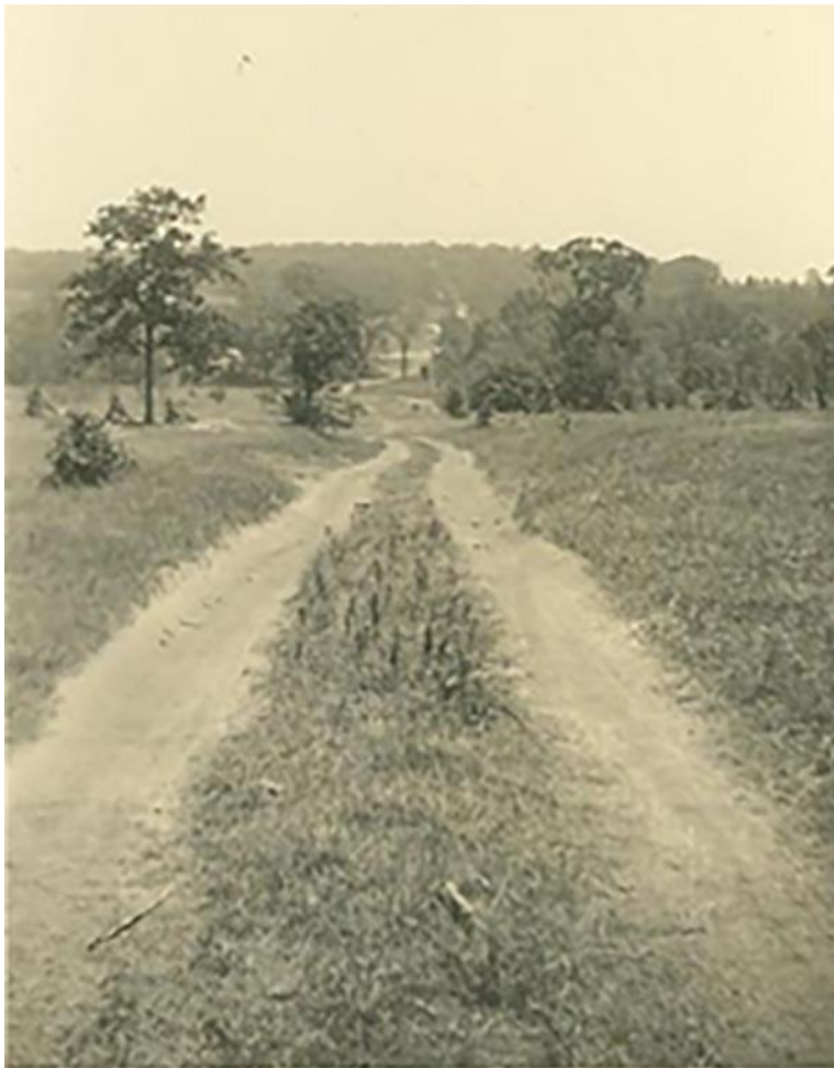
1936 Farm road from Chinn House to Chinn Branch, now South Chinn Drive, MANA Archives
