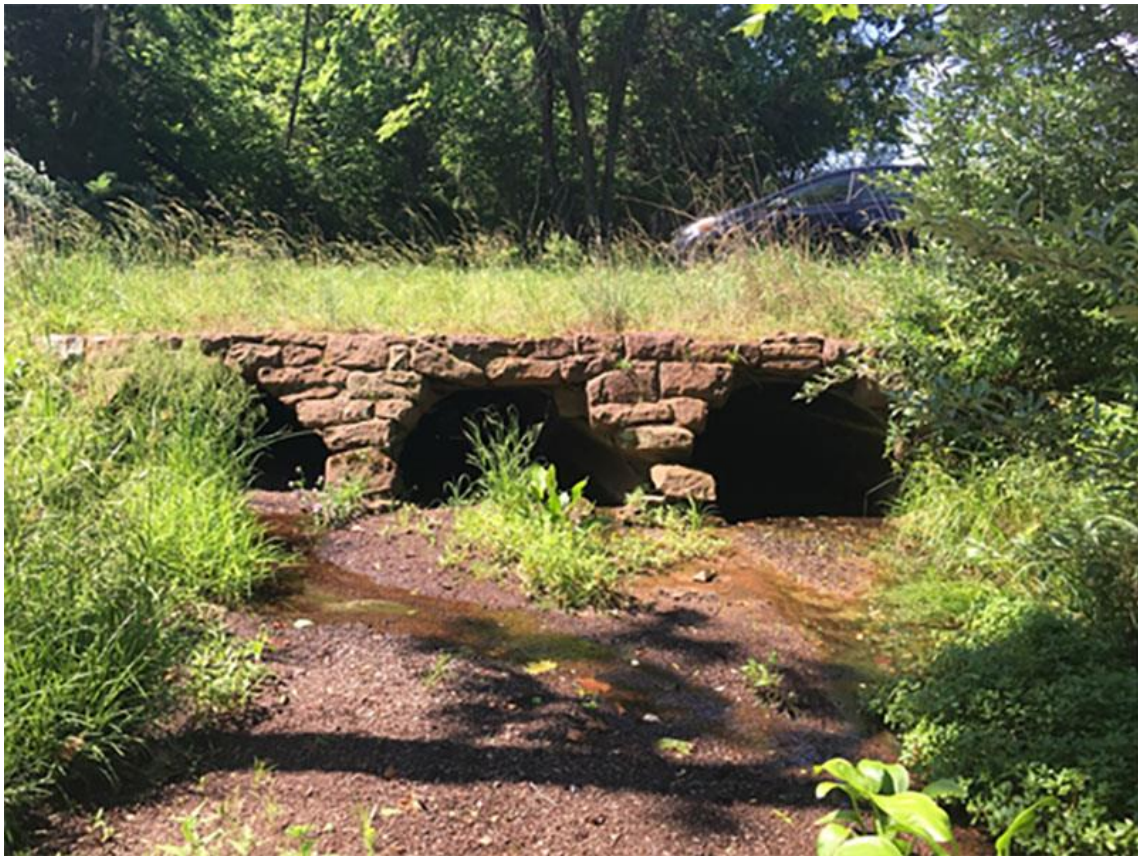
2016 north side of southern culvert over S. Chinn Drive
