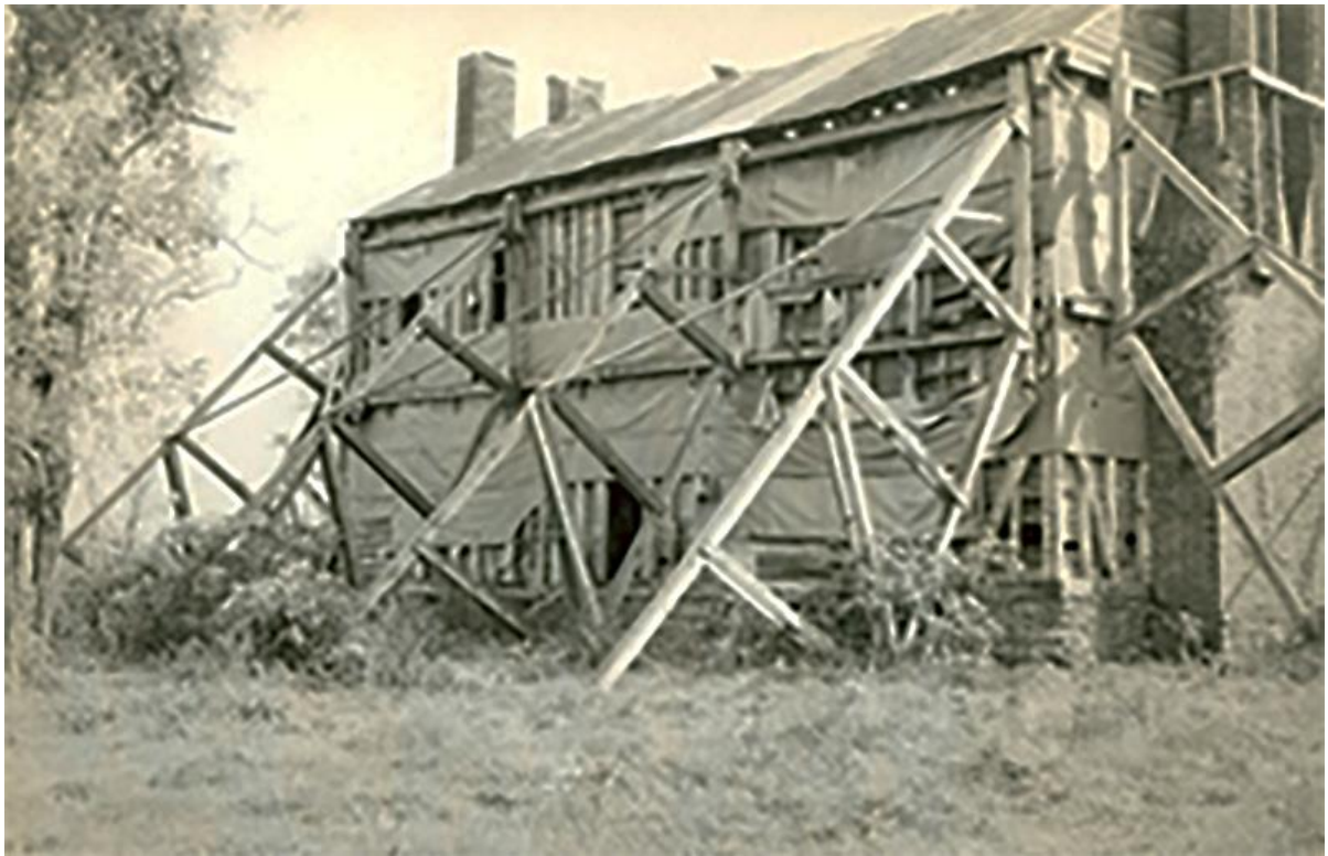
Chinn House, weatherboards removed, tar paper installed, 1940, MANA Archives
