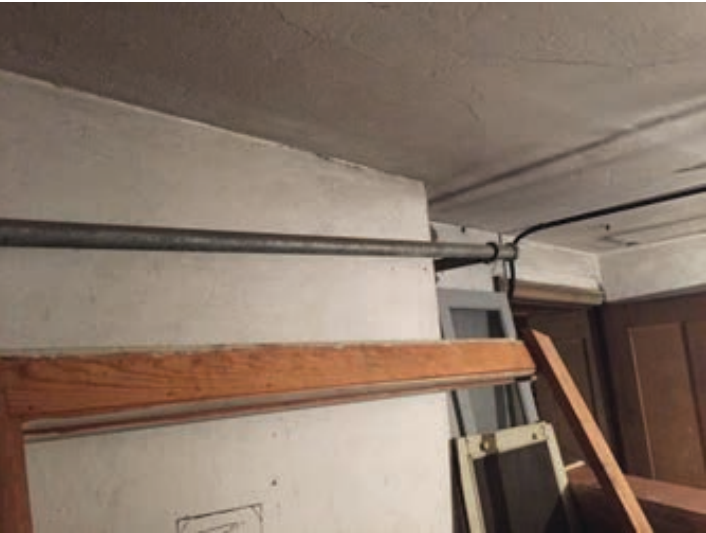
Galvanized domestic water pipes run throughout the basement
