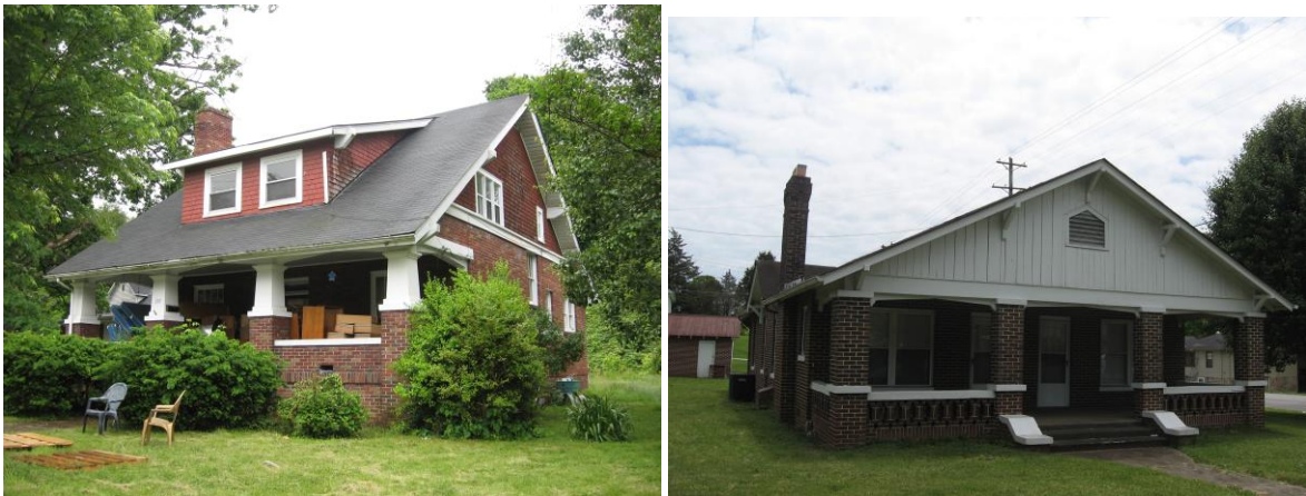
Figures 48 and 49: From left to right, CP-238 at 292 5 th Street in Jellico and CP-280, 702 E. Central Avenue in LaFollette.
