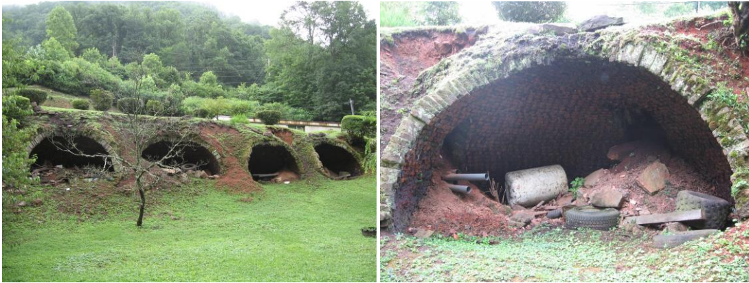
Figures 123 and 124: From left to right, east battery of the coke ovens and a detail of the coke oven interior.
