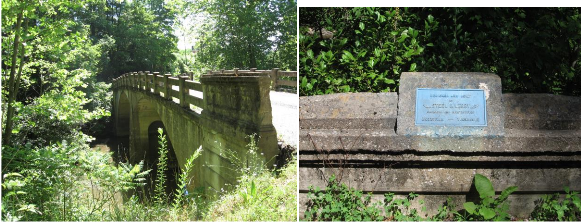
Figures 130 and 131: Steel and Lebbly Bridge (CP-304).
