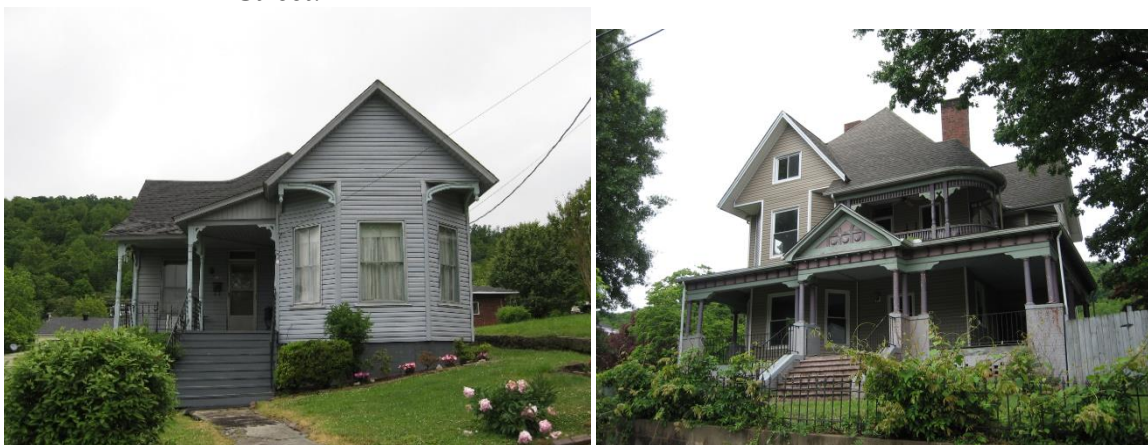
Figures 139 and 140: CP-261 at 594 Welch Street and CP-258 at 462 Welch Street.
