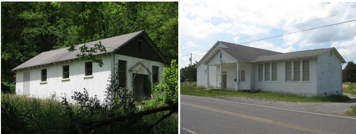
Figures 84 and 85: From left to right, CP-275 Terry Creek School in Pioneer and CP-226 Davis Chapel School in LaFollette.
