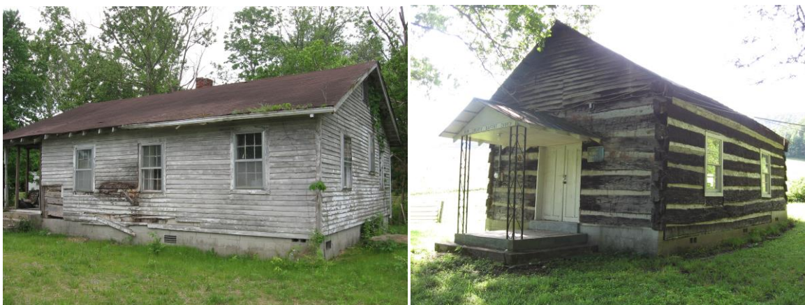
Figures 11 and 12: Left to right, CP-224 at 295 Glade Springs Road in Fincastle and CP-300 at 6369 Stinking Creek Road.
