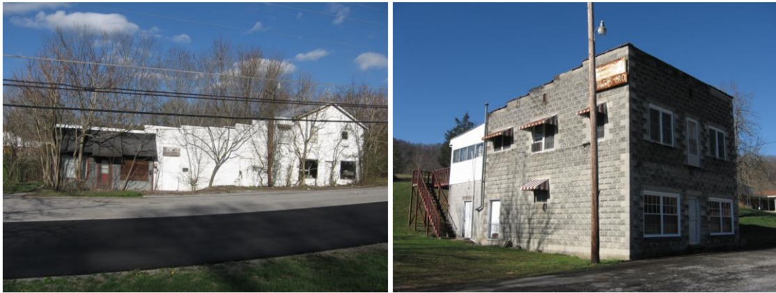
Figures 87 and 88: From left to right, CP-168 at 440 Demory Road and CP-161 at 2154 Highway 116.
