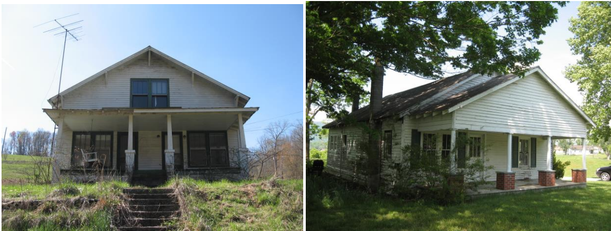
Figures 52 and 53: From left to right, CP-173 at 300 Sugar Hollow Road and CP-225 at 1195 Davis Chapel Road.
