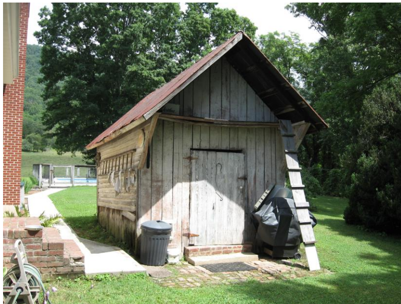
Figure 66: CP-328 at 13330 Back Valley Drive.
