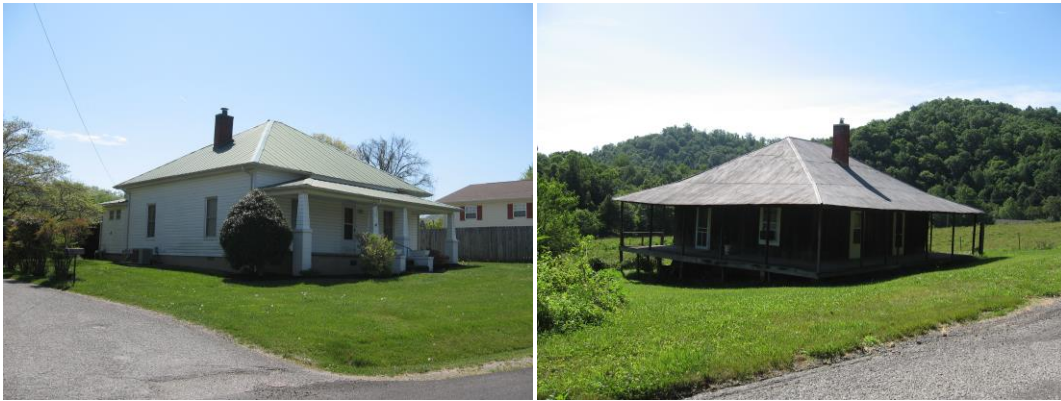
Figures 18 and 19: From left to right, CP-195 137 at Hill Street in Caryville and CP-302 4 Old Stinking Creek Road.
