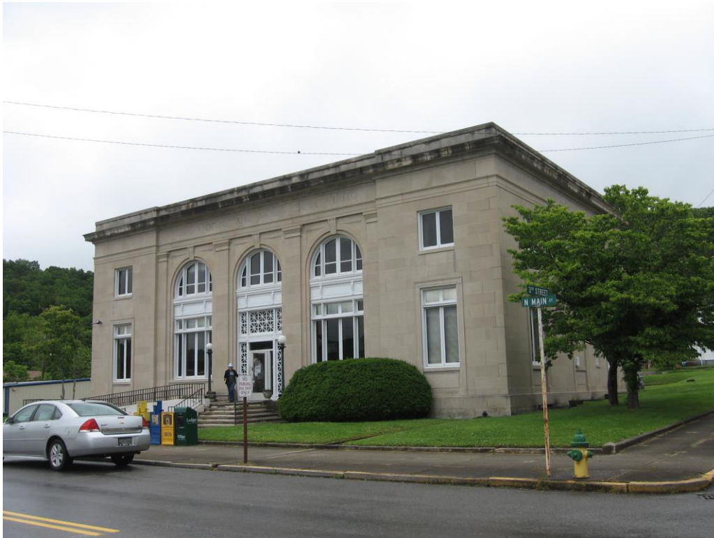
Figure 113: U.S. Post Office and Mine Rescue Station, view northeast.
