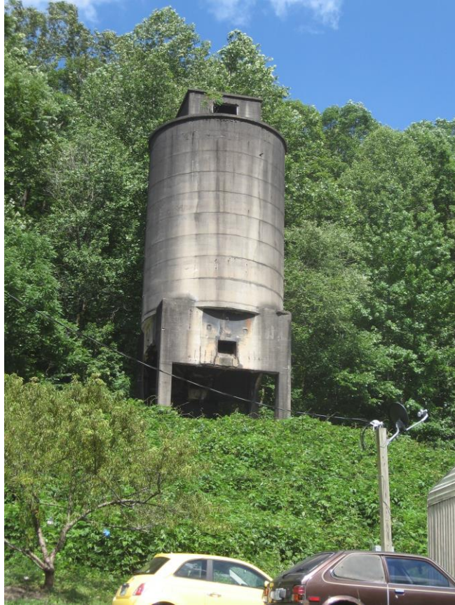
Figure 103: CP-317 Chaska Coal Loading Tower.
