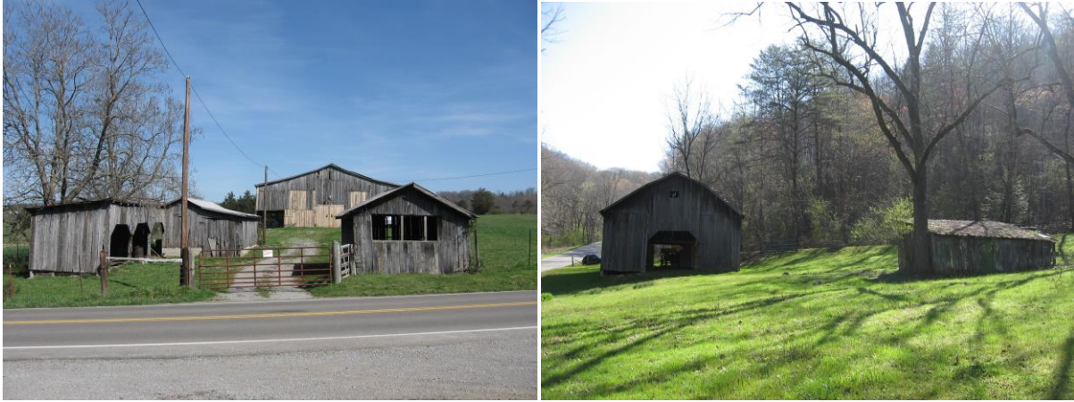
Figures 64 and 65: From left to right, CP-165 at 188 Pinecrest Road and CP-172 1595 Demory Road.
