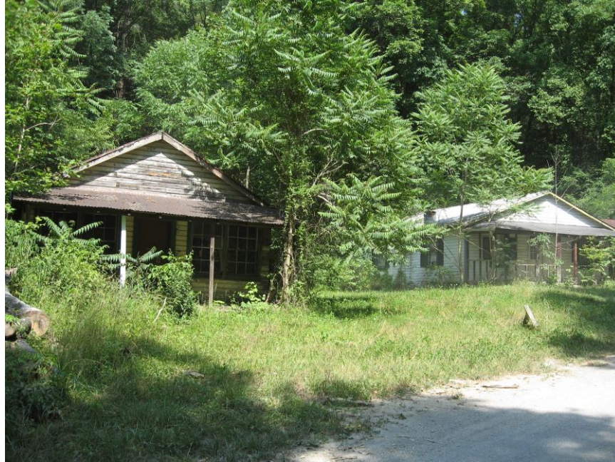
Figure 104: CP-305 Gennett Camp Structures.
