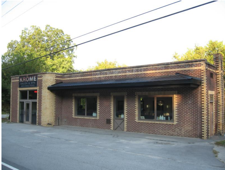
Figure 93: CP-138, 1508 Jacksboro Highway.
