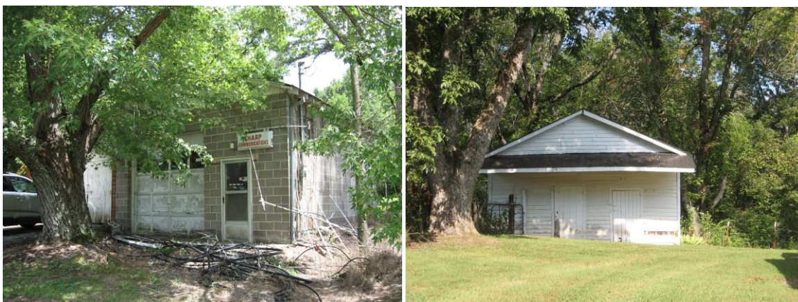
Figures 71 and 72: From left to right, CP-360 at 1605 Sharps Ridge Lane and CP-394 at 4192 General Carl Stiner Highway.
