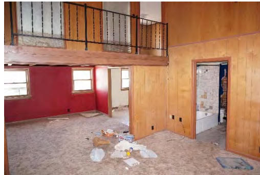
PHOTO 53: TYPICAL SECOND FLOOR APARTMENT FINISHES
