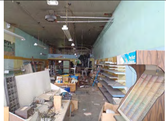
PHOTO 36: DEBRIS IN BUILDING BEFORE CLEANOUT
