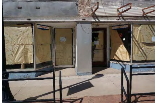
PHOTO 26: DETAIL OF STOREFRONT
