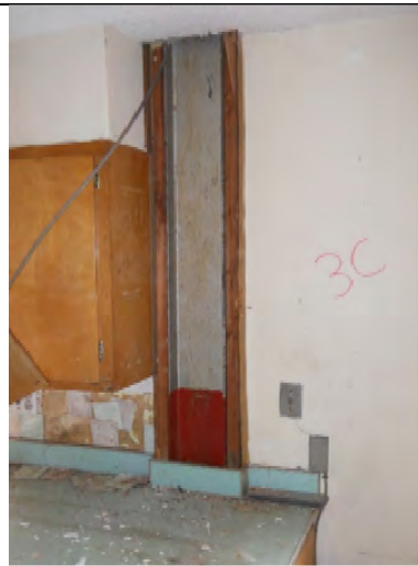
PHOTO 41: GREY AND RED STEEL COL AT NORTH WALL OF SECOND FLOOR
