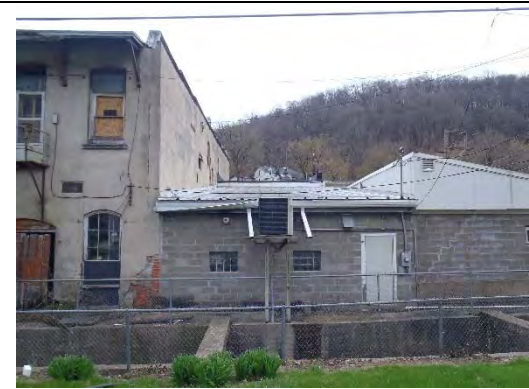
PHOTO 12: NORTH FAÇADE- NEIGHBORING BUILDINGS
