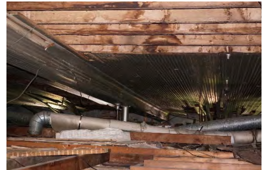
PHOTO 60: SPACE ABOVE APT CEILINGS IN FORMER BALLROOM
