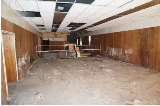
PHOTO 43: FIRST FLOOR AFTER DEBRIS REMOVAL
