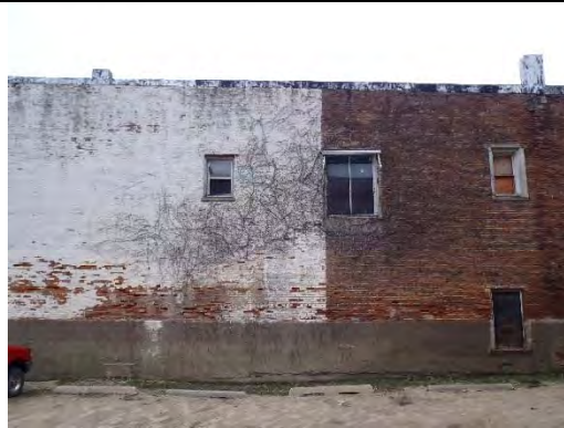
PHOTO 5: PARTIAL EAST FACADE
