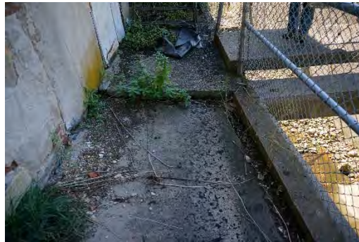
PHOTO 29: WALKWAY BETWEEN BUILDING AND STORM SEWER IN NORTH YARD
