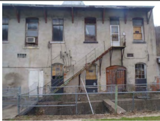
PHOTO 11: PARTIAL NORTH FAÇADE
