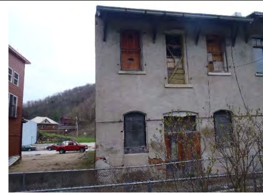
PHOTO 9: PARTIAL NORTH FAÇADE
