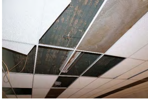
PHOTO 44: WOOD CEILING OF FIRST FLOOR SPACES
