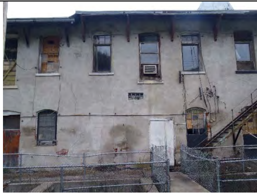
PHOTO 10: PARTIAL NORTH FAÇADE
