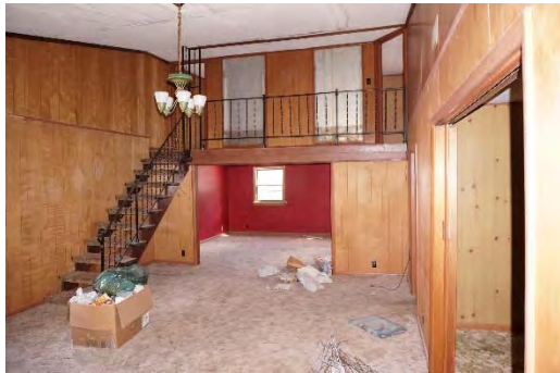
PHOTO 52: TYPICAL SECOND FLOOR APARTMENT FINISHES
