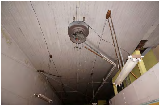
PHOTO 46: WOOD CEILING OF FIRST FLOOR SPACES
