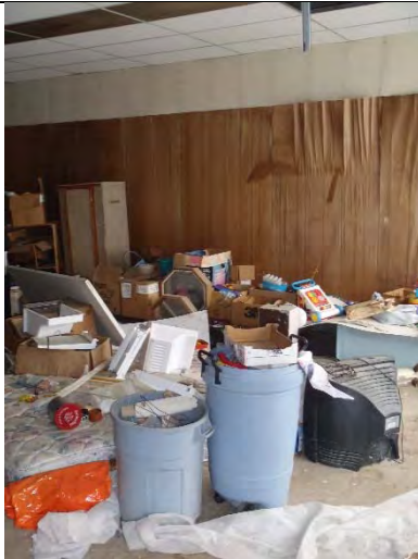
PHOTO 31: DEBRIS IN BUILDING BEFORE CLEANOUT
