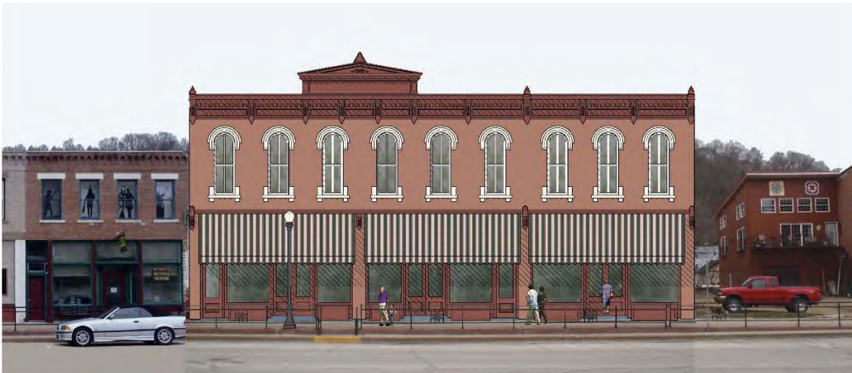
Showing rehabilitated façade with awning deployed.
