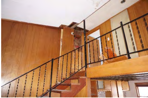
PHOTO 55: TYPICAL SECOND FLOOR APARTMENT FINISHES
