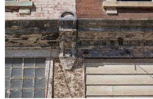
PHOTO 27: DETAIL OF STOREFRONT CORNICE
