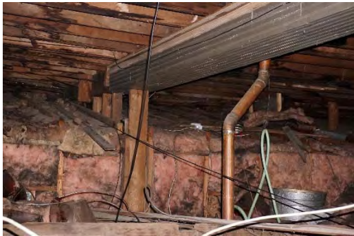
PHOTO 58: SPACE ABOVE APT CEILINGS IN FORMER BALLROOM
