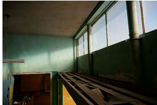
PHOTO 47: INTERIOR OF EXISTING STOREFRONT
