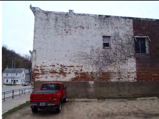
PHOTO 4: PARTIAL EAST FACADE.
