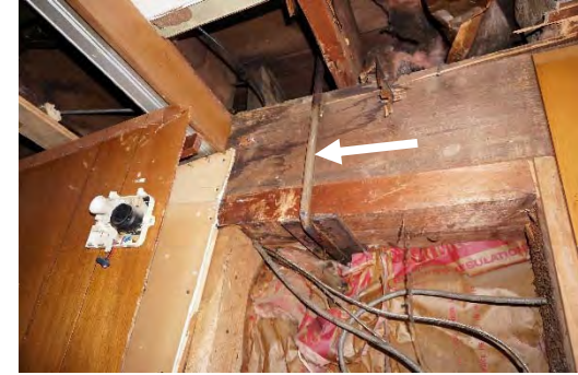
PHOTO 57: STRUCTURAL HANGER AT BUILDING CENTER BEAM
