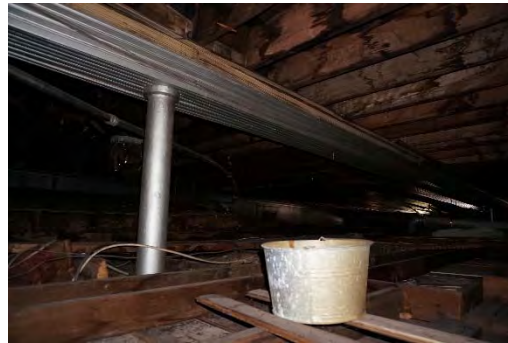
PHOTO 59: SPACE ABOVE APT CEILINGS IN FORMER BALLROOM
