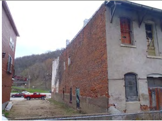
PHOTO 7: LOT EAST OF BUILDING
