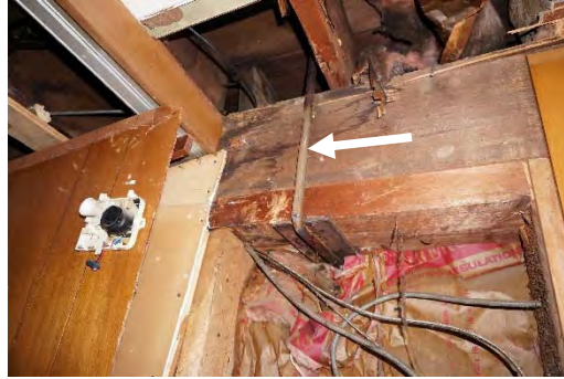
PHOTO 56: STRUCTURAL HANGER AT BUILDING CENTER BEAM
