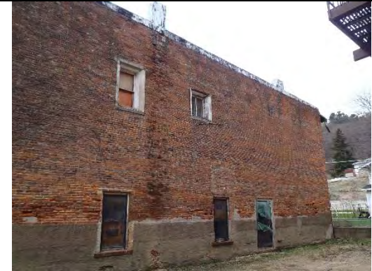
PHOTO 6: PARTIAL EAST FACADE
