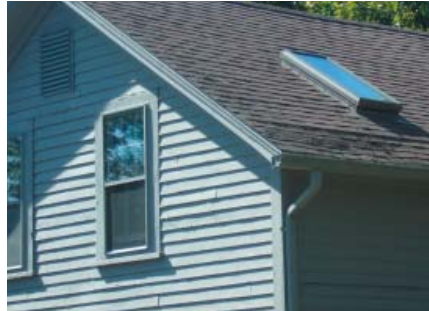
A standard aluminum ogee gutter and downspout blend with the building by matching the paint color.
