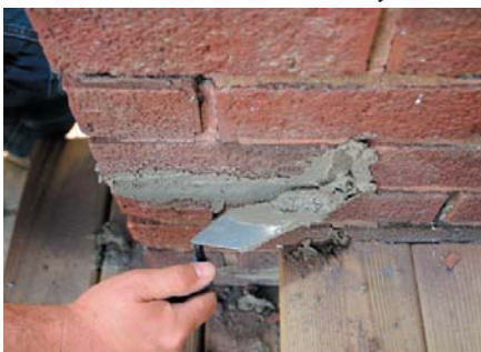
Sloppy re-pointing may leave excessive mortar on the face of the brick.
