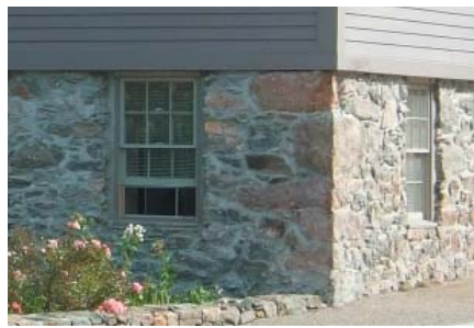
A stacked fieldstone foundation wall provides a structural and visual base for a building.
