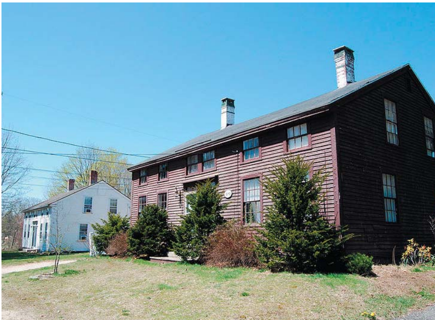
Two-story duplexes create a fabric of broad-front housing originally erected for the mill workers. The simple rectangular plan is economical, yet elegant.
