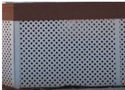
Avoid obscuring structural elements with lattice. The lattice should infill only the spaces between piers.
