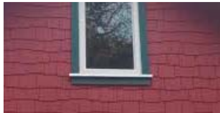
Jagged edges caused by alternating shingle exposures. Traditional shingle siding is aligned in horizontal courses.
