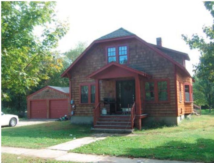
An addition to this home in Columbia Heights contributes to the composition without overwhelming the original structure.
