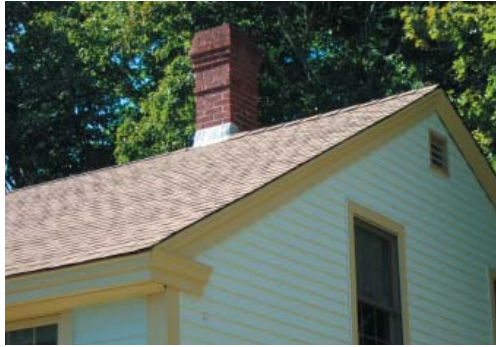
A chimney in Shannock is typically made of brick and rises from the center of the building.
