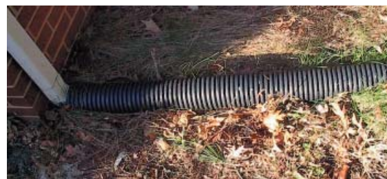
Extension hoses are unsightly additions and call attention to the poorly designed gutter system.
