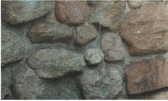
Masonry walls express strength and permanence.
