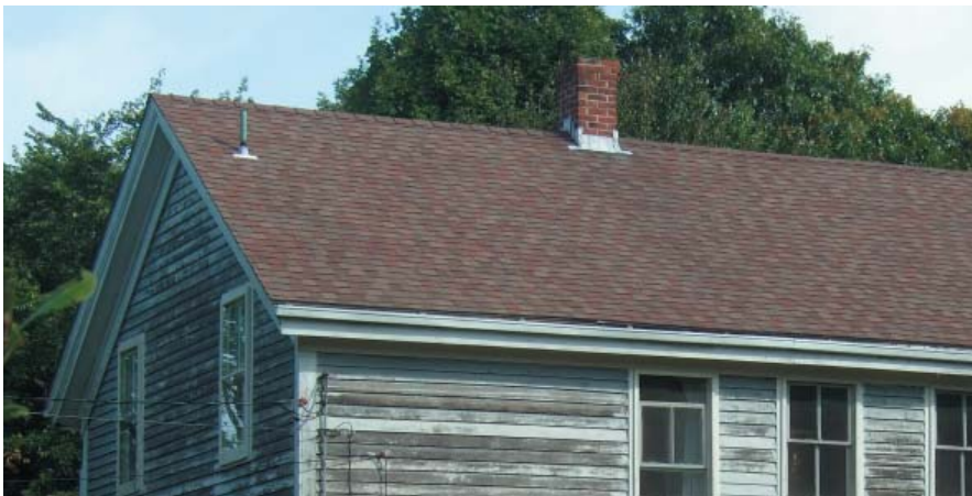
Shannock Village features a range of roofing materials, including both 3-tab and architectural asphalt shingles in a range of colors.
