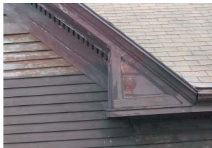
This historic eave return was later enclosed with flat trim to keep out pigeons.
