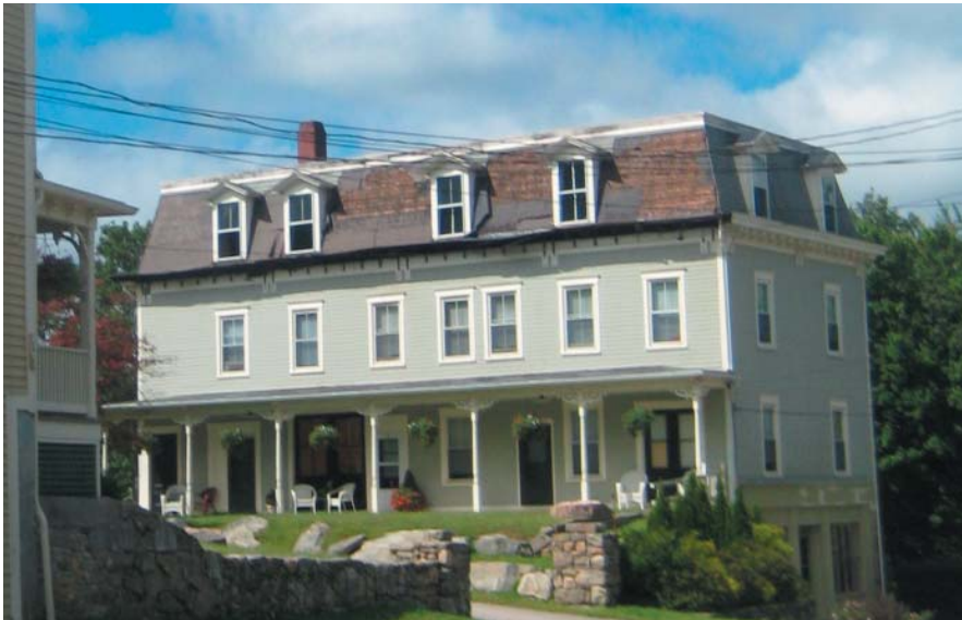
A Victorian mixed-use building with a Mansard roof and dormer windows.
