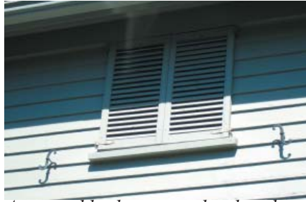
An operable shutter can be closed when the room is not in use.
