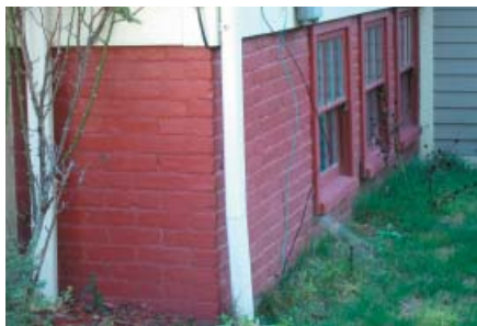
Traditional brick foundations are both structural and decorative.
