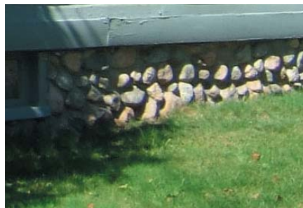
Stone foundations range from solid slabs to river rock.
