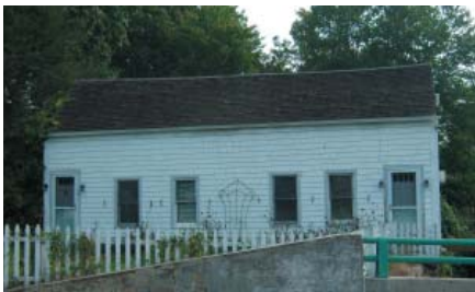
Split cedar shakes are appropriate roofing materials.
