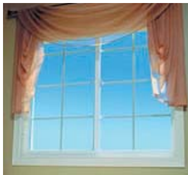
Tight-mulled windows have only a narrow vertical bar between units. This mull should be wide enough to separate two distinct window units.
