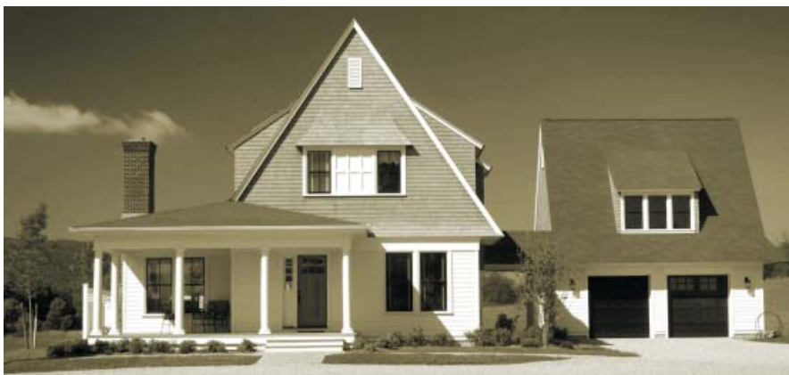
The garage is subordinate to the main house by having a lower roof spring line than that of the main house. However, the two structures share similar materials and proportions, creating an aesthetic harmony among all parts.
