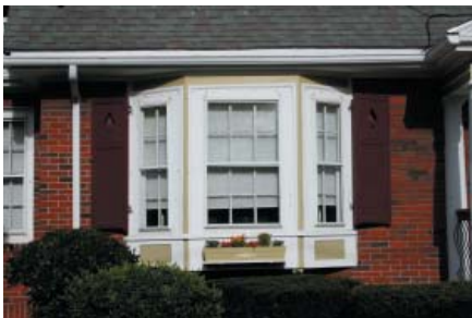
Inappropriately sized or poorly located shutters would not cover the window if they could be closed.
