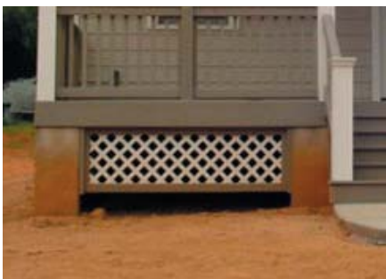
Avoid large gaps or completely open spaces under the porch, which collect unwanted refuse and animals.
