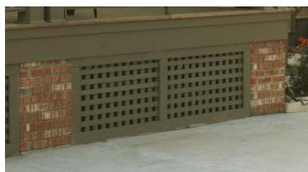
Infill panels between porch foundation piers are often wood lattice.
