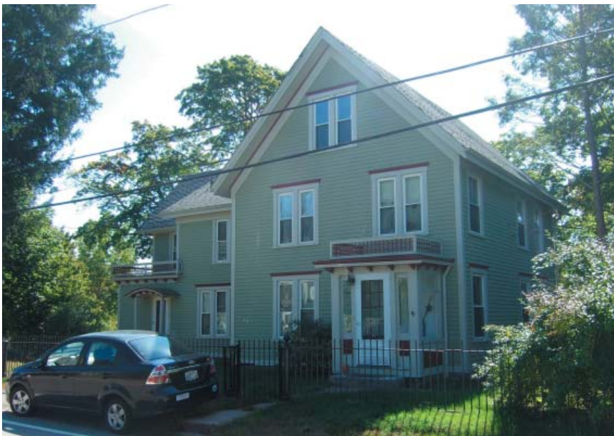
Neighborhood buildings are set back from the road. Low stone walls, fences or hedge rows are common to define the private front yard.
