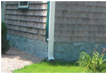
A thin coat of mortar over poured concrete foundations can create a more traditional look.
