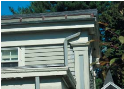
Built-in gutters use the inside of the eaves to channel water flow.
