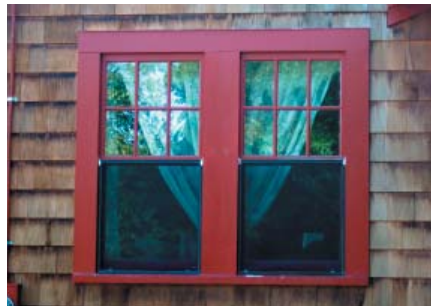
Ganged windows appear as two units with structure and trim between.
