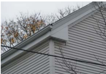
The ubiquitous "pork-chop" eave return applies a triangular box at the intersection of the eave and rake.
