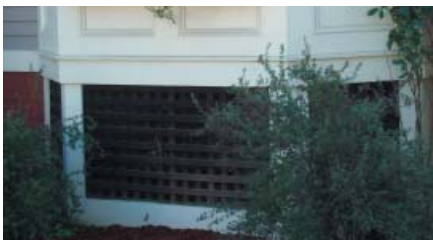
Lattice under a bay window protects the sheltered area.
